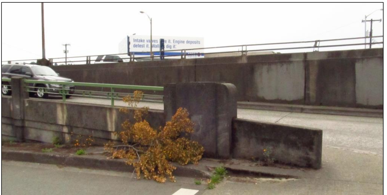
Photo 1-10: NE Quadrant - off-ramp from northbound Ballard Bridge to NW Ballard Way, looking west
