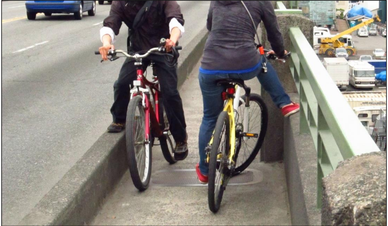
Photo 1-2: Existing conditions - opposing bicyclists along the northbound east side of Ballard Bridge
