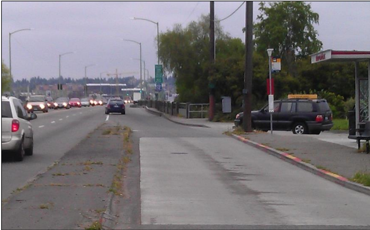
Photo 1-13: SE Quadrant - right turning movements from on-ramp north of bus stop, looking north
