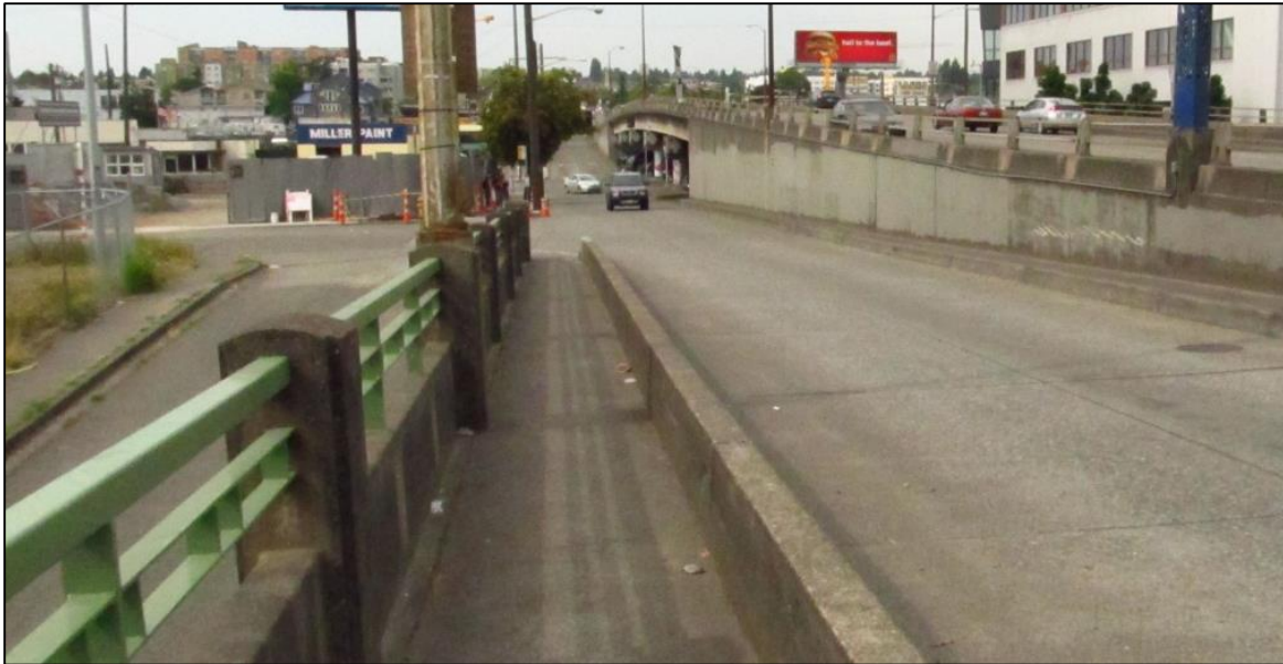
Photo 1-7: NW Quadrant - on-ramp to southbound Ballard Bridge from NW Ballard Way, looking north
