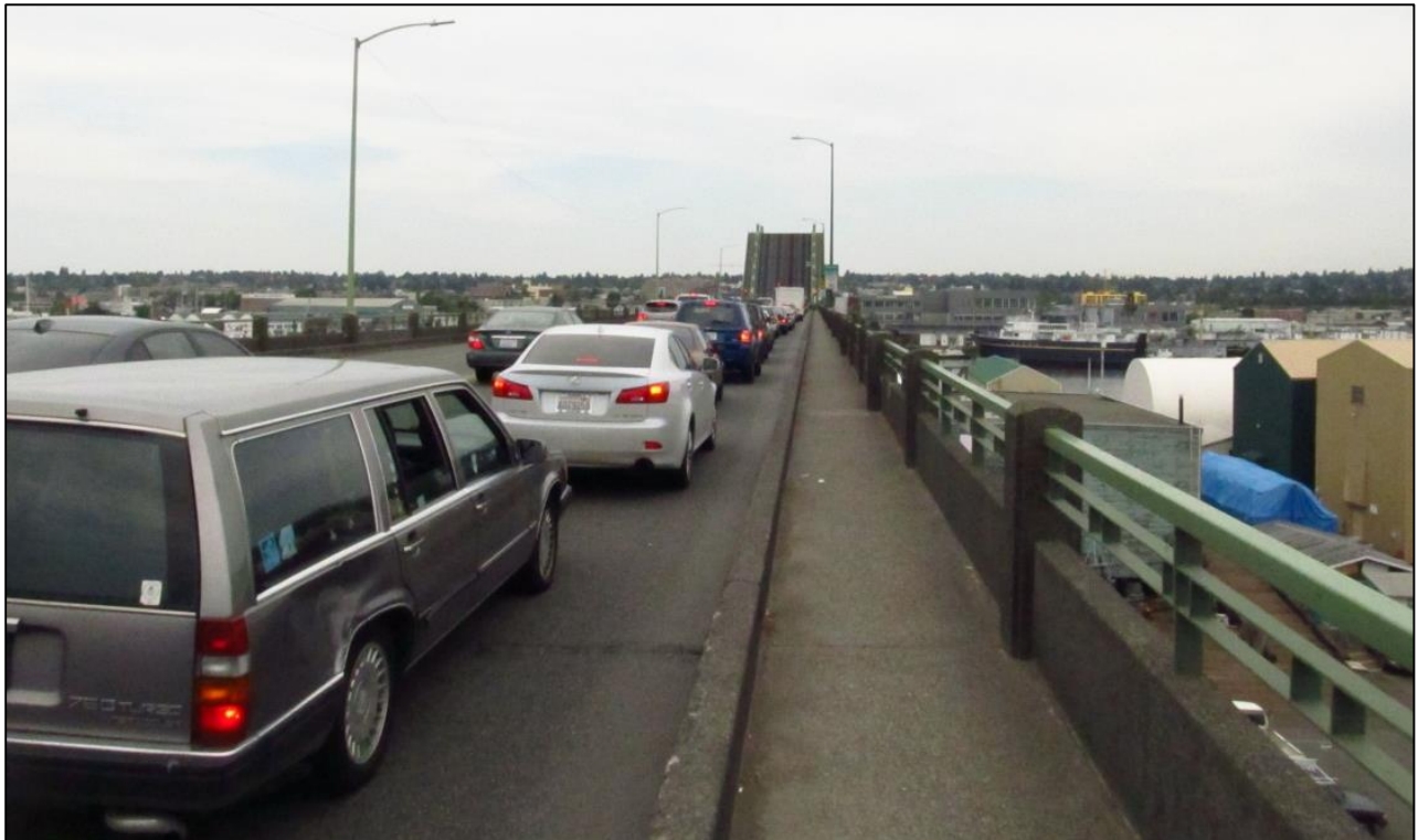
Photo 1-3: Existing conditions - narrow sidewalks on Ballard Bridge
