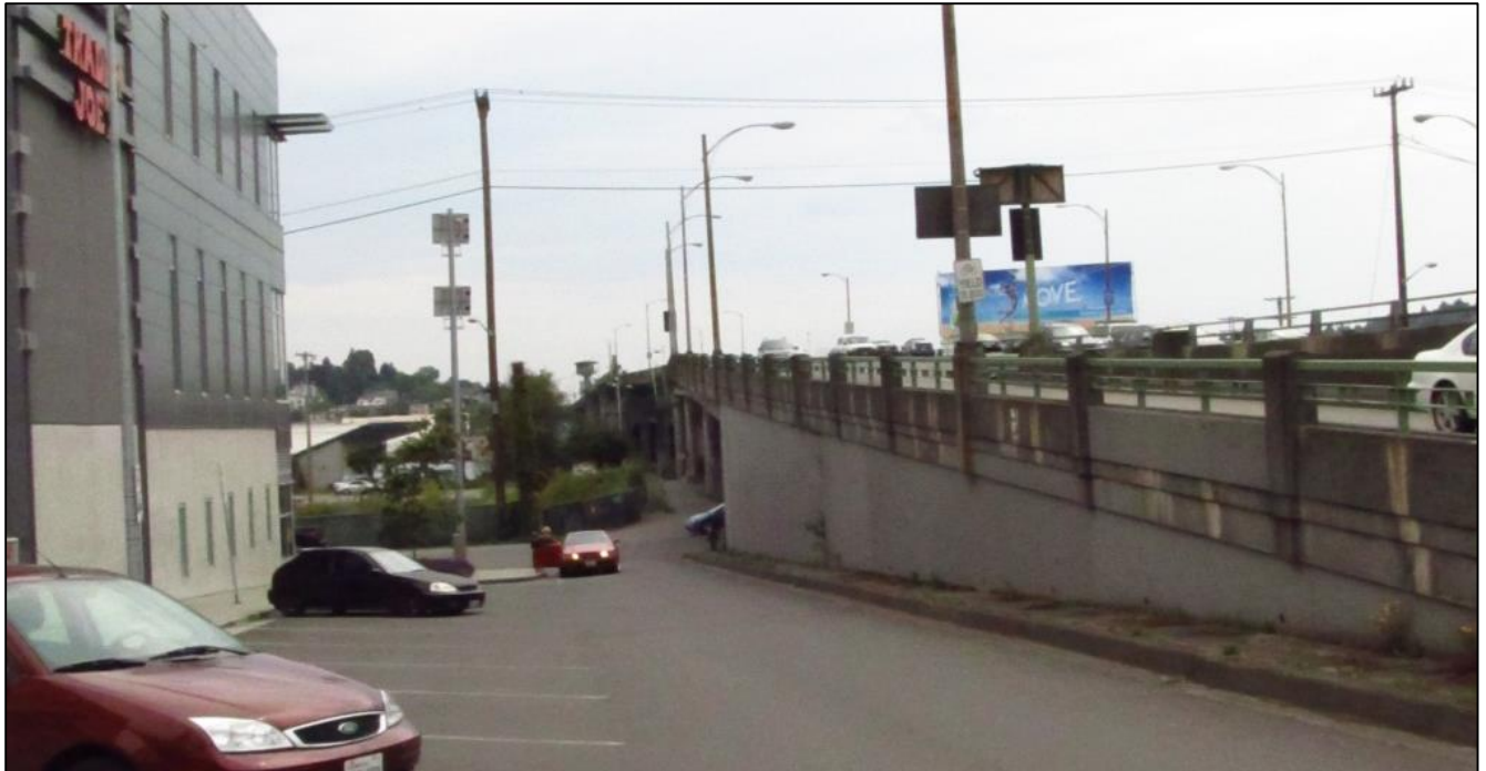
Photo 1-9: NE Quadrant - off-ramp from northbound Ballard Bridge to NW Ballard Way, looking south
