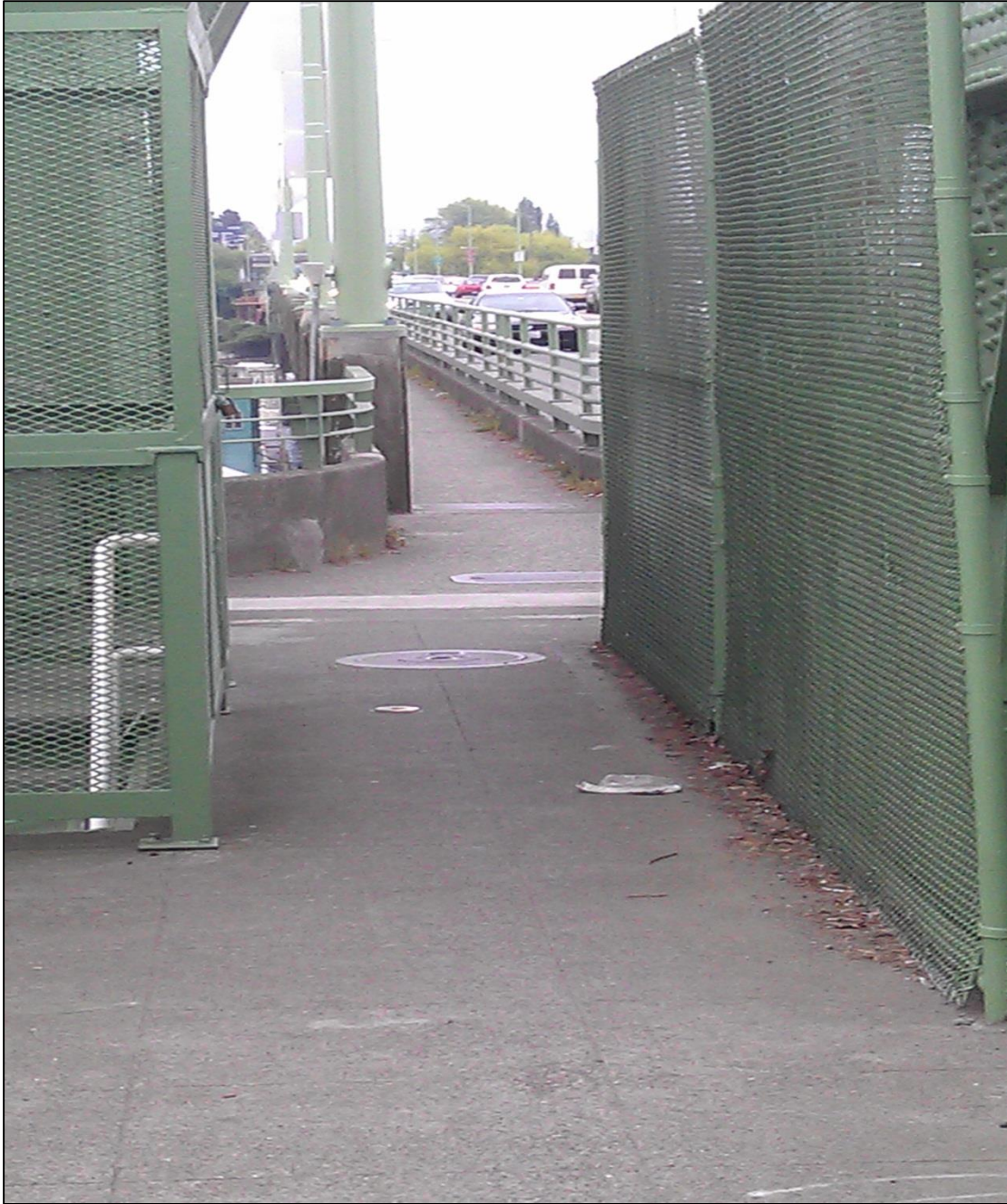
Photo 1-1: Existing conditions - narrowing sidewalks at corners of Ballard Bridge bascule
