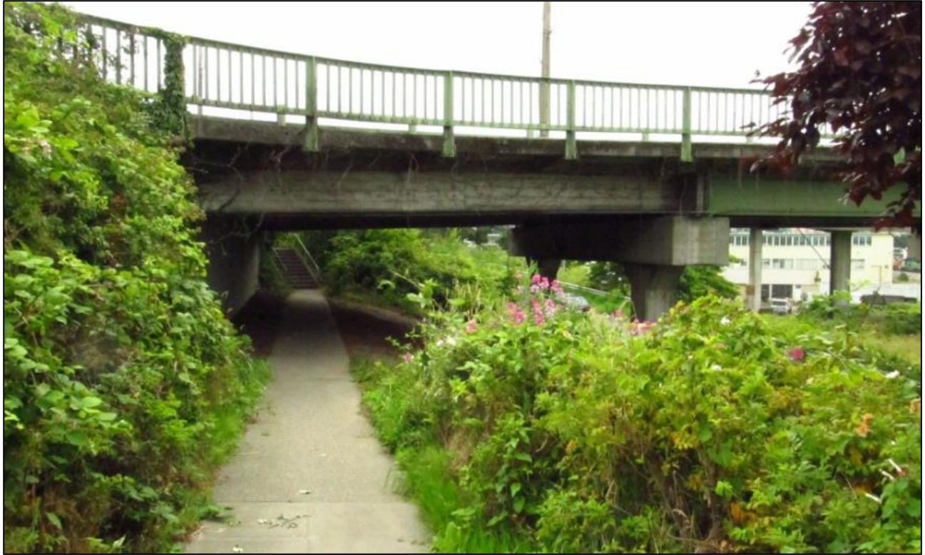
Photo 2-1: Pedestrian path crossing under Emerson Street, looking south
