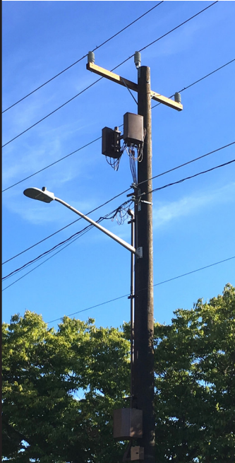
Image 1: Typical wood pole design with panel antennas
