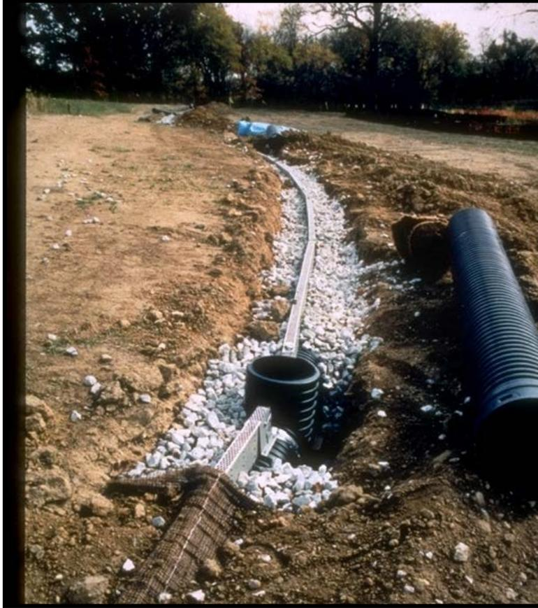
Figure E.6. Level Spreader Prior to Backfill and Downstream Stabilization.
