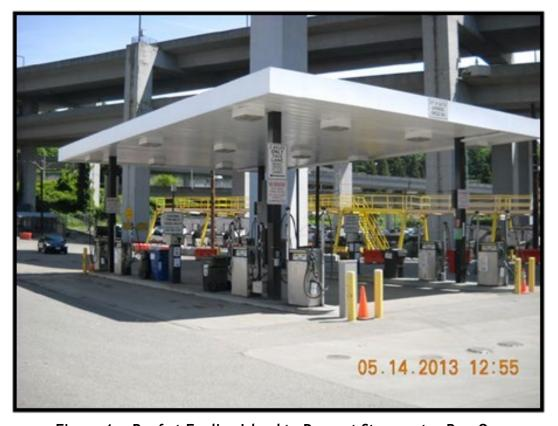
Figure 4. Roof at Fueling Island to Prevent Stormwater Run-On.
