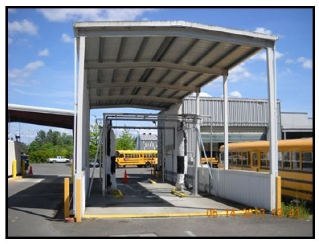
Figure 6. Car Wash Building with Drain to the Sanitary Sewer.
