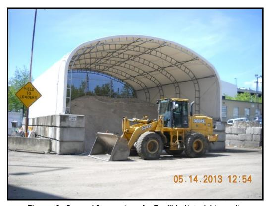
Figure 12. Covered Storage Area for Erodible Material (gravel).
