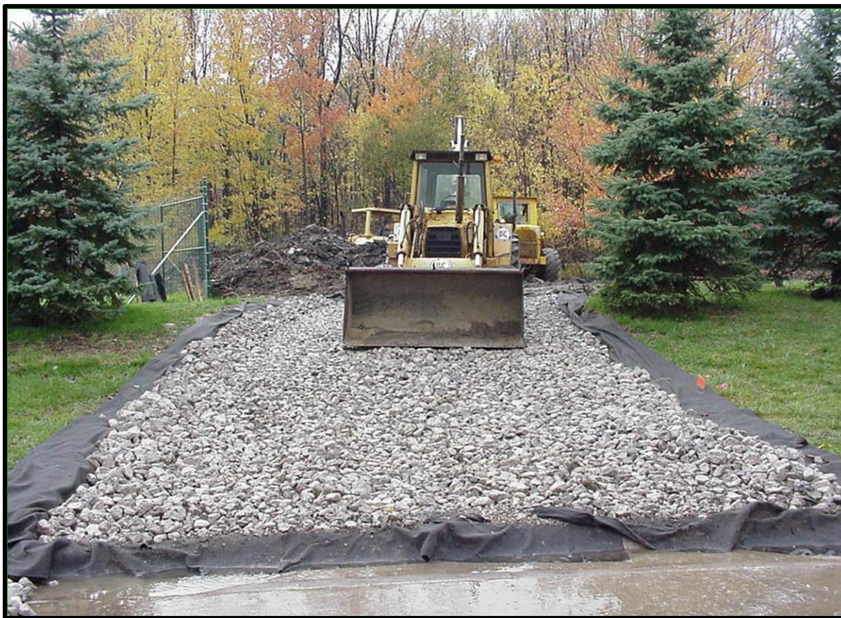
Figure 6. Stabilized Construction Access.
