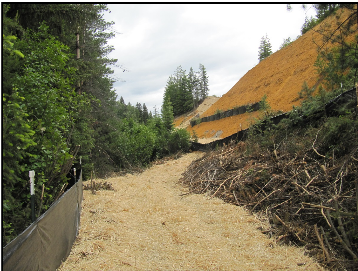
Figure 13. Filter Fence Installed on a Slope.
