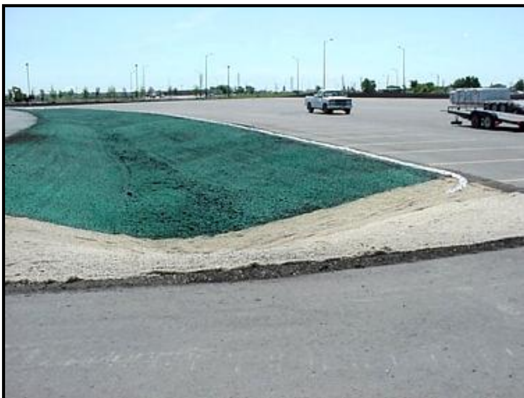
Figure 1. Hydroseeding Method.
