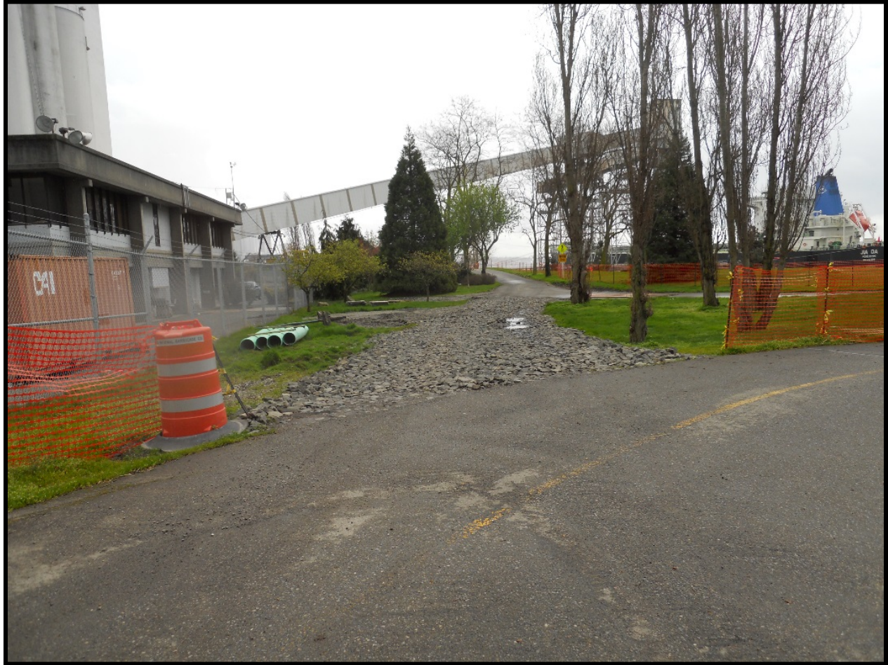
Figure 7. Stabilized Construction Access.
