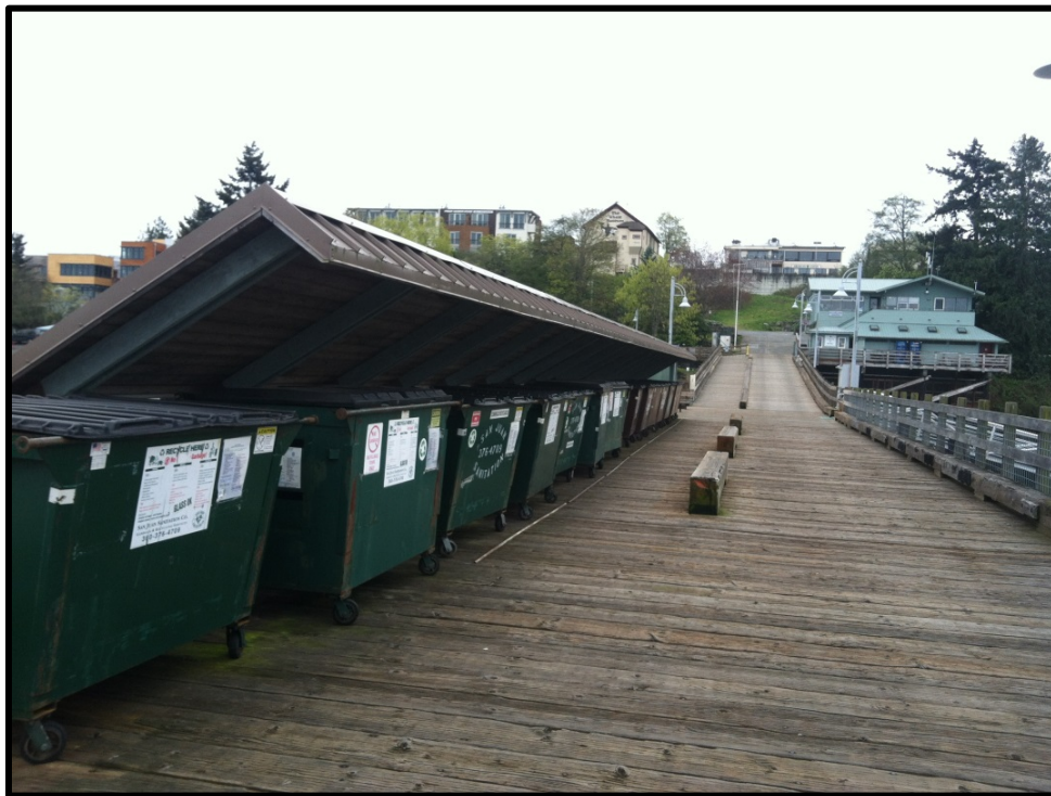
Figure 1. Covered Outdoor Storage of Solid Wastes.
