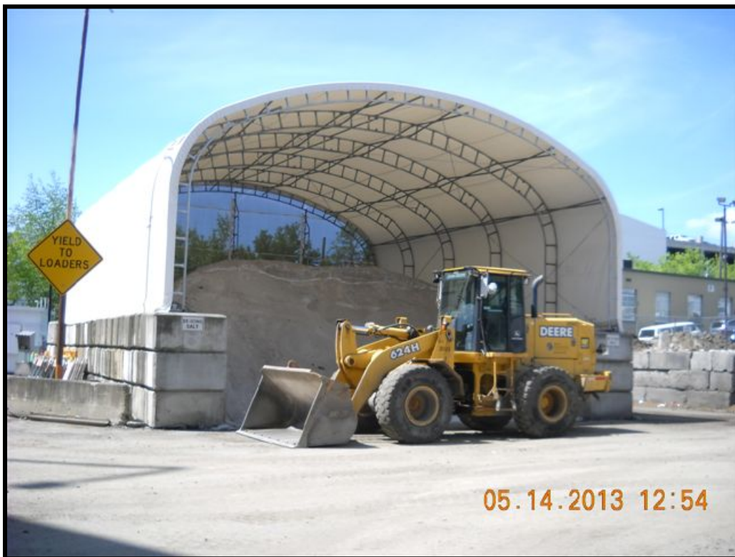
Figure 12. Covered Storage Area for Erodible Material (gravel).
