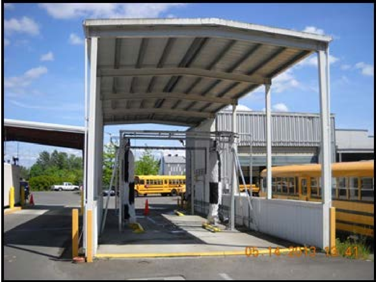
Figure 3. Car Wash Building with Drain to the Sanitary Sewer.
