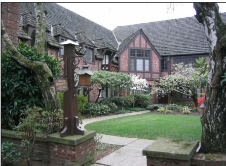
A well-defined courtyard with both a visual and physical connection to the street.
