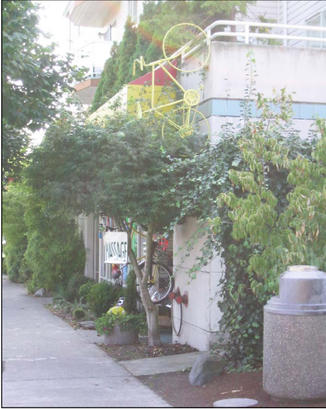
Design elements such as landscaping and creative signs add interest and give a human dimension to street-level building facades.
