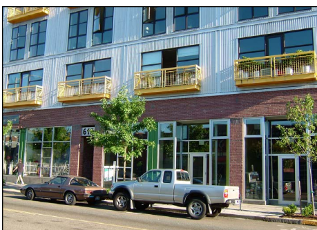
Brick, large storefront windows and masonry kick boards exhibit a sense of permanence at the street.
