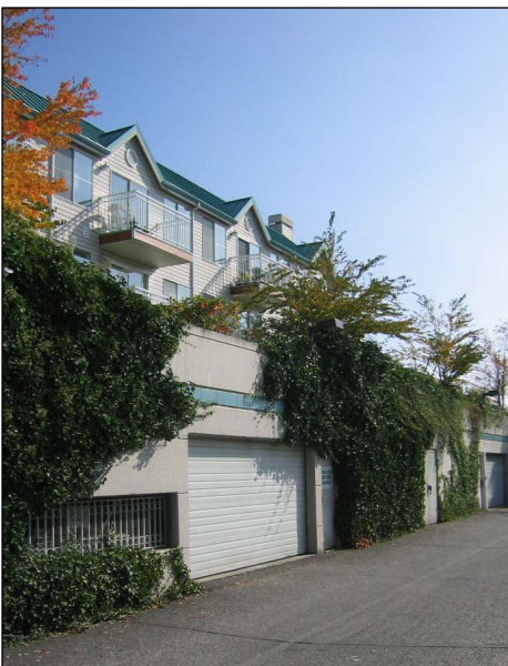
A good example of a larger, mixed-use building stepping back away from a neighboring single family area. The ground floor is further softened with generous, lush landscaping.
