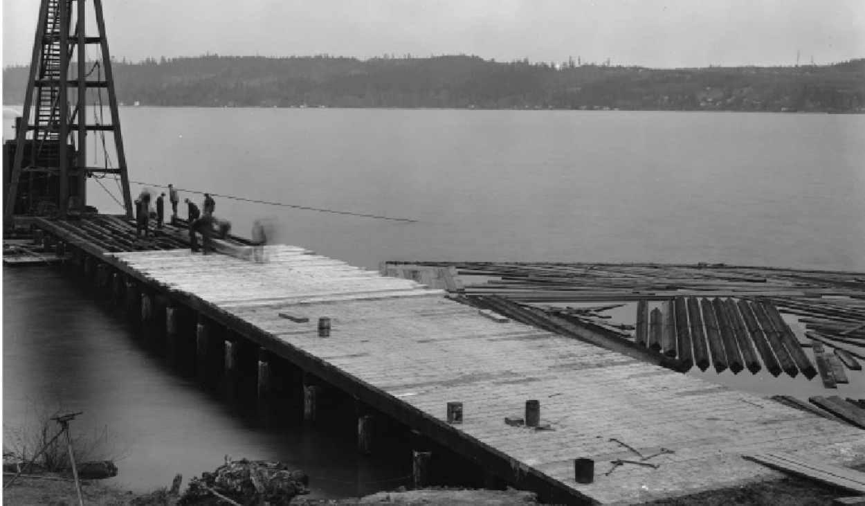
Image 4 Construction of Pier 1, later named Building 321, in 1938. 11
