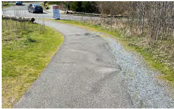
Looking west at root heave along path that connects from Lake Shore Drive NE to boat launch parking lot.
