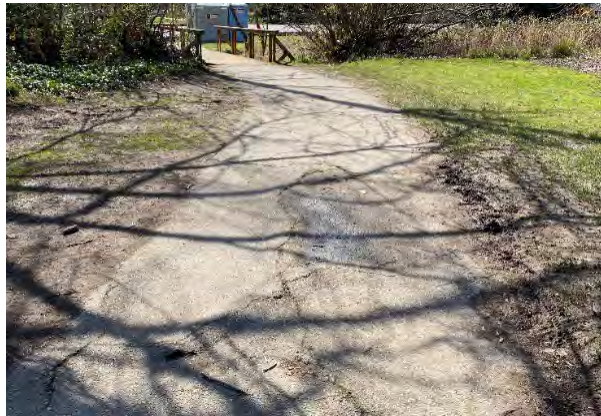
Looking south at root heave along path and bridge across creek.
