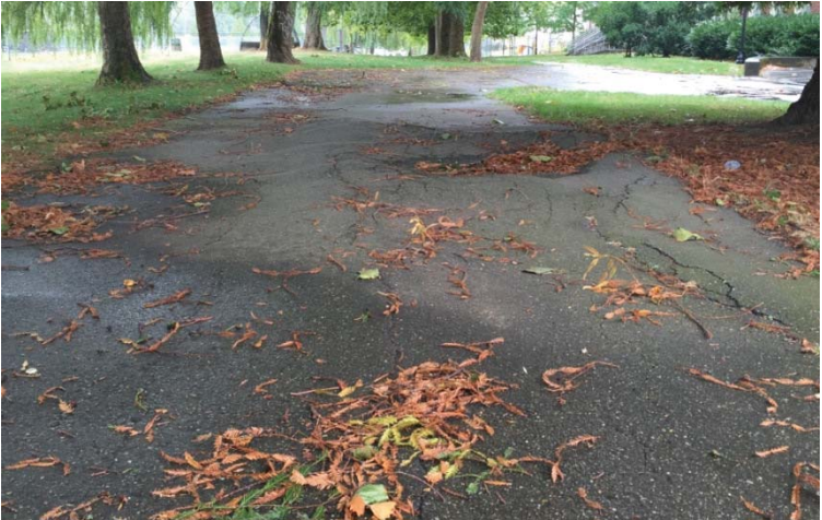
Rainier Beach Playfield path, before construction
