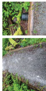
Wet Area Crossing With Culvert
