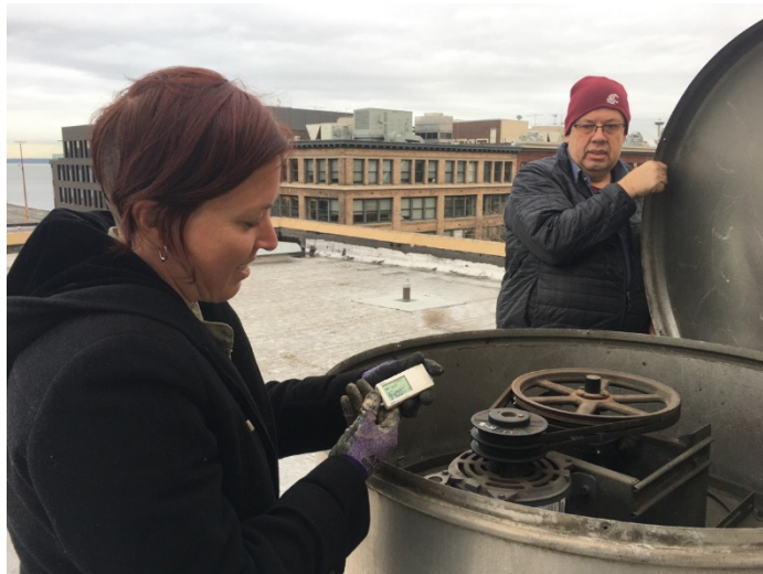
Figure 15: SBC staff and building facility manager retrieve a HOB0 UX90 motor runtime logger used to verify reduced parking garage exhaust fan schedule. It was confirmed.
