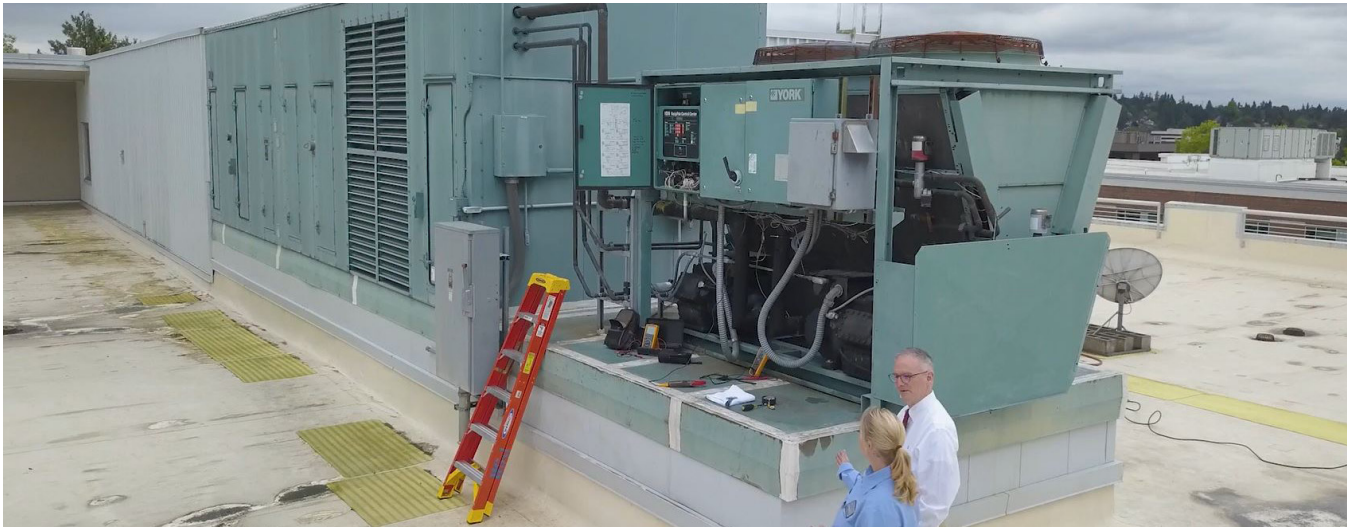
Photo by PSR Mechanical
