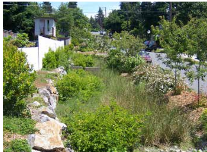
Figure 12. 110th St. Cascade Led by SPU to protect Piper's Creek
