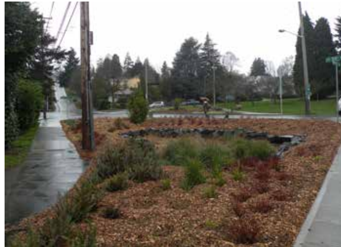
Figure 10. Roadside bioretention installed on 55th Ave. NE Installed by Seattle Department of Transportation
