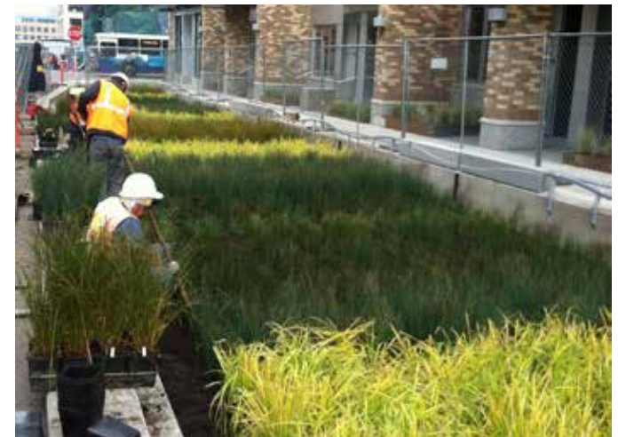
Figure 13. Swale on Yale Led by SPU in partnership with Vulcan, Inc. to protect Lake Union
