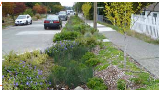
Roadside bioretention captures runoff from the road in the Sunrise Heights and Westwood neighborhoods
