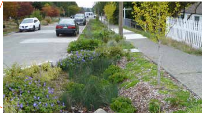
Roadside bioretention captures runoff from the road in the Sunrise Heights and Westwood neighborhoods
