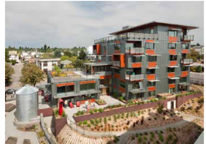
Figure 11. GreenFire Campus in Ballard Cistern and bioretention installed for Stormwater Code
