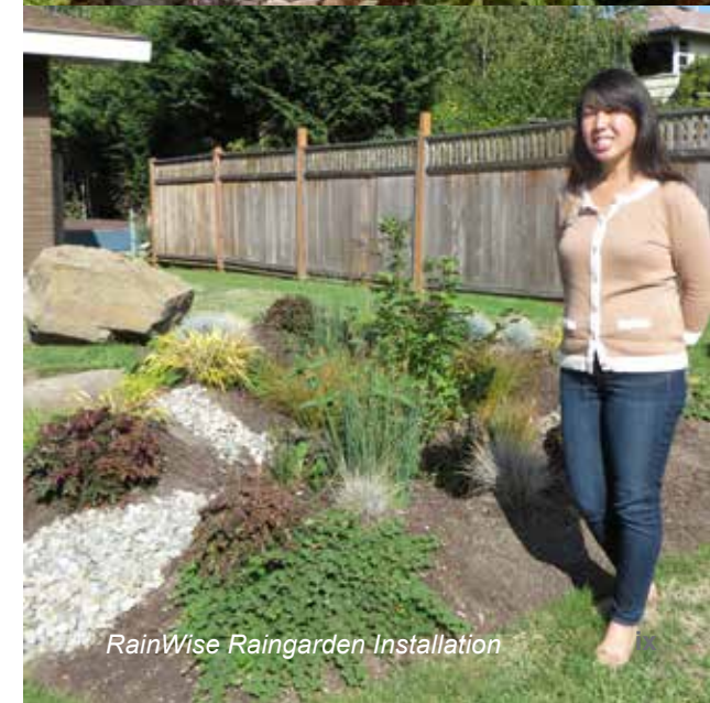
Bioretention Installation for Stormwater Code
