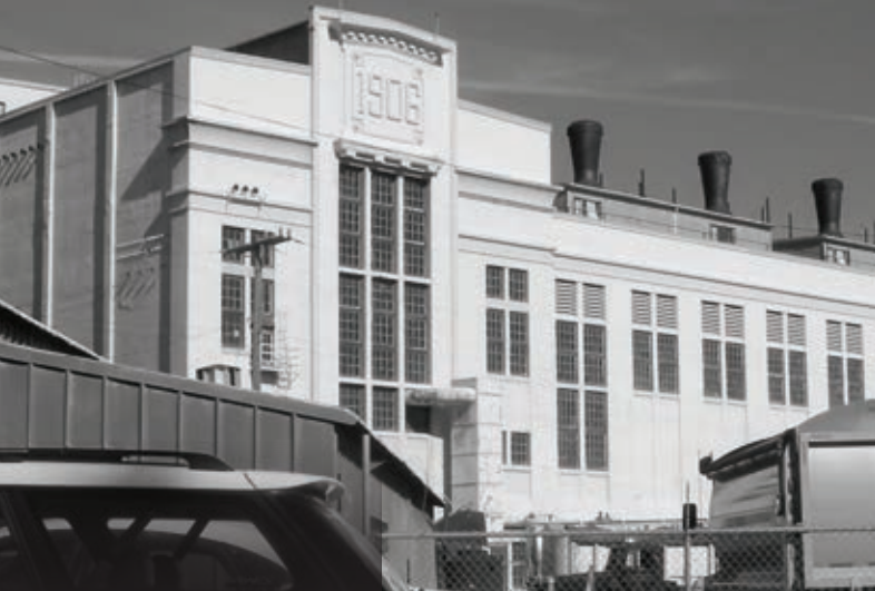
Georgetown Steam Plant (1906) / Georgetown PowerPlant Museum. Sawirka Sawirka: Joe Mabel
