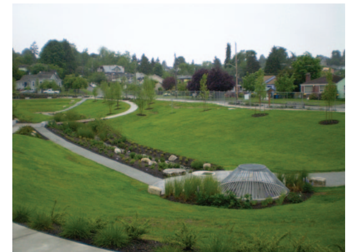
This above-ground stormwater holding area at 30th Ave E and E John Street operates as community open space when not in use. Photo by Benjamin Lukoff.
