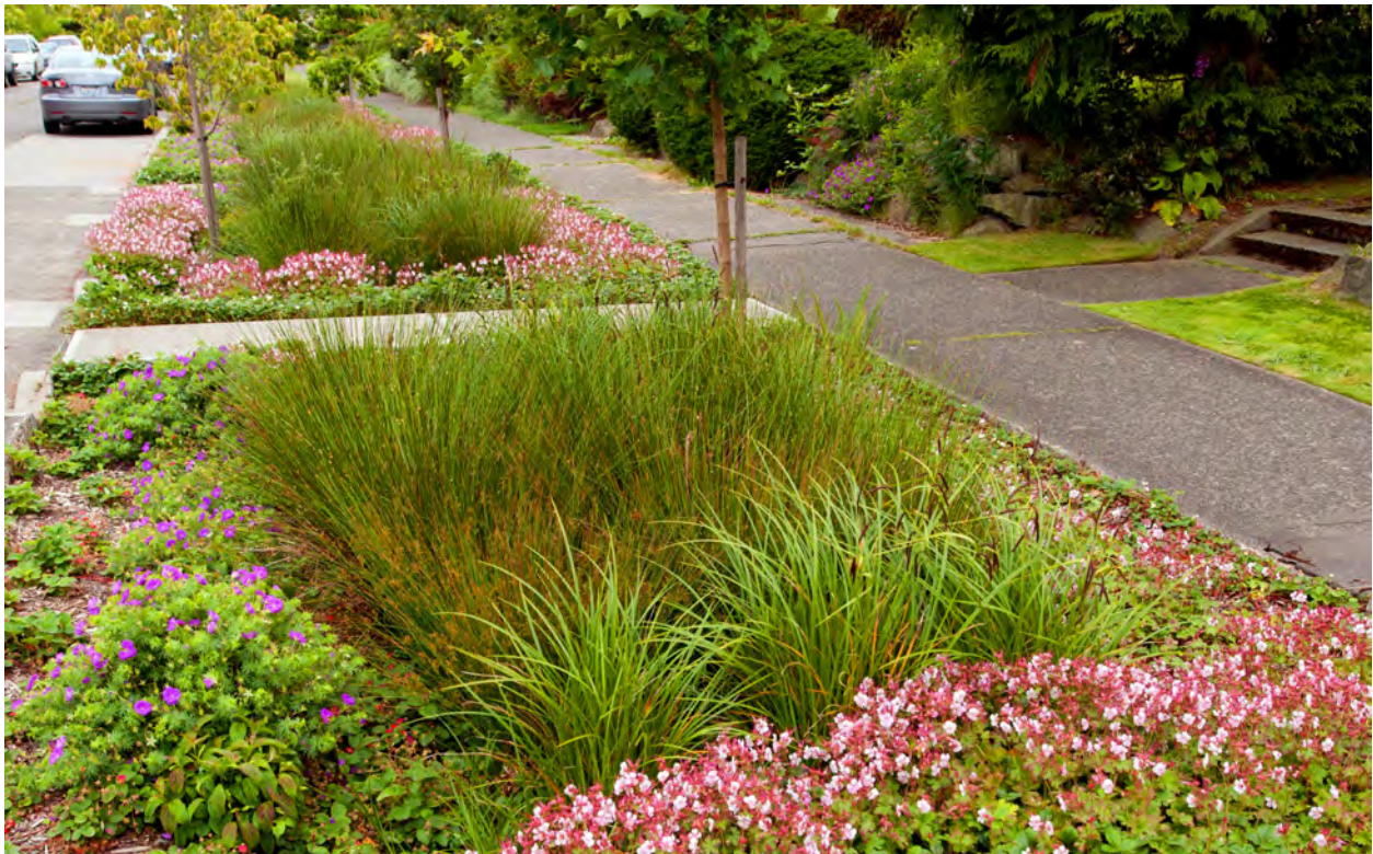
Green Stormwater Infrastructure in Ballard. (Image: Seattle Public Utilities)
