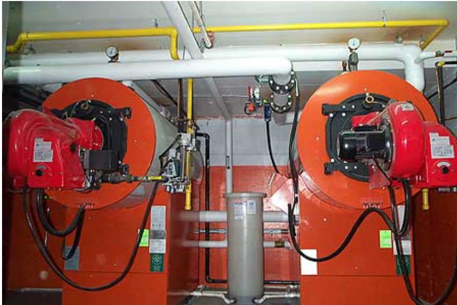
Figure 10 – CHP Mini-Plant in Lonsdale
