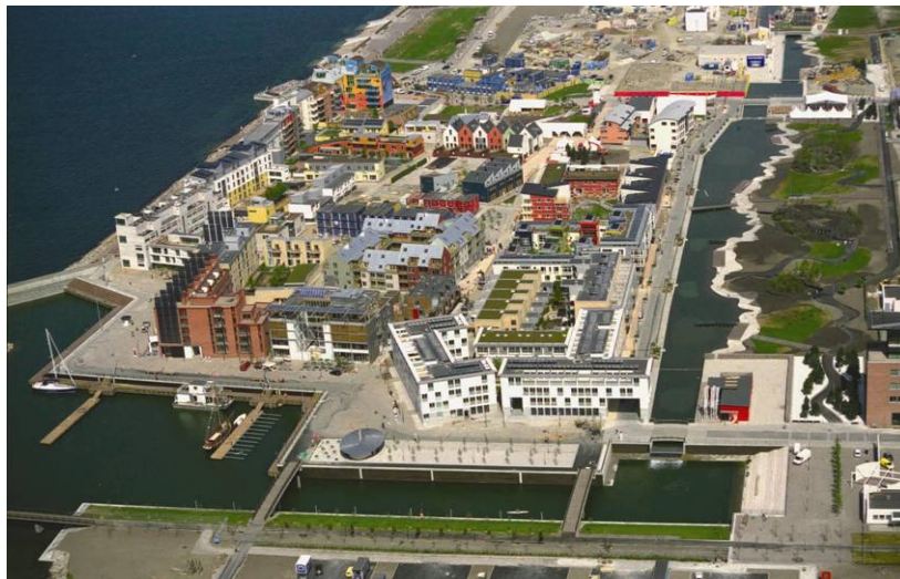
Figure 5 – Aerial View of Western Harbor
