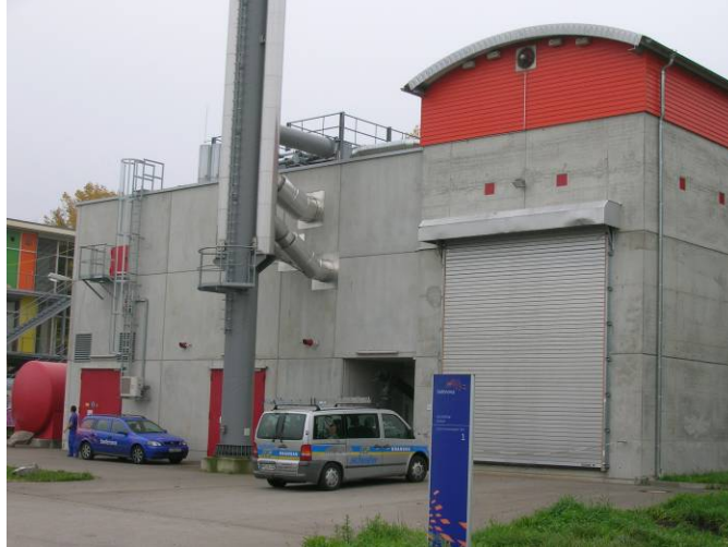
Figure 8 – Wood Chip Fired Neighborhood Scale CHP Plant in Vauban
