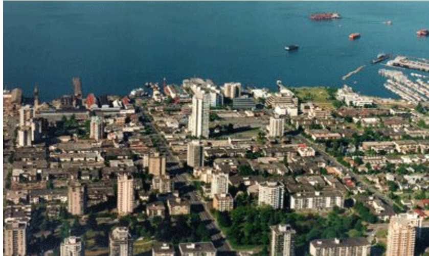
Figure 9 – Lonsdale District Energy System
