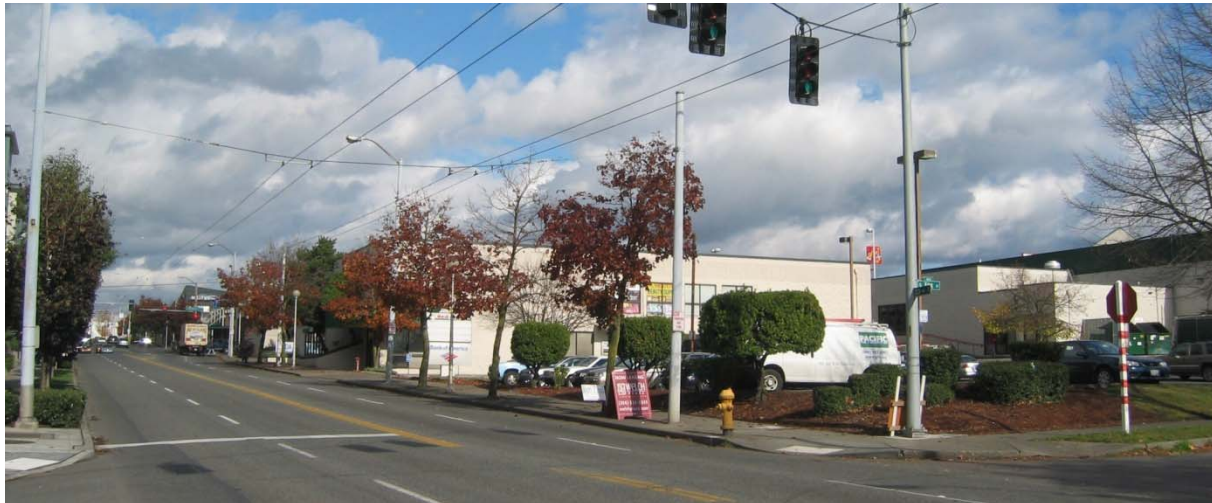
View of Promenade South from 23 rd Avenue, looking northeast.
