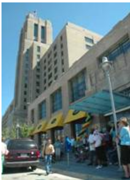
Exterior Renovated Sears Building
