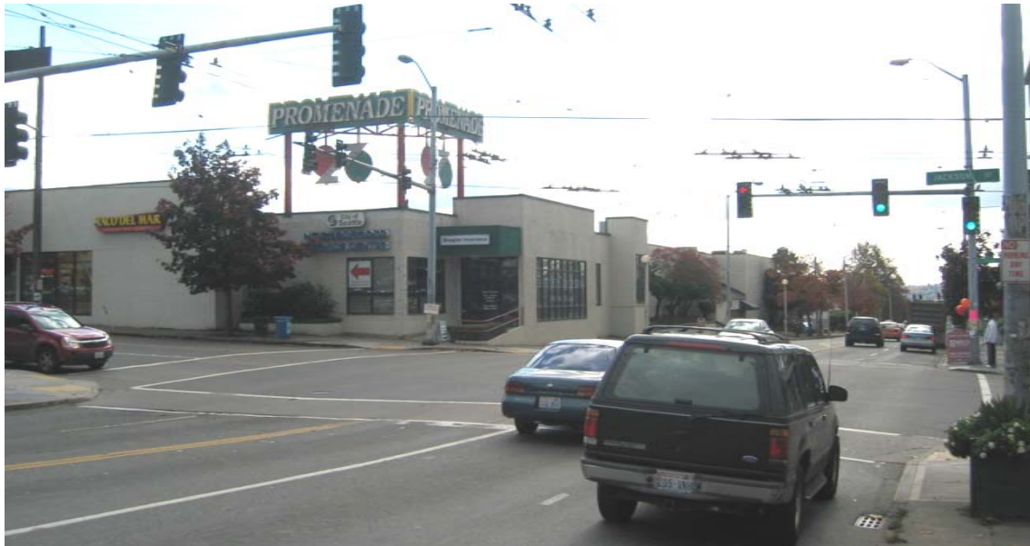
View of Promenade South from 23 rd Avenue, looking southeast across Jackson Street intersection.
