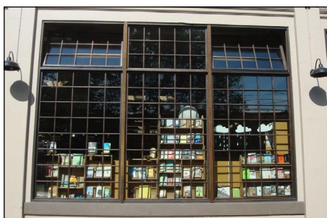
Window trim detailing.
