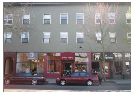
Transparent windows, retail modules and consistent entrances lend to human-scaled streetscape.
