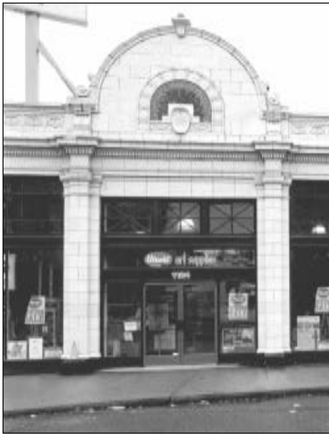
Context—pilasters, arched terracotta cladding, parapet
