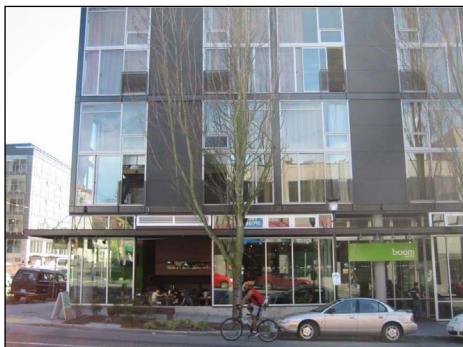
Use of modern materials
