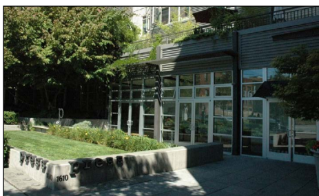
The courtyard of Press Condominiums provides a residential open space amenity on Belmont Avenue E.
