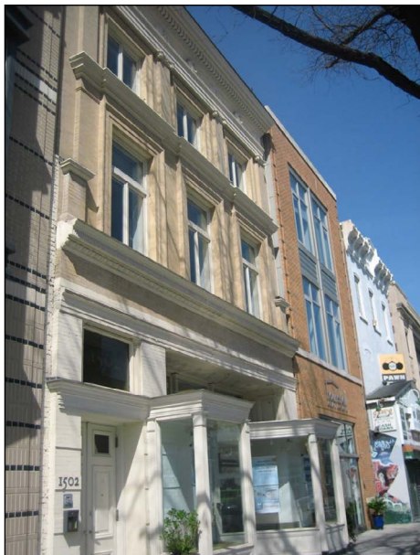
From this vantage point on the sidewalk, the upper story addition is not visible from the street, due to its setback.
