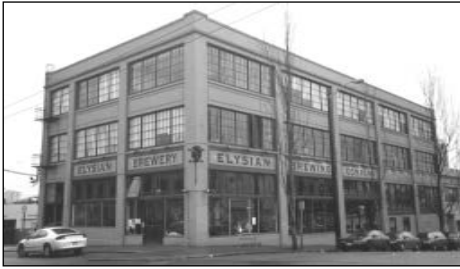
Context—light industrial signage and building design; tall windows
