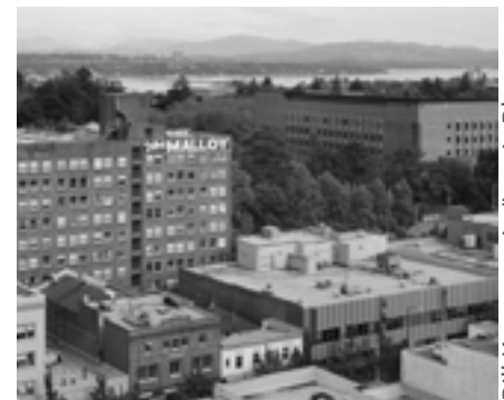
Residential and institutional density in the U District presents opportunities to capture and reuse waste heat.
