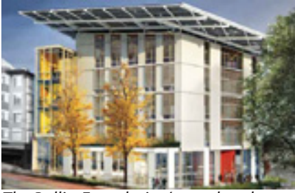
The Bullitt Foundation's new headquarters in Capitol Hill are built to meet the rigorous standards of the Living Building Challenge. Among other notable features, the building harvests all of its own energy and water.
