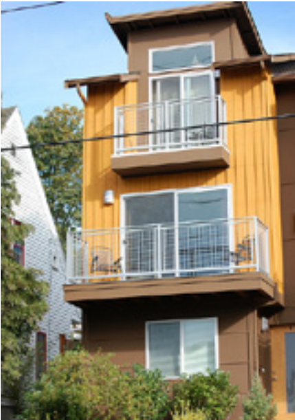
Lowrise and midrise residential buildings help make a transition from single-family to higher density areas.
