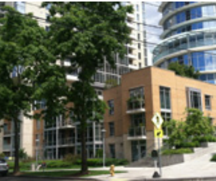
With good design at the ground level, highrise buildings can achieve a “human scale” pedestrian environment. (First Hill)
