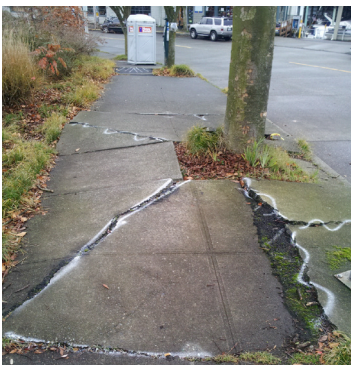
Cracked and narrow sidewalk
