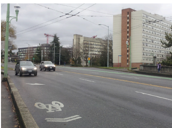
North end of University Bridge
