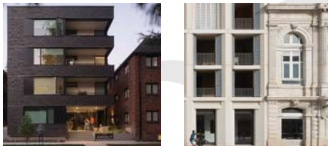
Two examples of new development reflecting context through the use of related materials, datum lines, and horizontal and vertical elements.
