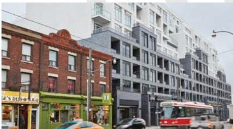
New development responds to datum line of adjacent existing building by stepping back at the second story and again at the upper levels.
