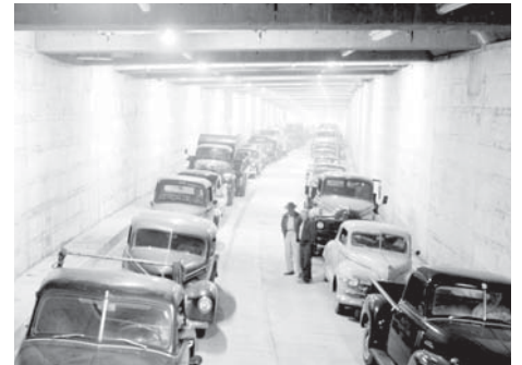
Battery Street Tunnel circa 1950. Image: Seattle Municipal Archives.
