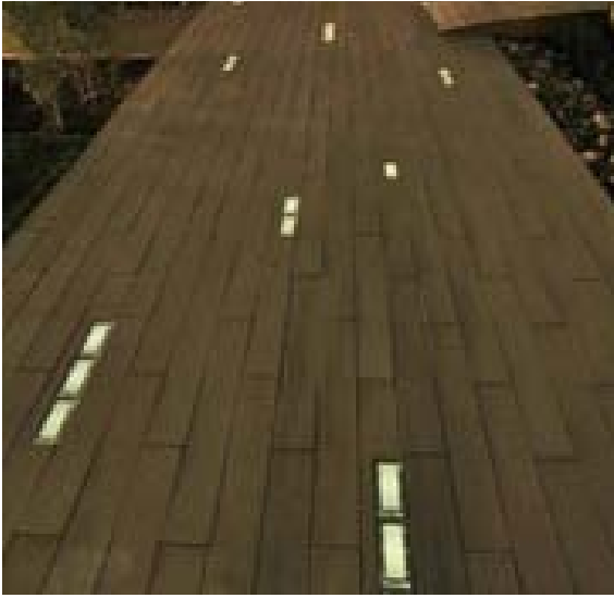
LED lighting pavers integrated in a pathway
