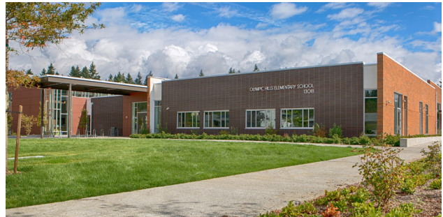
Figure 22. Olympic Hills Elementary School (McGranahan Architects)
