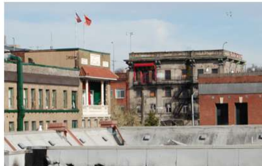
Unreinforced masonry buildings in the Chinatown-International District.
