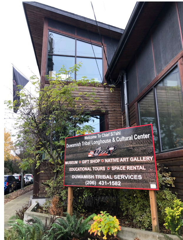
Duwamish Tribal Longhouse and Cultural Center
