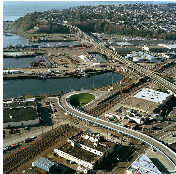
W Galer St Overpass and the Magnolia Bridge
