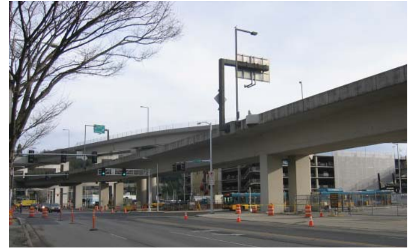
View of I-90 ramps from South-of-Dearborn Area
