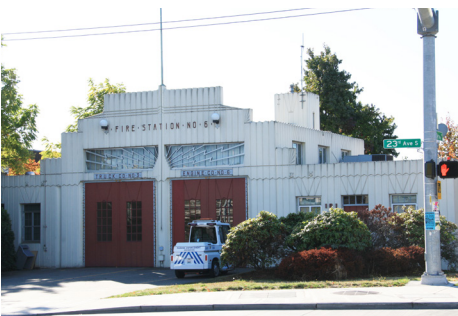
Fire Station 6, a historic landmark at 23rd Ave and Yesler Way
