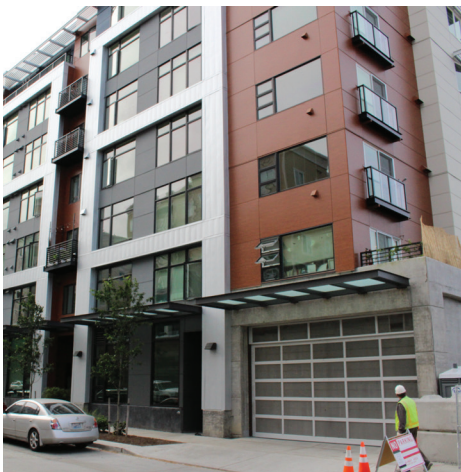
Carefully located and designed parking access won't dominate the building facade.
