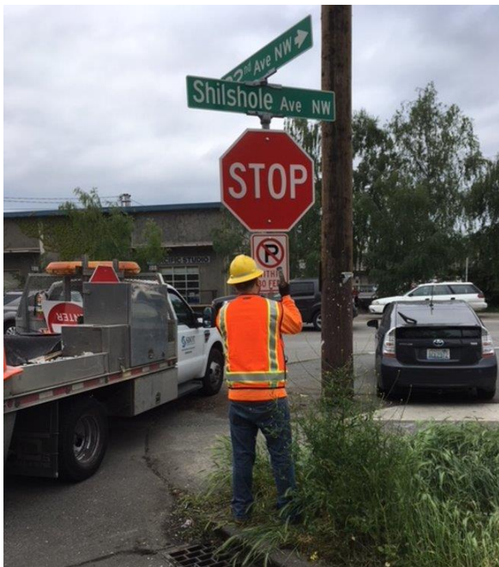
SDOT Employee repairs street sign in Ballard.
