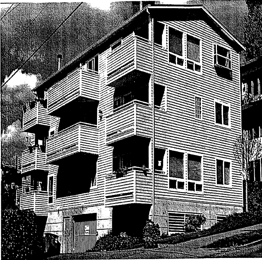
"Stuck-on" balconies like these should be avoided. Balconies should be integrated into the building's modulation.
