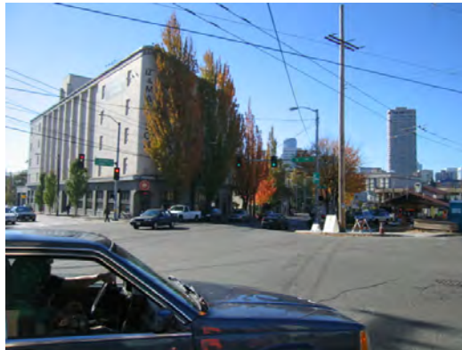
Self-Storage Building at Madison and 12th
