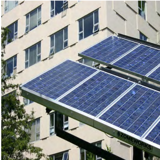
Photovoltaics on E. Cherry St.
