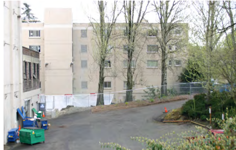
Area behind Self-Storage Building
