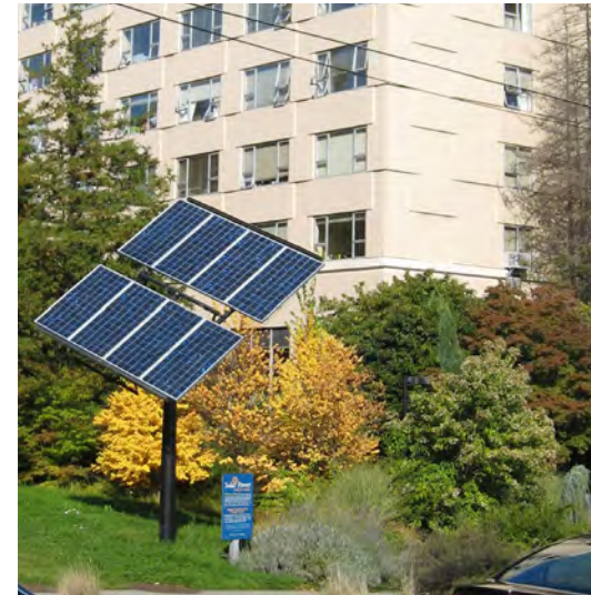
Solar Photovoltaic Array In Front Of Bellarmine Residence
