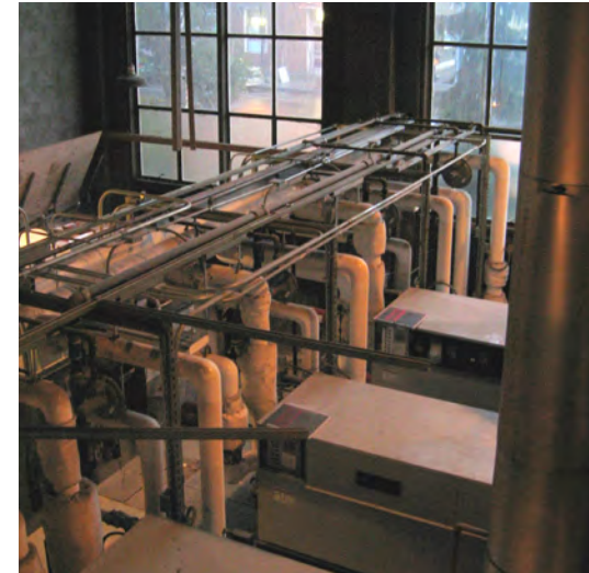
Thermal Energy Distribution System
