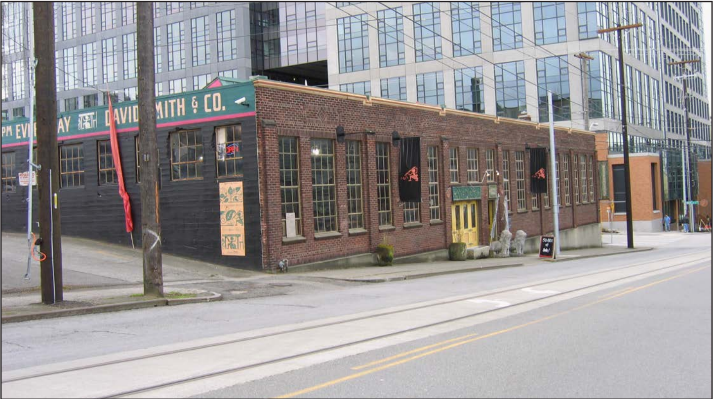
Figure 22 • North façade viewing southwest
