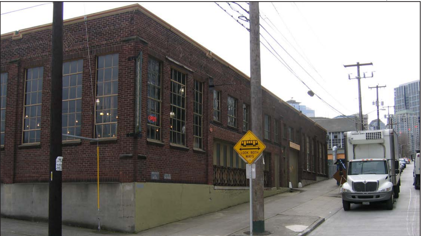
Figure 27 • West façade, viewing southeast
