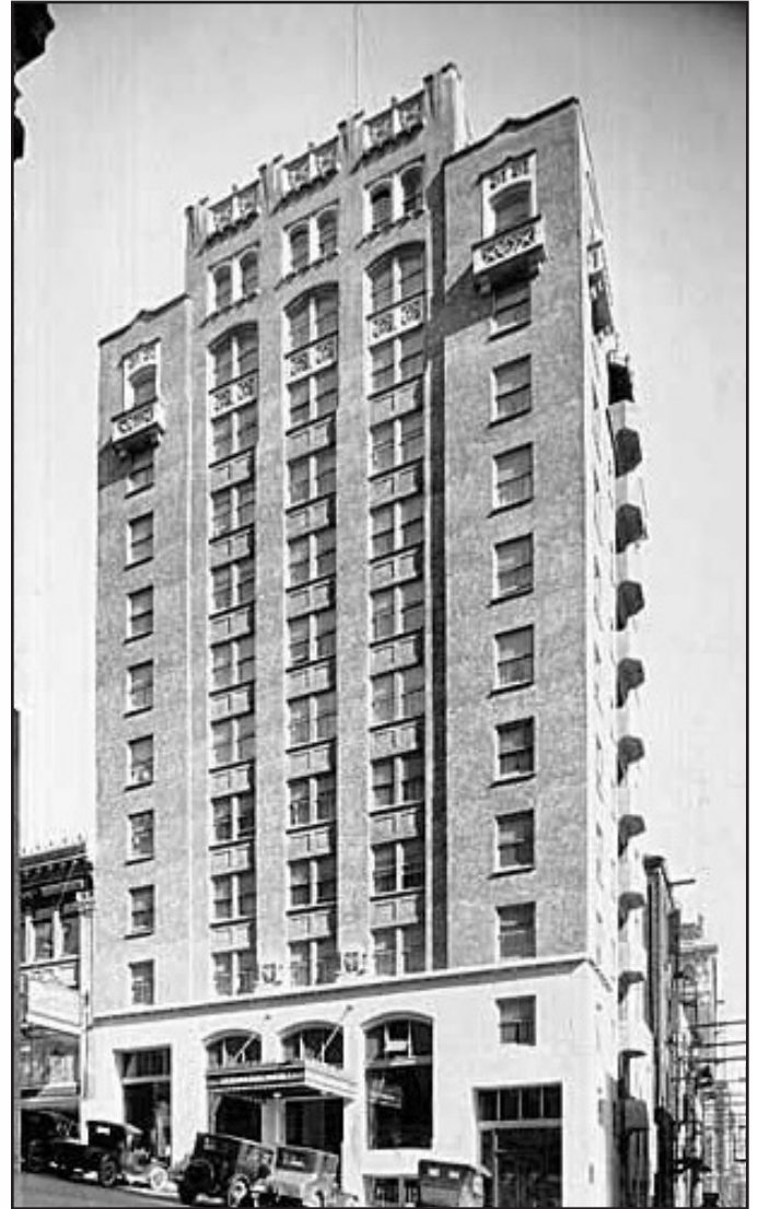
Figure 67 • Continental Hotel (ca. 1927, Stuart & Wheatley, demolished)
