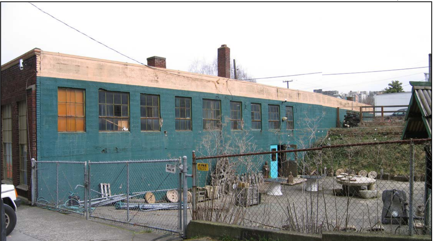
Figure 29 • South façade viewing northeast
