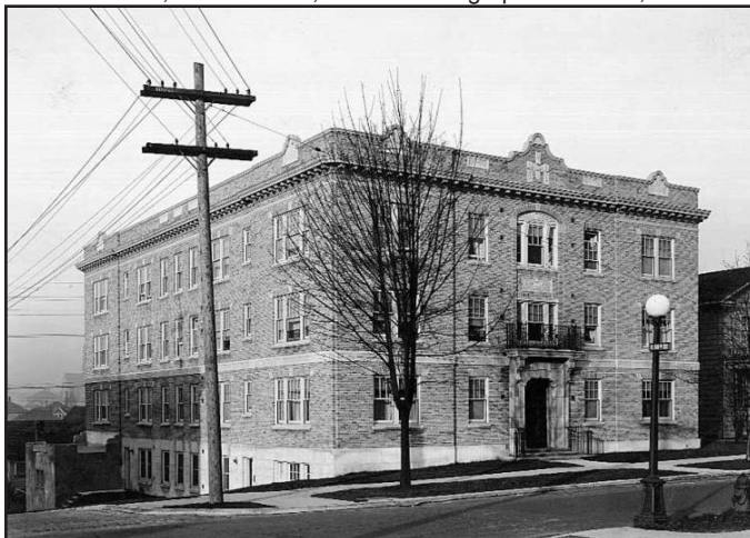
Figure 72 • Davison Apartments (1926, Stuart & Wheatley)
