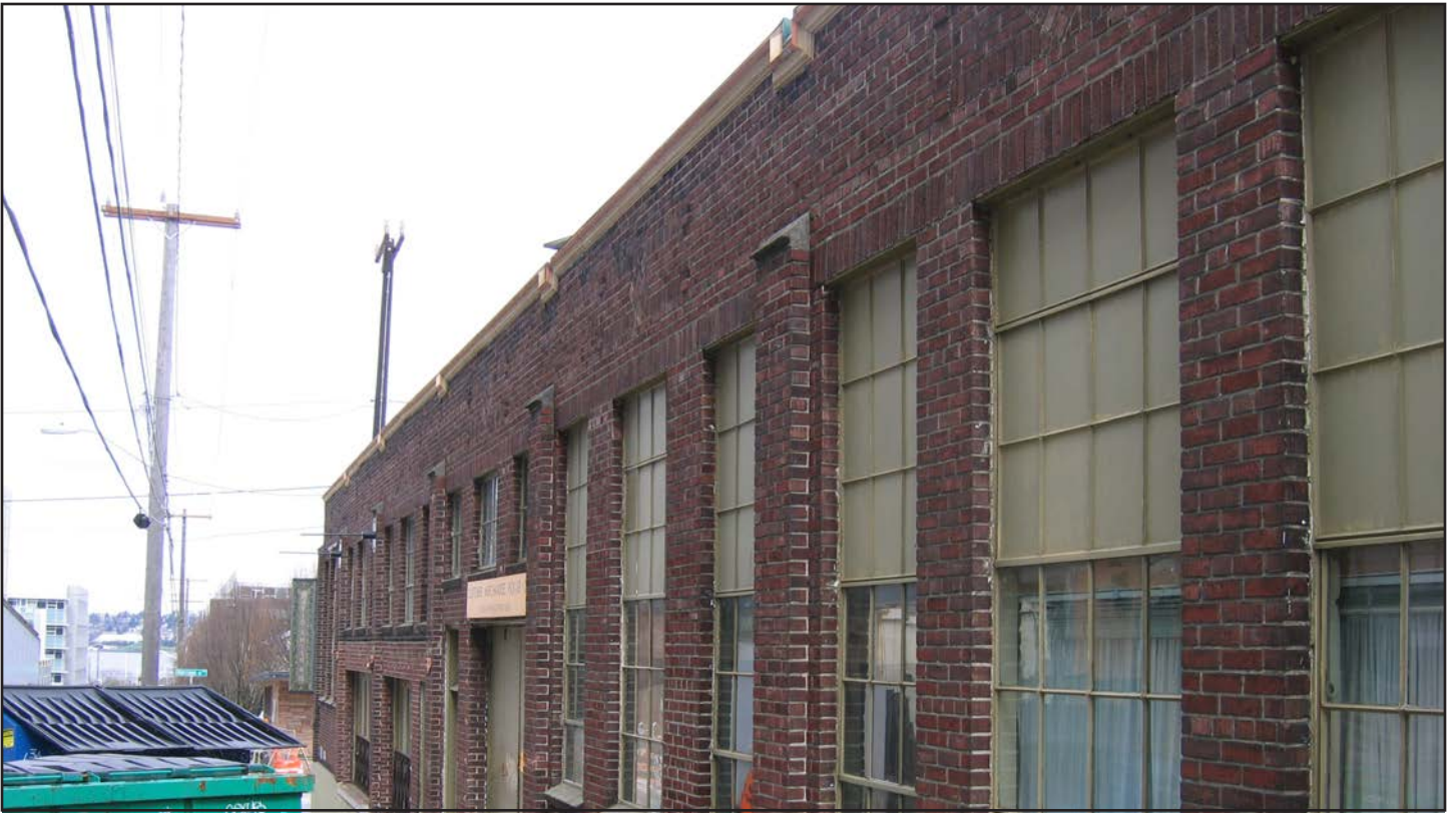
Figure 28 • West façade, viewing northeast
