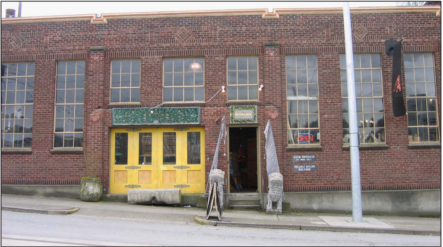
Figure 24 • North façade, central portion
