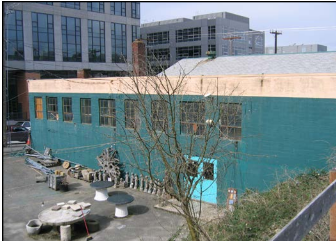
Figure 18 • Viewing northwest from adjacent alley at subject building's south façade
