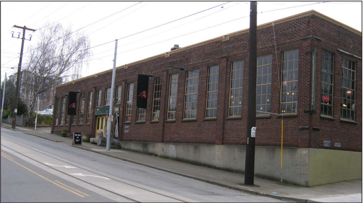
Figure 26 • North façade, viewing southeast
