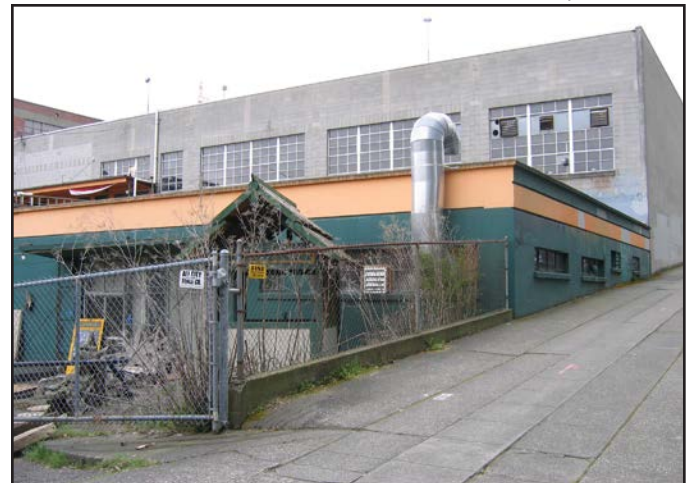
Figure 21 • Viewing southeast from Boren Avenue N at adjacent building
