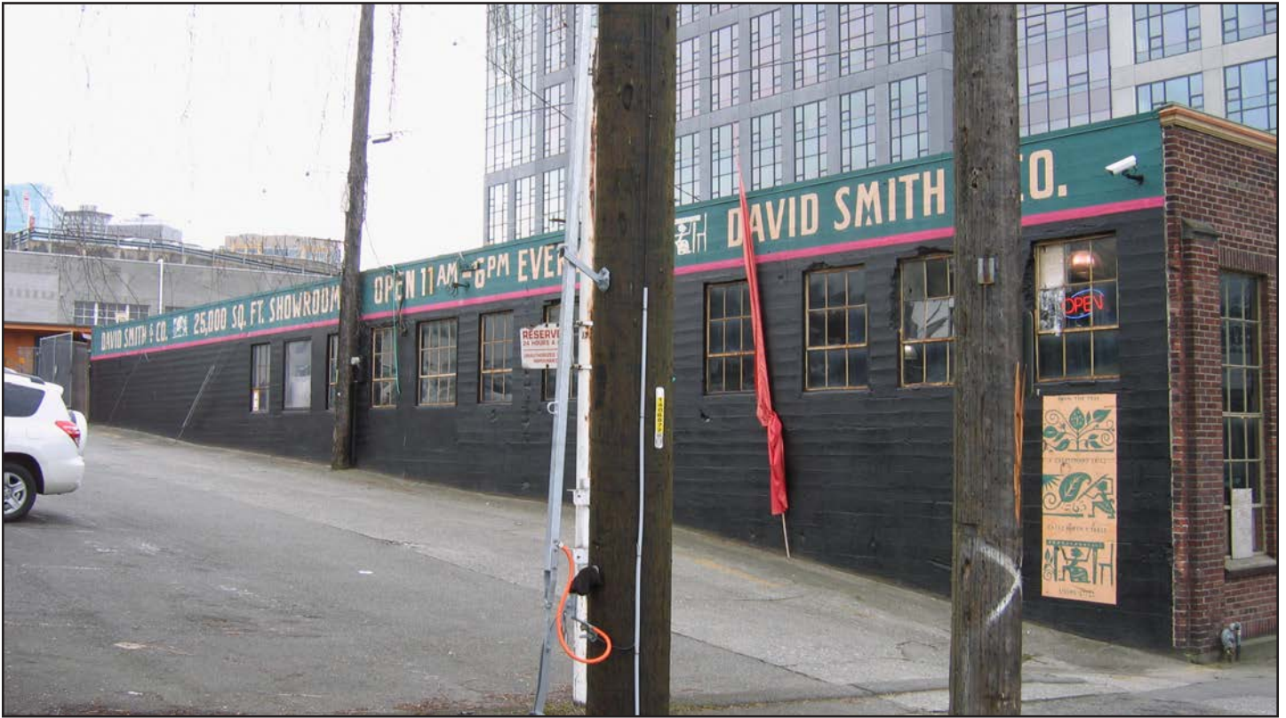
Figure 30 • East façade viewing southwest (alley)
