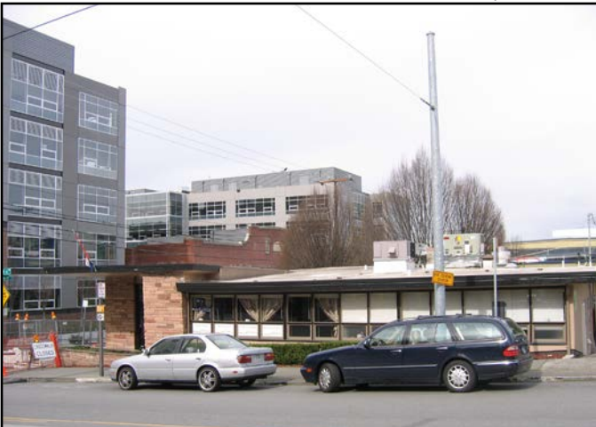
Figure 6 • View E, viewing northwest from N Harrison Street, east of Boren Avenue N
