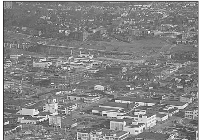
Figure 57 • South Lake Union viewing toward freeway construction from Space Needle, 1962
