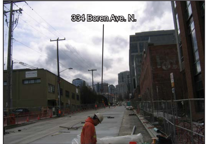
Figure 5 • View D, viewing south from corner of Boren Avenue N and N Republican Street
