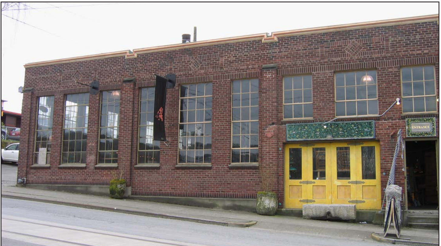
Figure 23 • North façade, eastern portion
