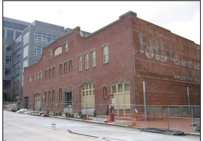
Figure 12 • Van Vorst Building (413-421 Boren Avenue N)
