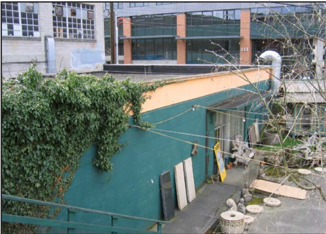
Figure 20 • Viewing southwest from adjacent alley at adjacent building
