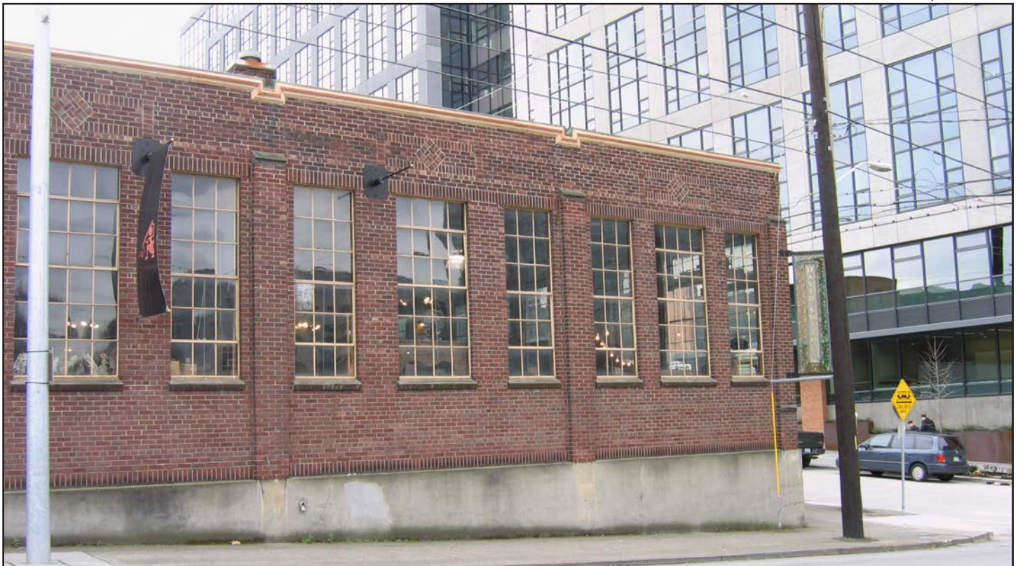
Figure 25 • North façade, western portion
