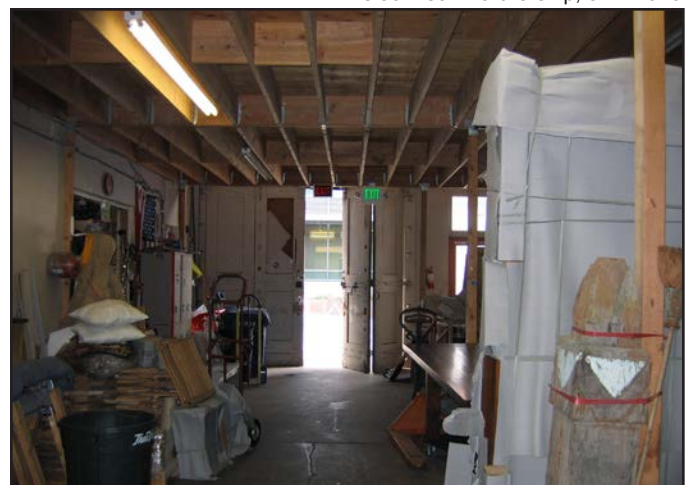
Figure 36 • Interior, main floor, rear portion, viewing south
