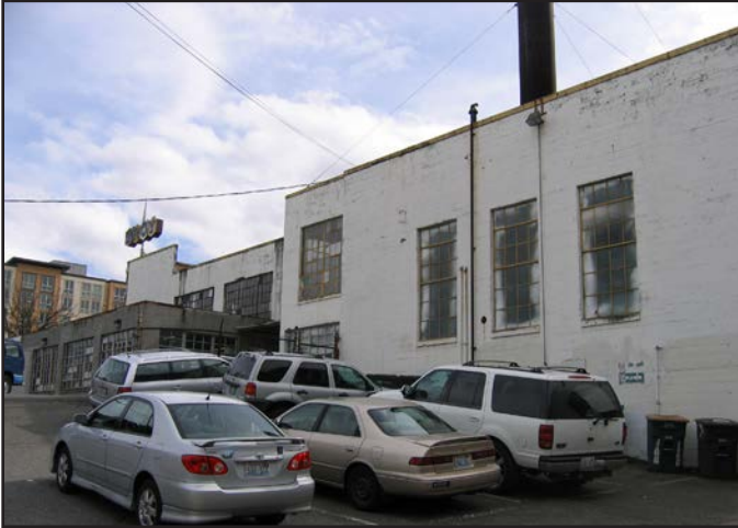
Figure 16 • Viewing southeast from adjacent alley
