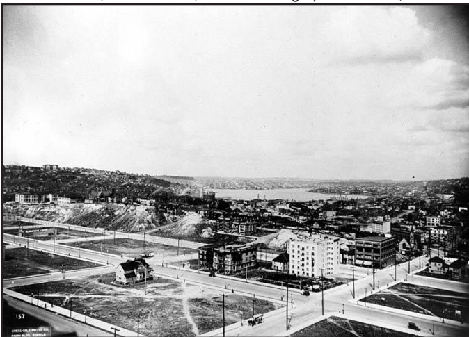
Figure 49 • Final Denny Re-grade viewing northeast, ca. 1930
