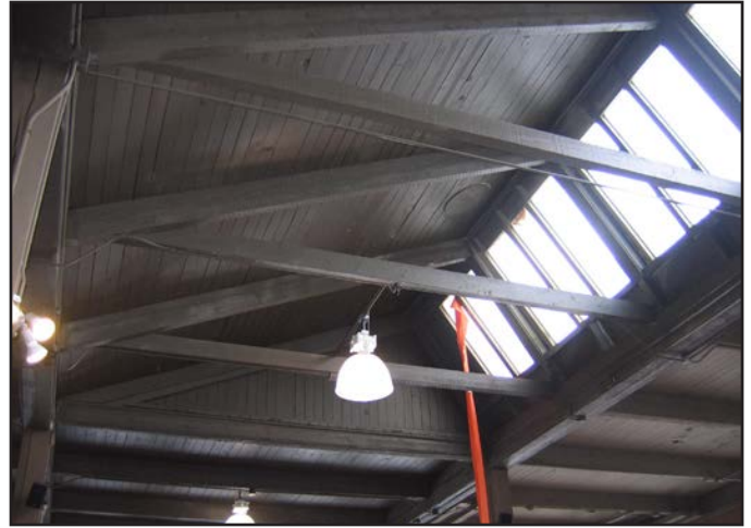
Figure 32 • Interior, roof monitor, viewing northwest
