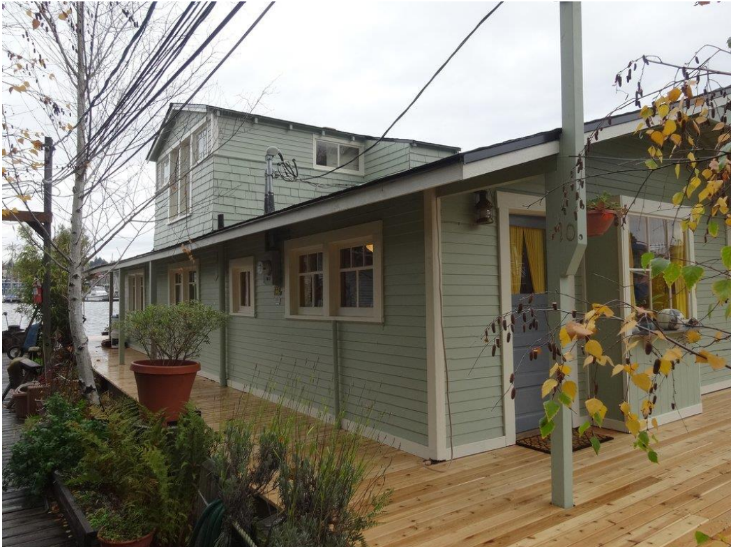
C23. View northeast, showing the west side and the kitchen entrance on the south side. (Nov. 20, 2020)
