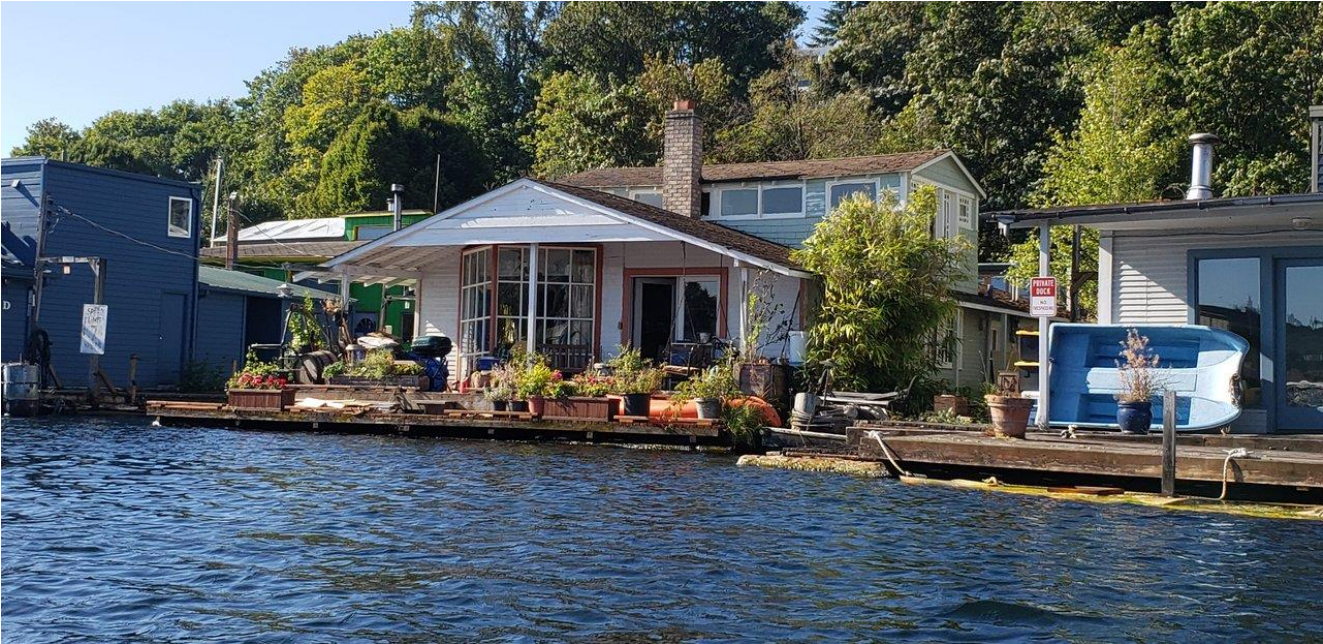
C6. View south, from the water, of the north (primary) and west sides
