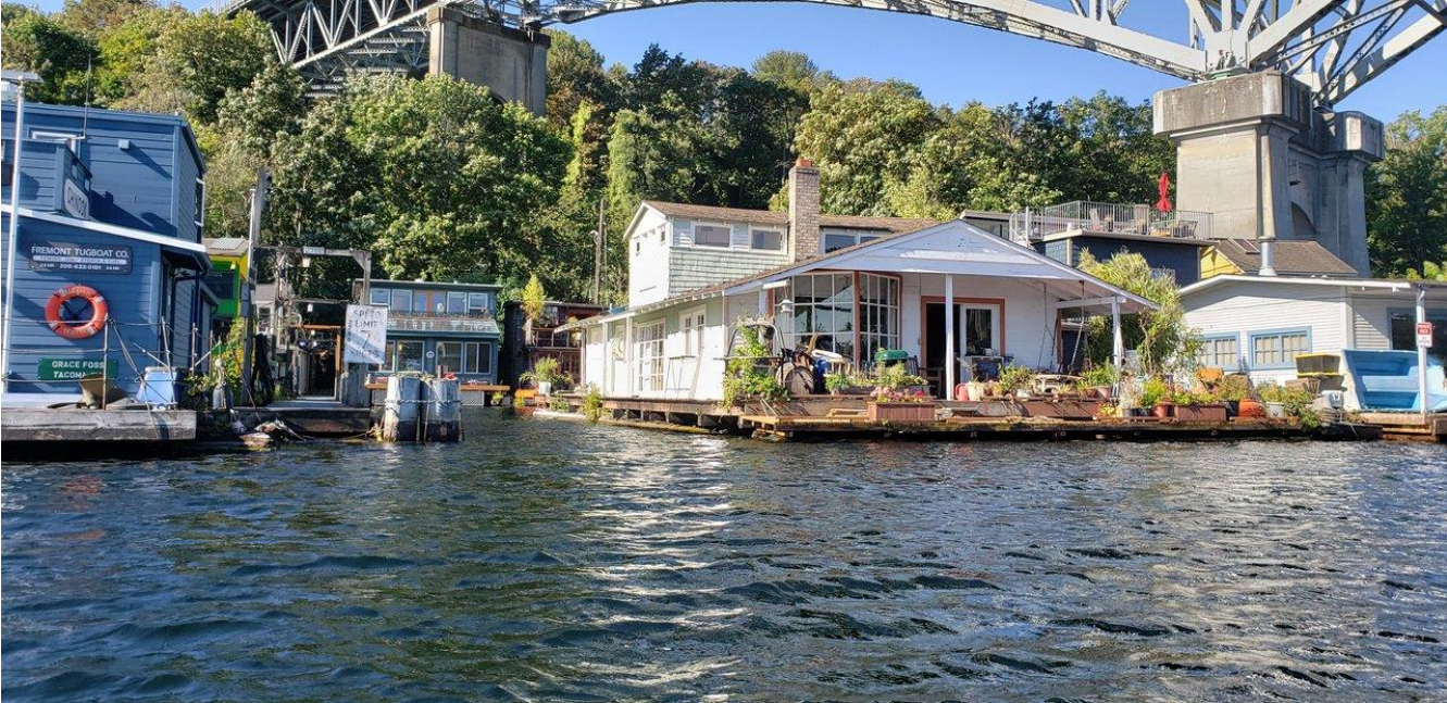
C8. View south, from the water, of the primary north elevation.
