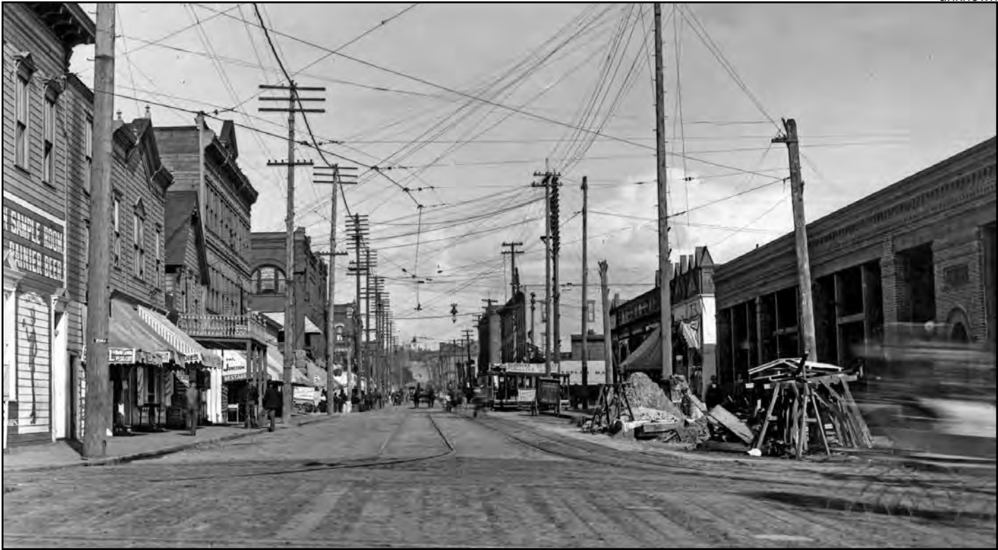
Figure 42. Hahn Building under construction, ca. 1897
