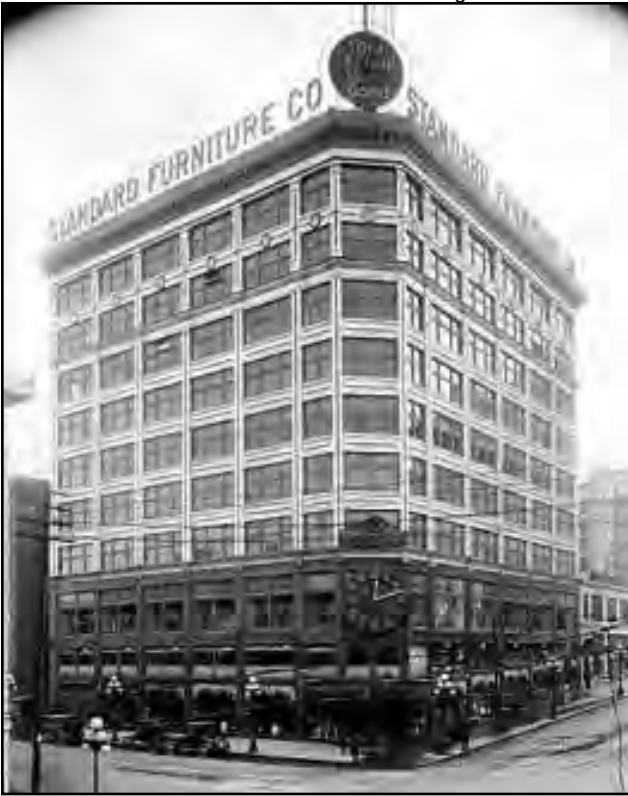
Figure 32. Standard Furniture Building (1905-07, A. Warren Gould) at Second Avenue and Pine Street
