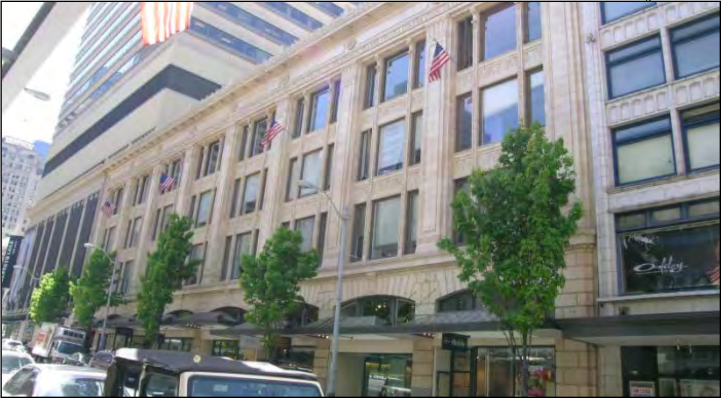
Figure 68. The Decatur Building, 1521 6th Avenue (1921-22, Henry W. Bittman, City of Seattle Landmark)
