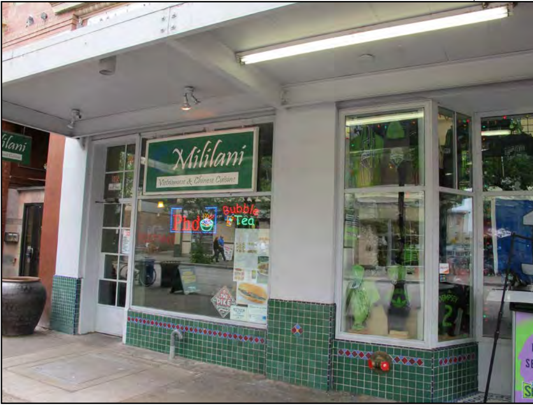
Figure 13. Hahn Building, northern façade storefront, western end
