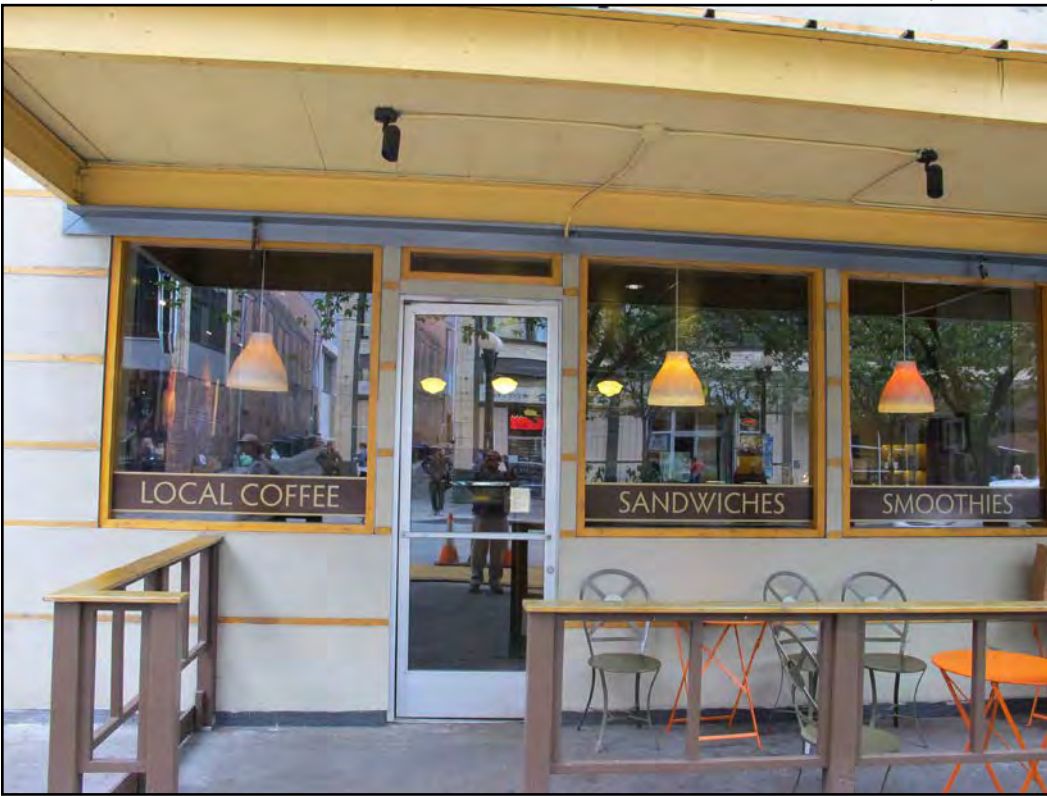
Figure 14. Hahn Building, northern façade storefront, eastern end
