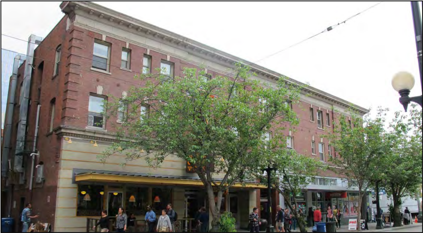
Figure 12. Hahn Building, northern façade
