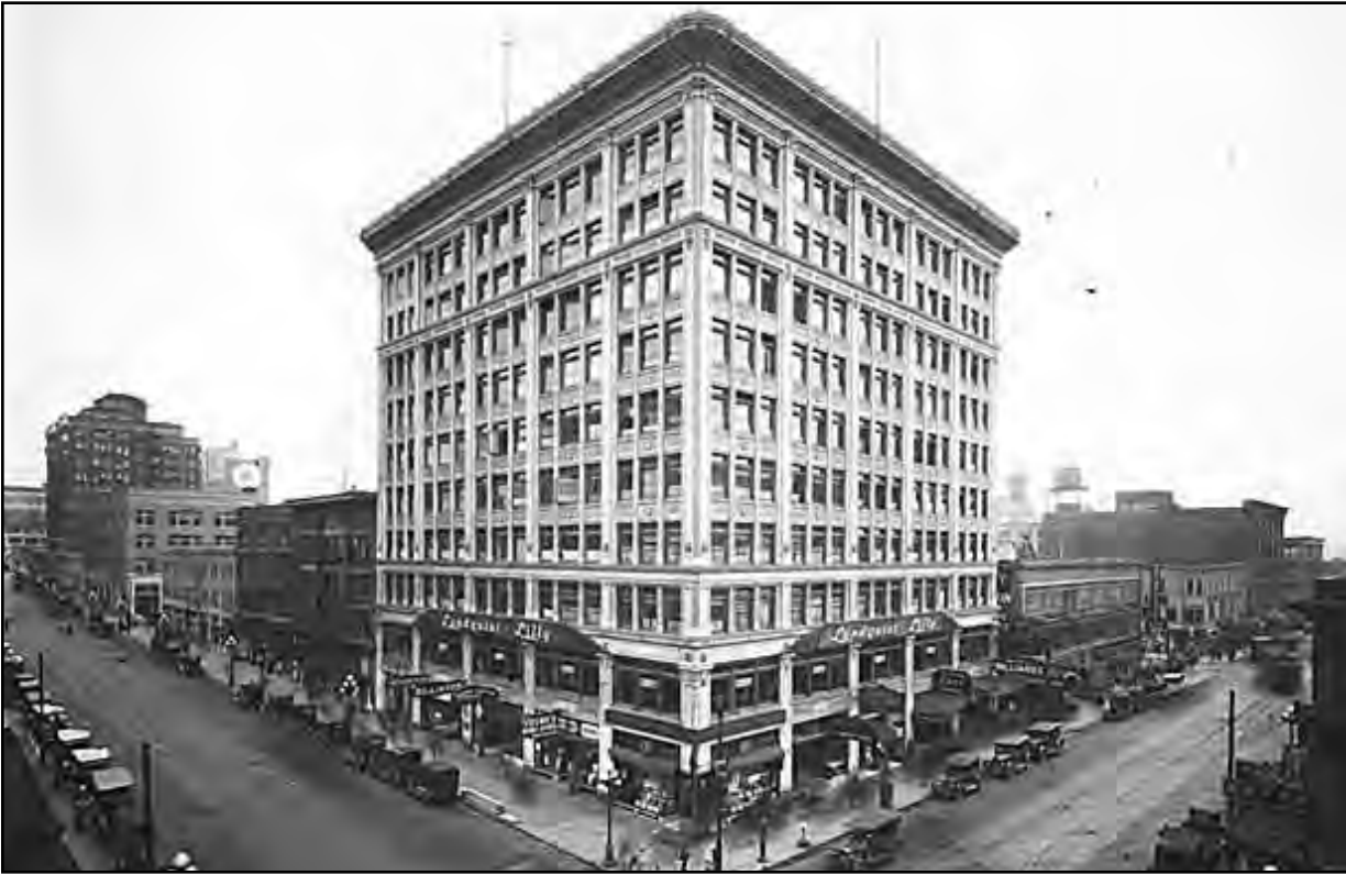
Figure 38. The Joshua Green Building (1912, John Graham Sr.) at Fourth Avenue and Pike Street
