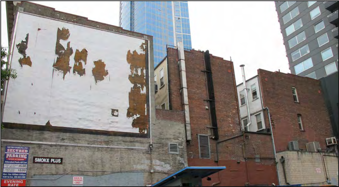
Figure 18. Hahn Building, southern façade
