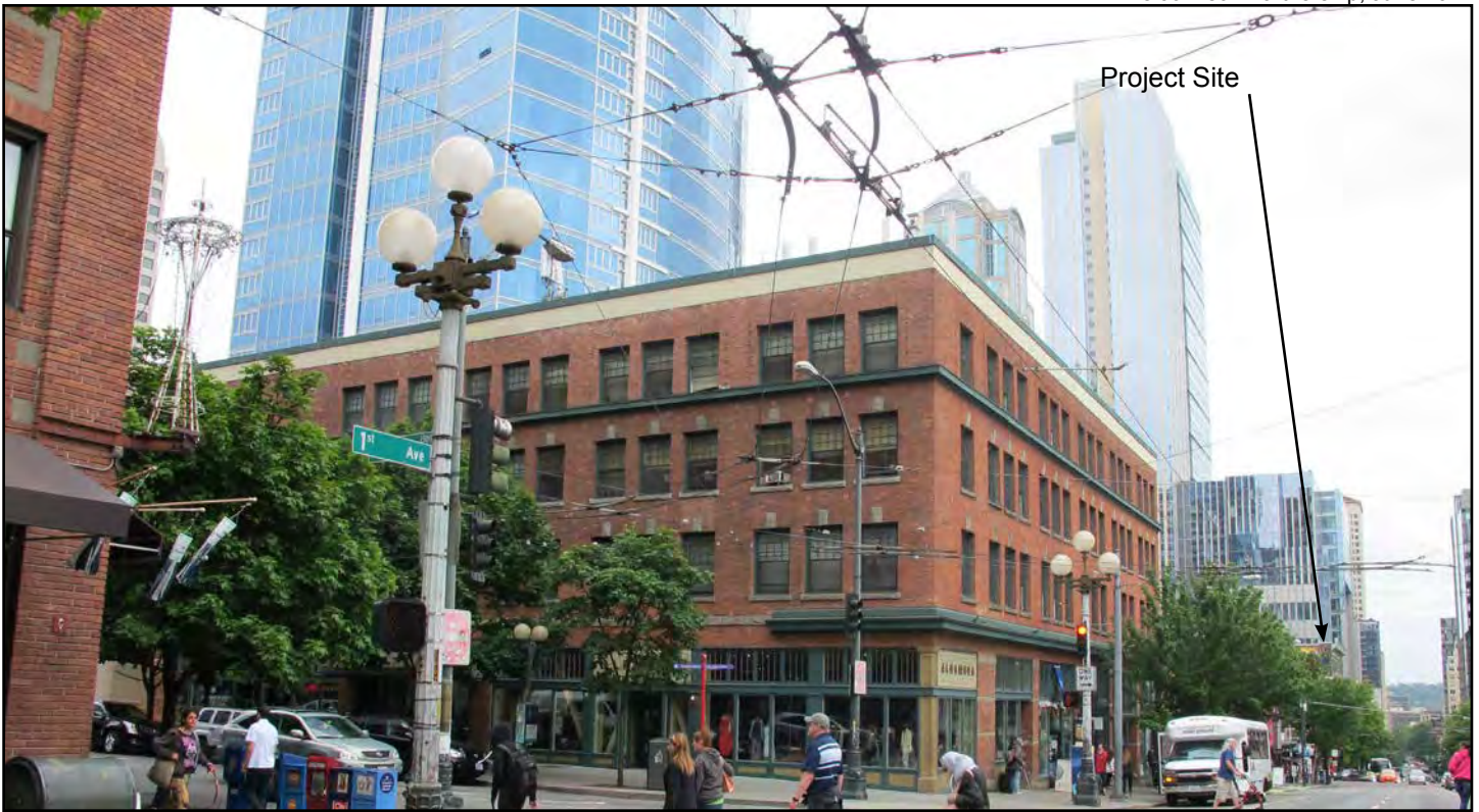
Figure 6. View C—Viewing south down First Avenue
