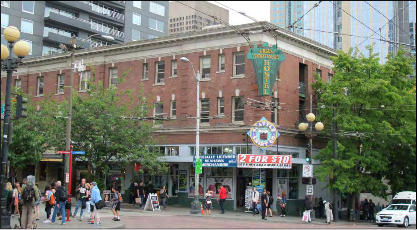
Figure 11. Hahn Building, northern façade
