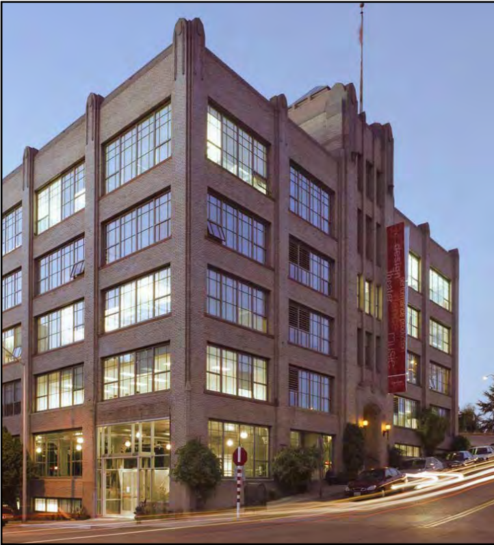
Figure 72. Volker Building 2101 9th Avenue, now Cornish College of the Arts (1928, Henry W. Bittman, National Heritage Register)
