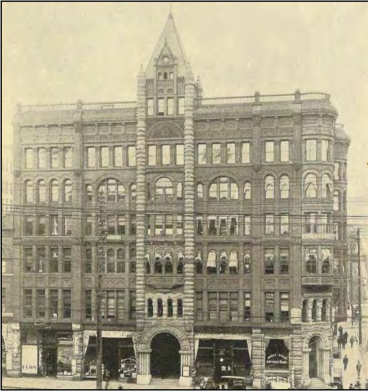
Figure 60. Pioneer Building (1889-91, Elmer H. Fischer)
