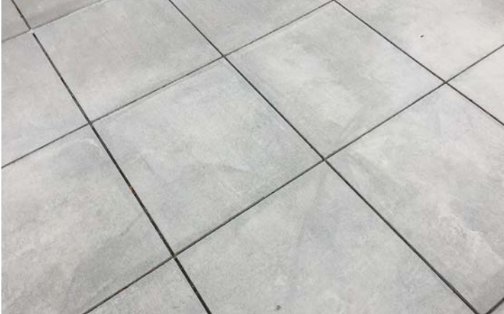
Concrete paving with sawcut joints
