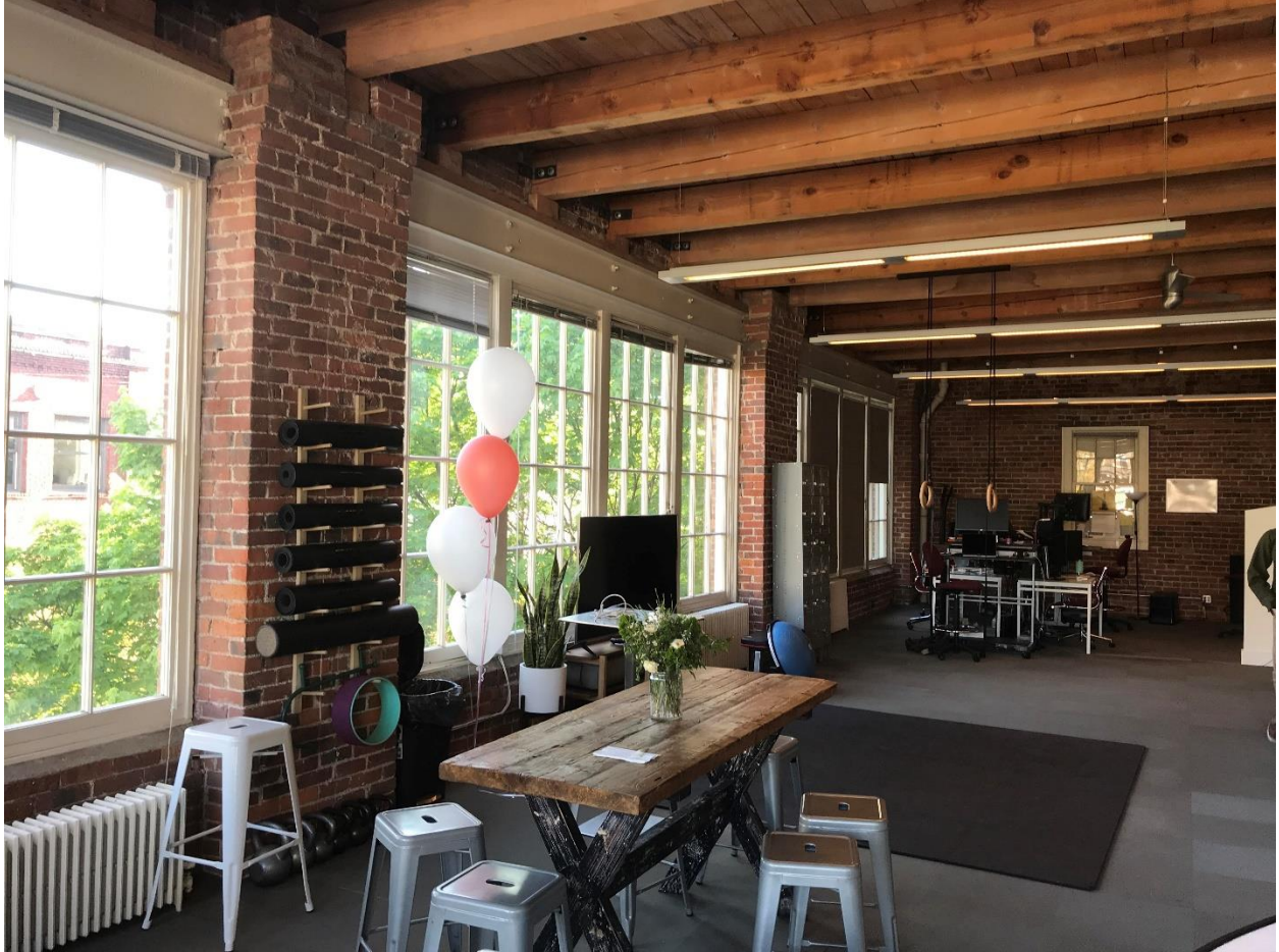
Figure 30) Photograph of exposed brick masonry exterior walls at north end of third floor level open office space.
