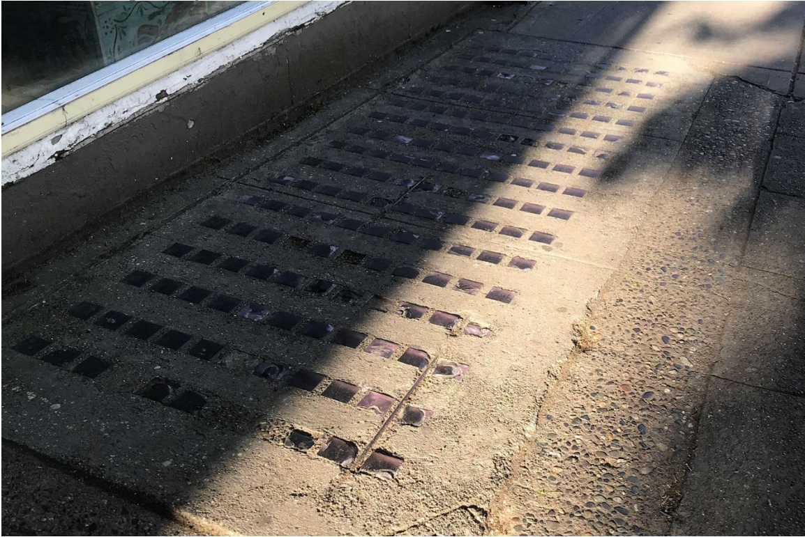
Figure 8) Sidewalk prism lights at areaway.
