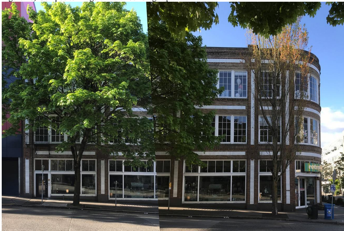
Figure 10) Composite image of north building façade.
