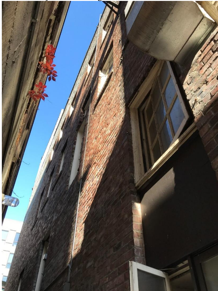
Figure 15) Partial view of south façade of building.
