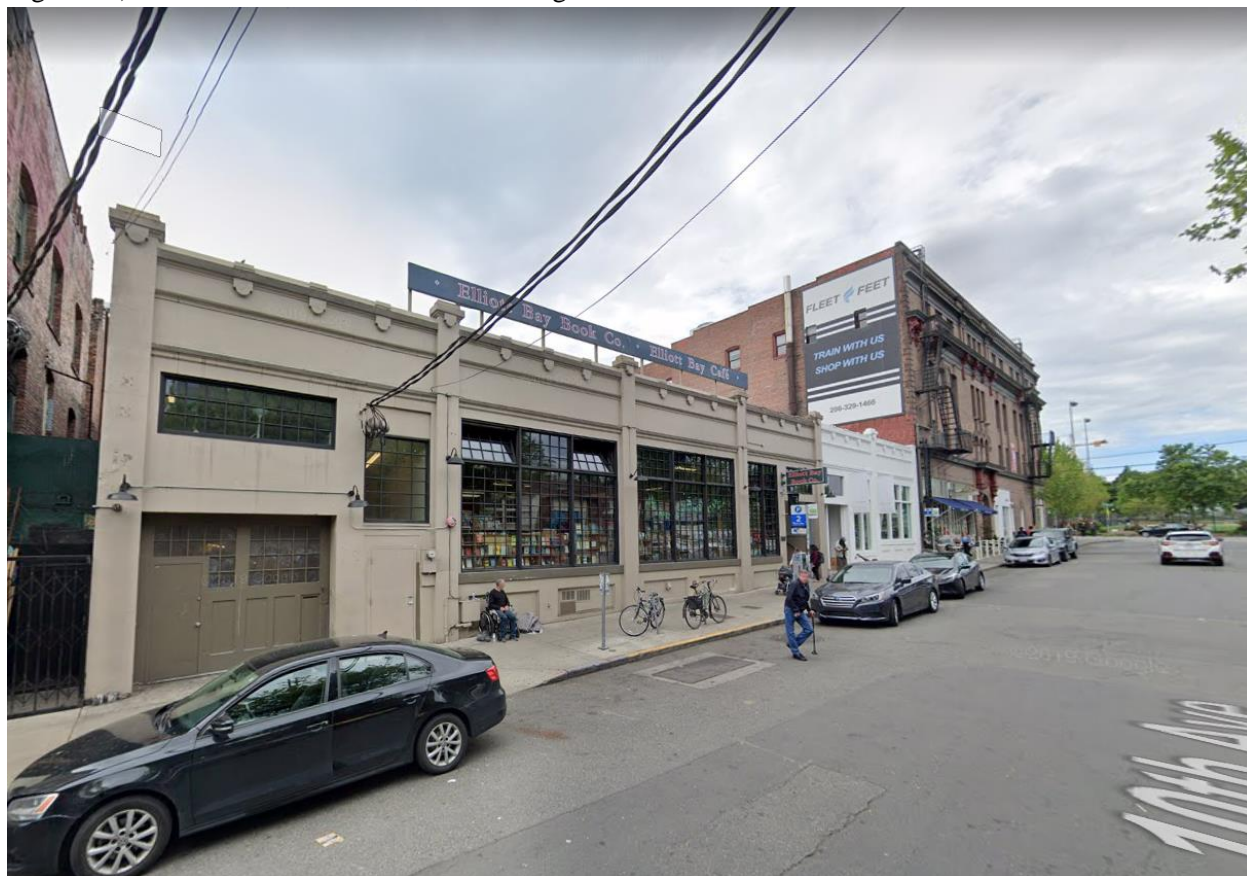
Figure 99) 1517-1521 10 th Avenue, 2019. Google.
