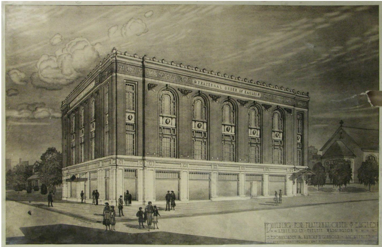
Figure 63) Everett Aerie of Eagles Project, 1921. NAHA P659, 1.4.
