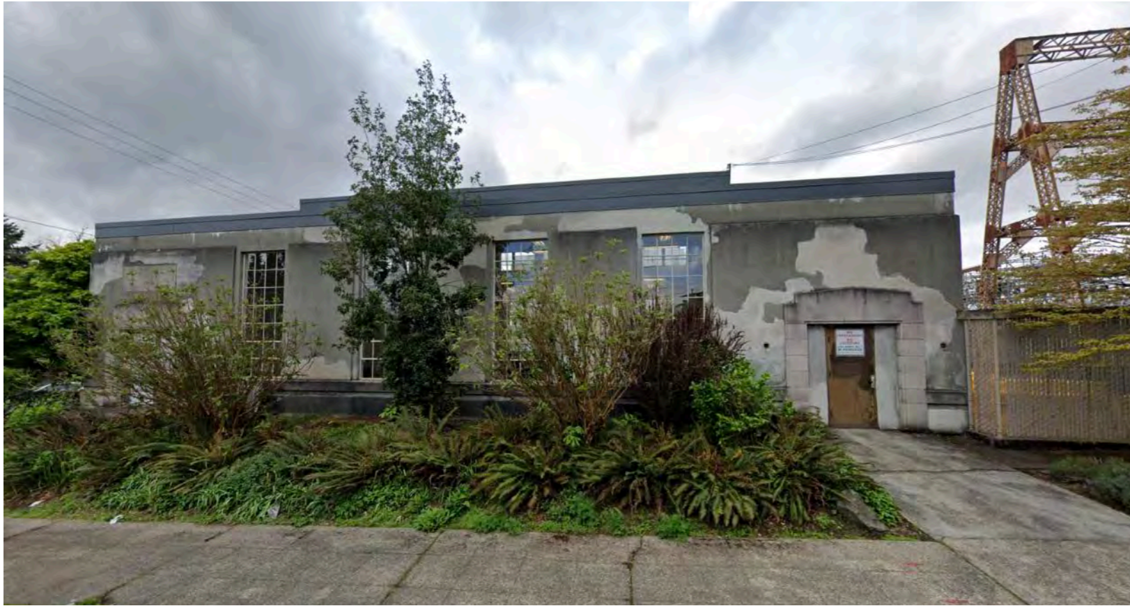
North Distribution Substation/North Substation Machine Shop 814 NE 75th Street NE, 1930
