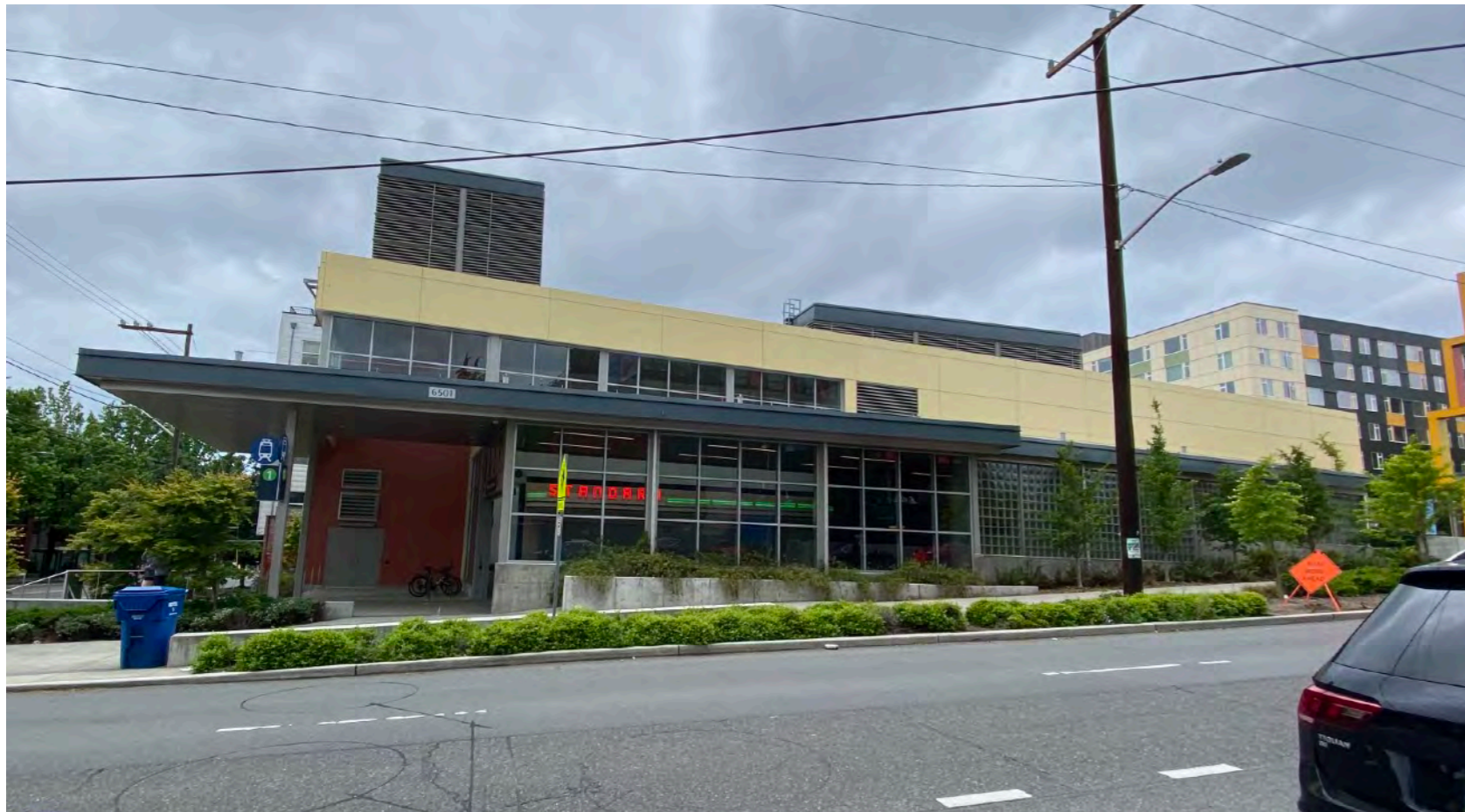
Standard Radio façade at Roosevelt light rail station
