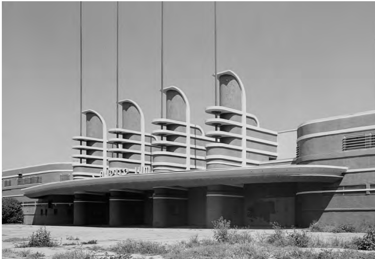
Pan-Pacific Auditorium, Los Angeles (1935, Welton & Becket, former National Register, demolished)
