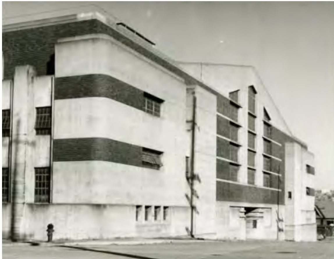
Armory Building, 1939, Naramore & Young
