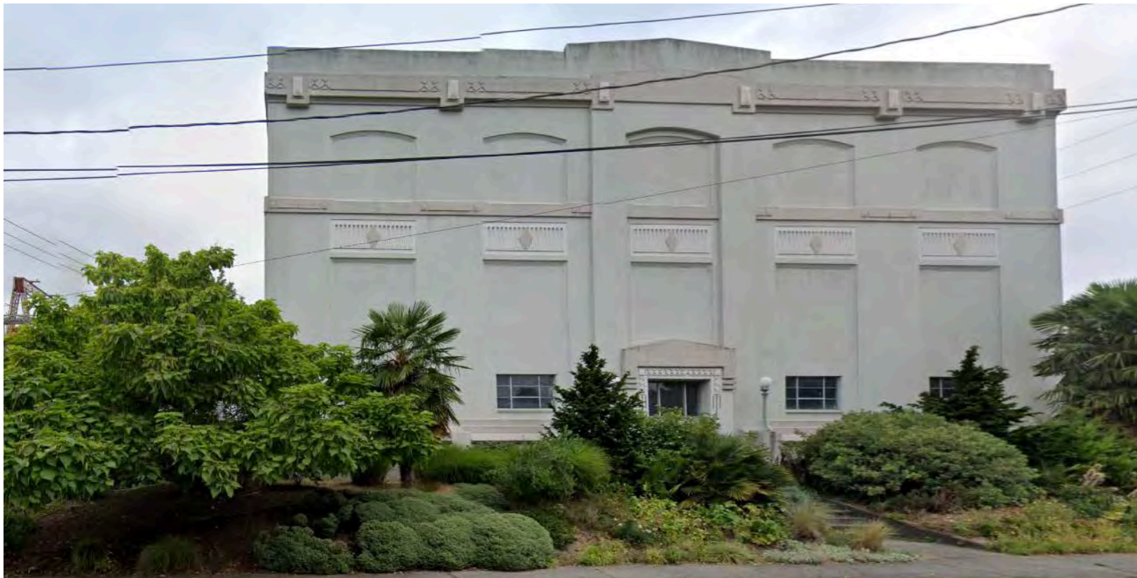
North Rectifier Substation 814 NE 75th Street NE, 1954
