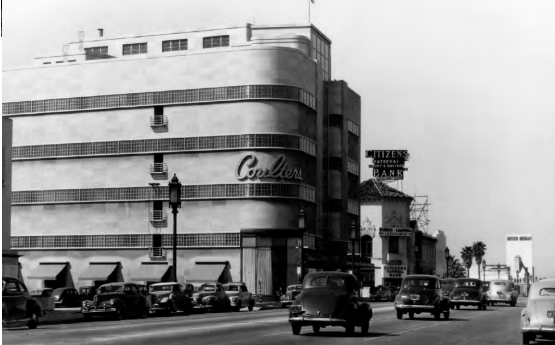
Coulter's Department Store, Los Angeles (1938-39, Stiles O. Clements, demolished)
