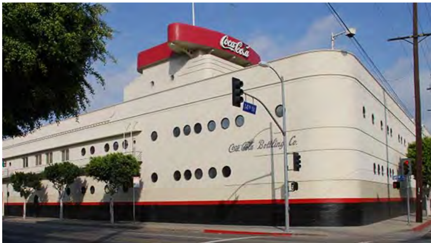
Coca-Cola Bottling Plant, Los Angeles (1939, Robert V. Derrah, National Register)
