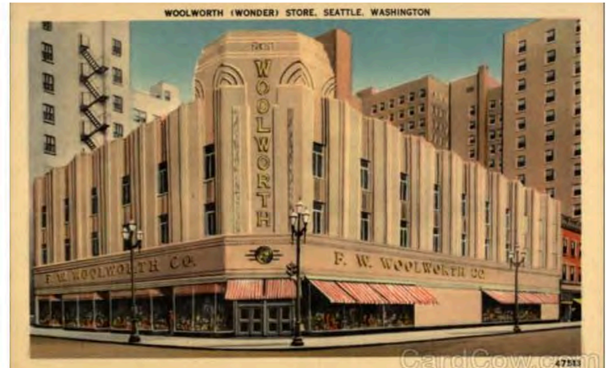
F.W. Woolworth Company Store, now Ross 301 Pike Street 1935, Harold B. Hillman, extant
