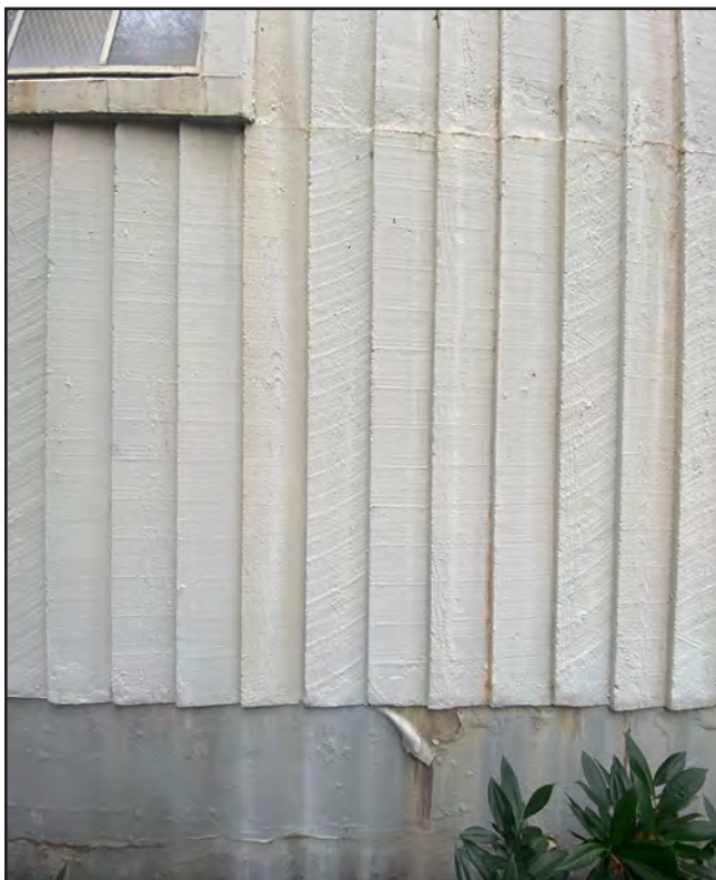
Figure 27 • Details of concrete finish at courtyard and main entry
