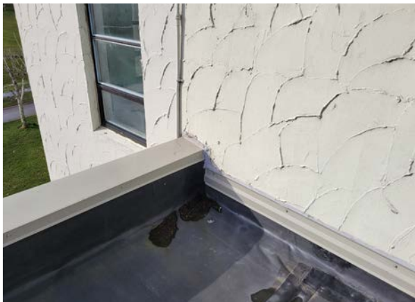
Photo 24 - Parapet saddle tied into concrete
