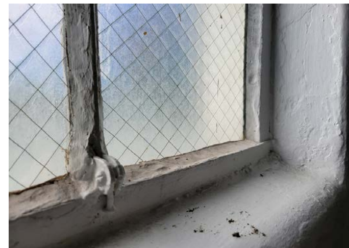
Photo 20 - Steel framed window with single pane wired glass
