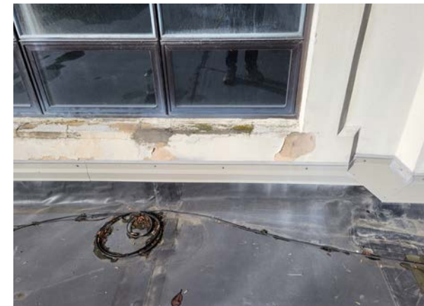
Photo 26 - Low flashing heights at windows
