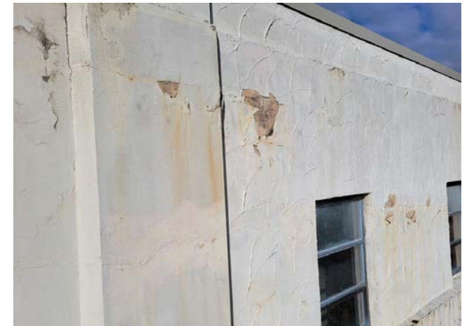
Photo 13 - Concrete cracks and peeling paint
