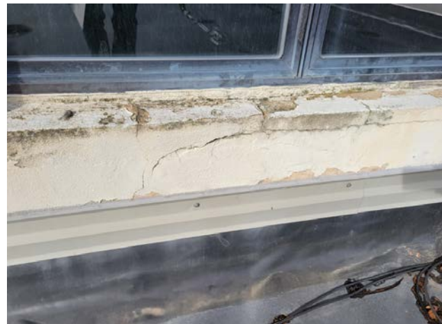
Photo 12 - Concrete cracks
