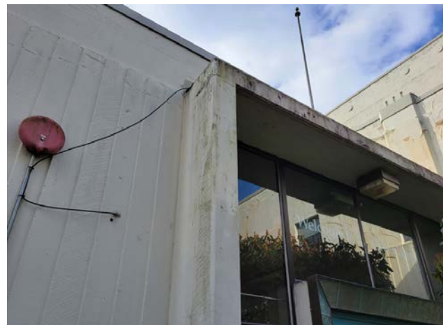
Photo 15 - Stained concrete at window head
