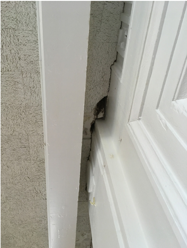
Image 3: View of separation between field house and pool addition caused by 2001 Nisqually Earthquake. A properly detailed seismic joint is recommended at this location.
