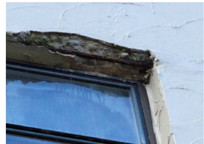
Photo 16 - Concrete spall at window head
