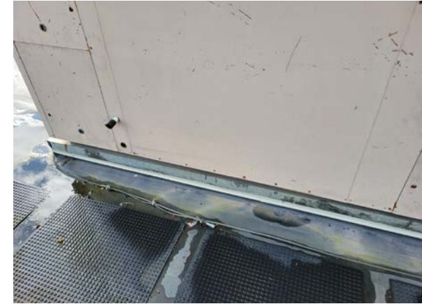
Photo 23 - Low roof curb at equipment
