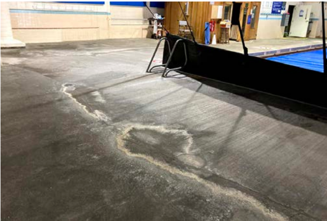
Image 2: View of cracking and spalling at pool deck
