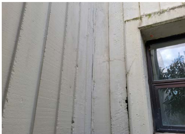
Photo 14 - Failed sealant
