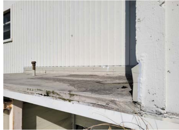
Photo 22 - PMMA waterproofing at concrete canopy
