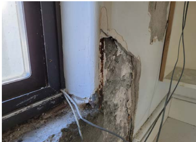
Photo 11 - Uninsulated concrete interior
