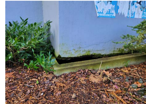
Photo 9 - View of settlement at building base
