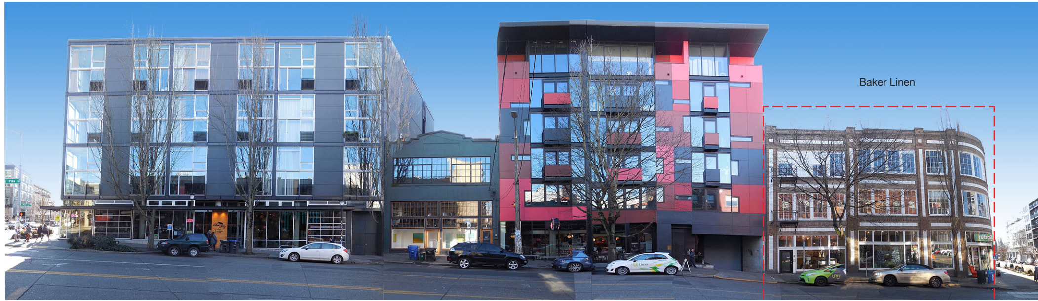
North elevation of the Baker Linen Building as seen from E Pike Street looking south
