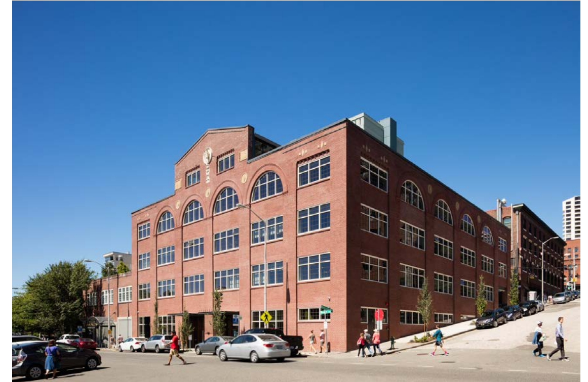
Union Stables, 2414 Western Avenue, Seattle ©Lara Swimmer
