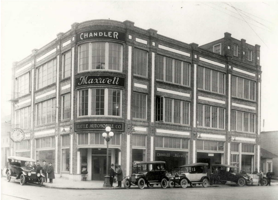
SE view of Baker Linen as seen from E Pike Street, 1916 (Courtesy of Paul Steiner Kilpatrick).
