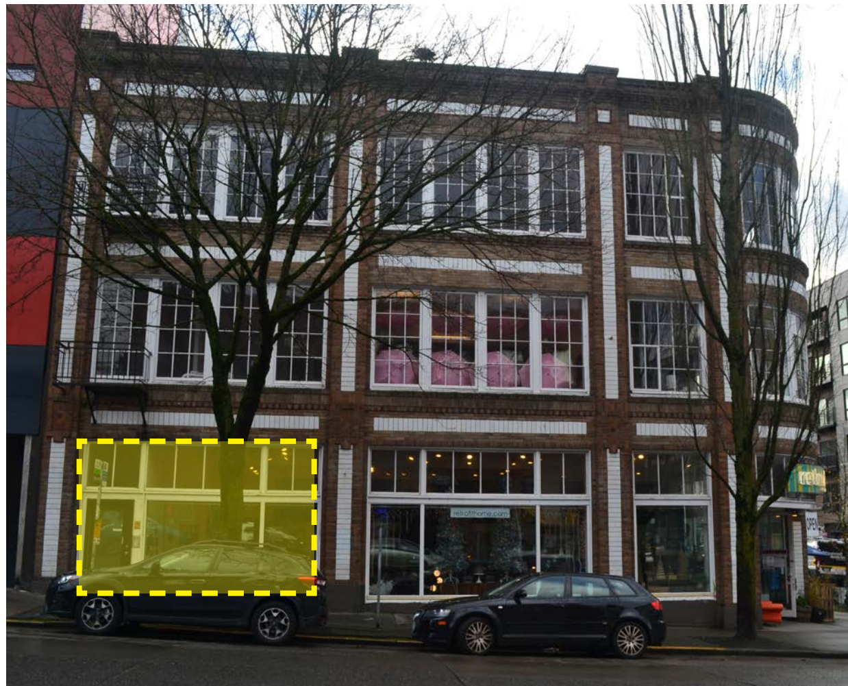
Current Condition - North Elevation
