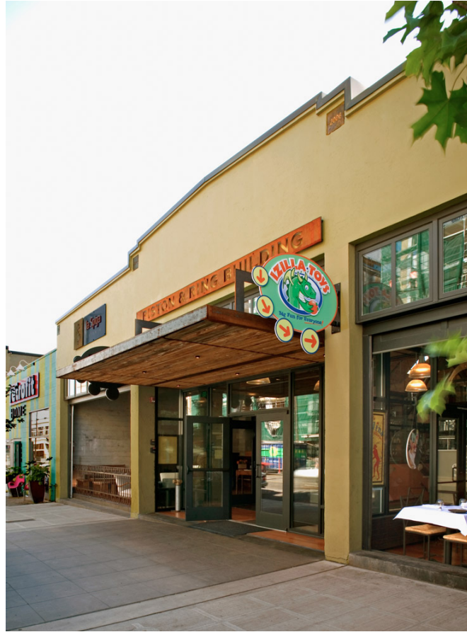
Piston & Ring Building, 1429 12th Ave., Seattle ©Michael Burns
