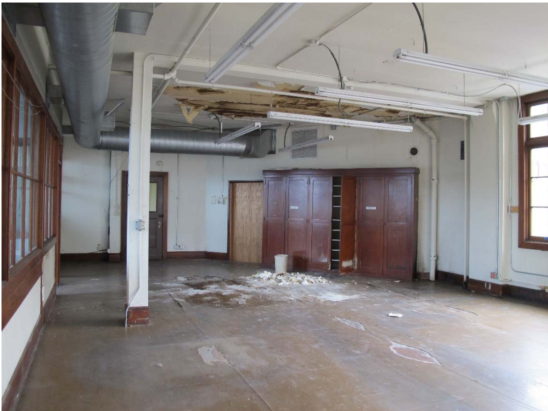
Fig. 113 – Interior, second floor, south offices
