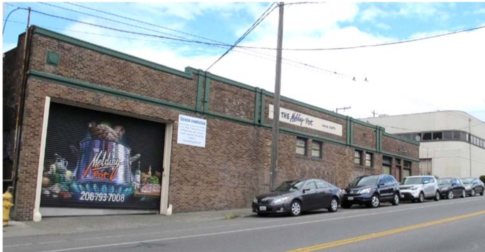
Fig. 49 – Field Roast Grain Meat Company (1925), at 1432 South Jackson Street. It may have originally been constructed as the San Gennaro Foods Company, later operated as a milk depot.
