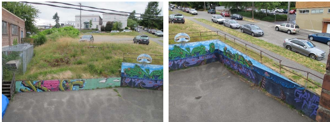
Fig. 80 – Parking area at rear of building
