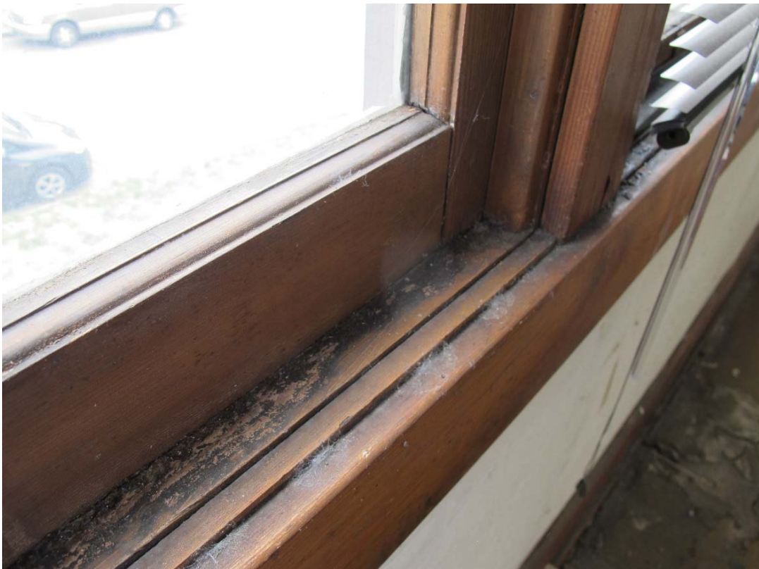
Fig. 115 – Interior, second floor, south wing room, detail of window interior
