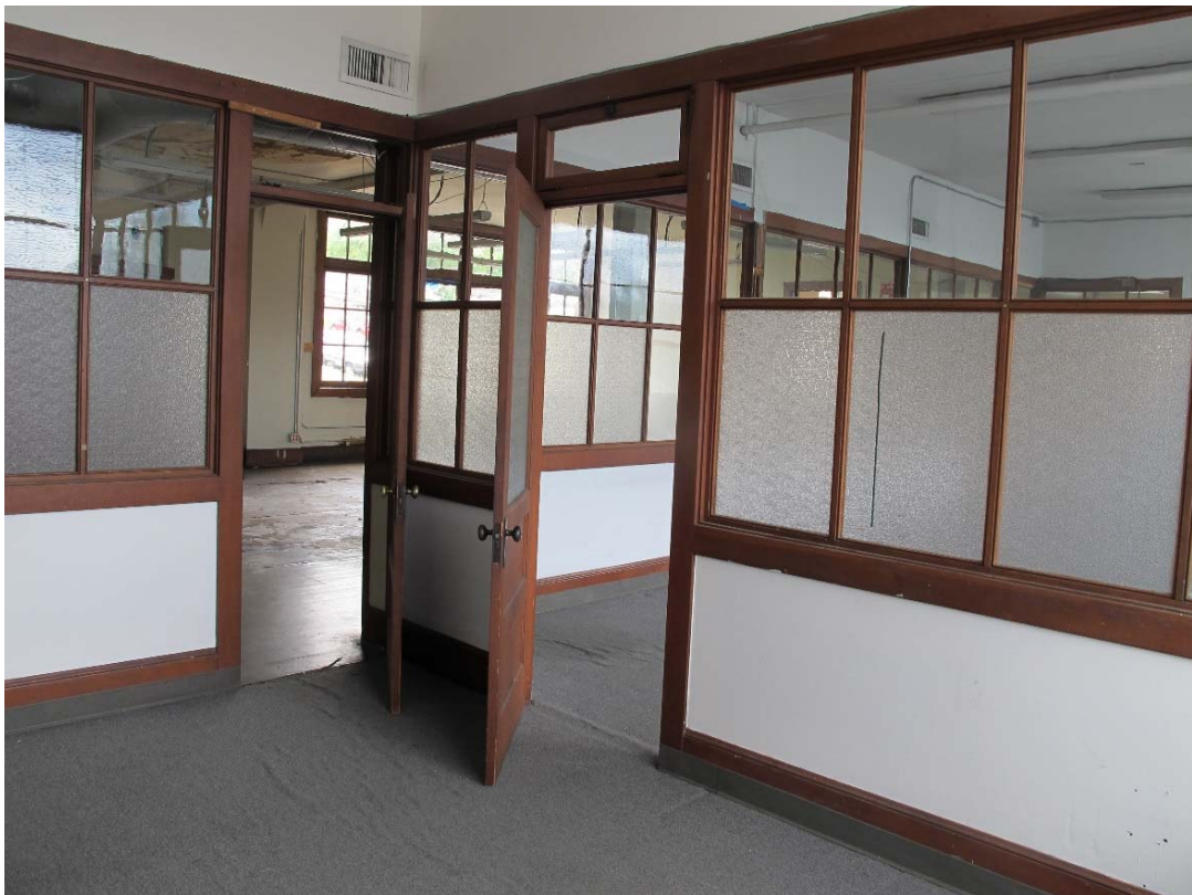
Fig. 107 – Interior, second floor, south offices
