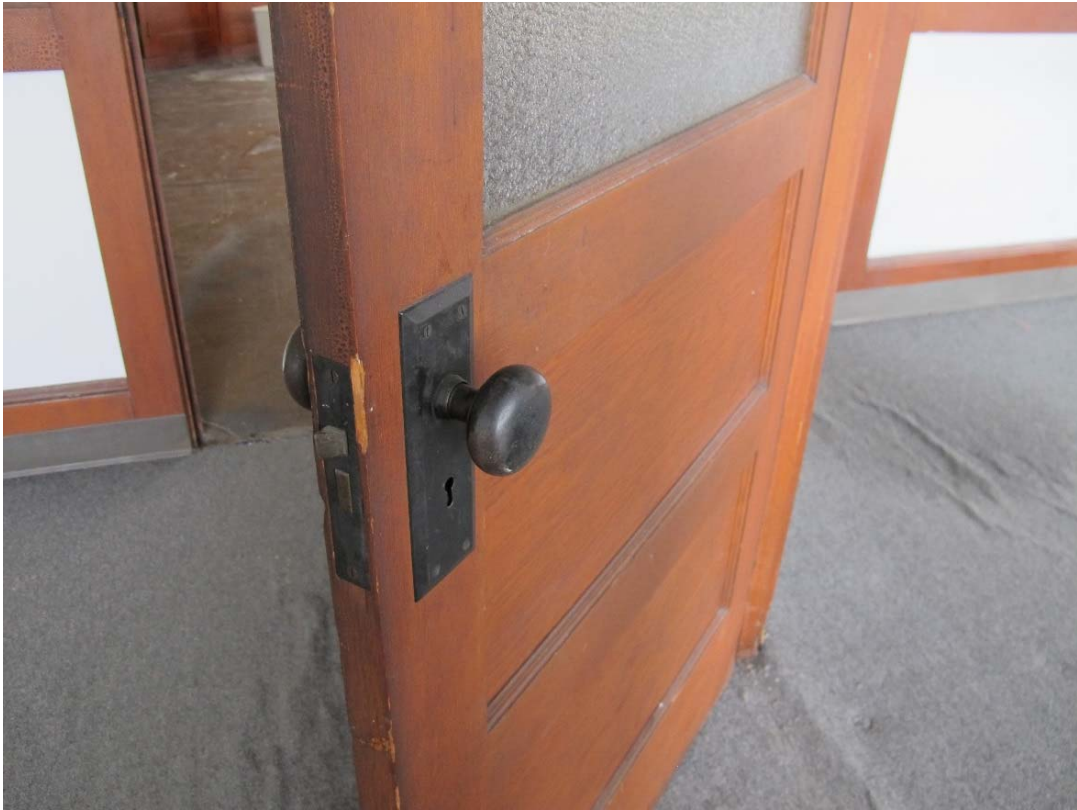
Fig. 118 – Interior, second floor, south offices, detail of door
