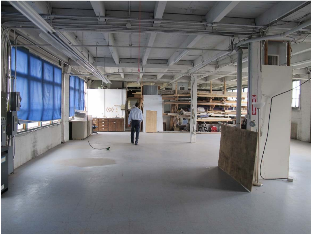
Fig. 102 – Interior, second floor, north part
