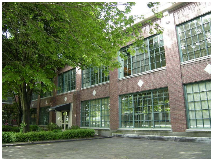
Fig. 46 – (Two images above) Black Bear Manufacturing Company building (1914, Andrew Willatzen), three blocks south of the subject site at 1130 Rainier Avenue South. The exterior is heavily obscured by trees. The building is a designated Seattle landmark.
