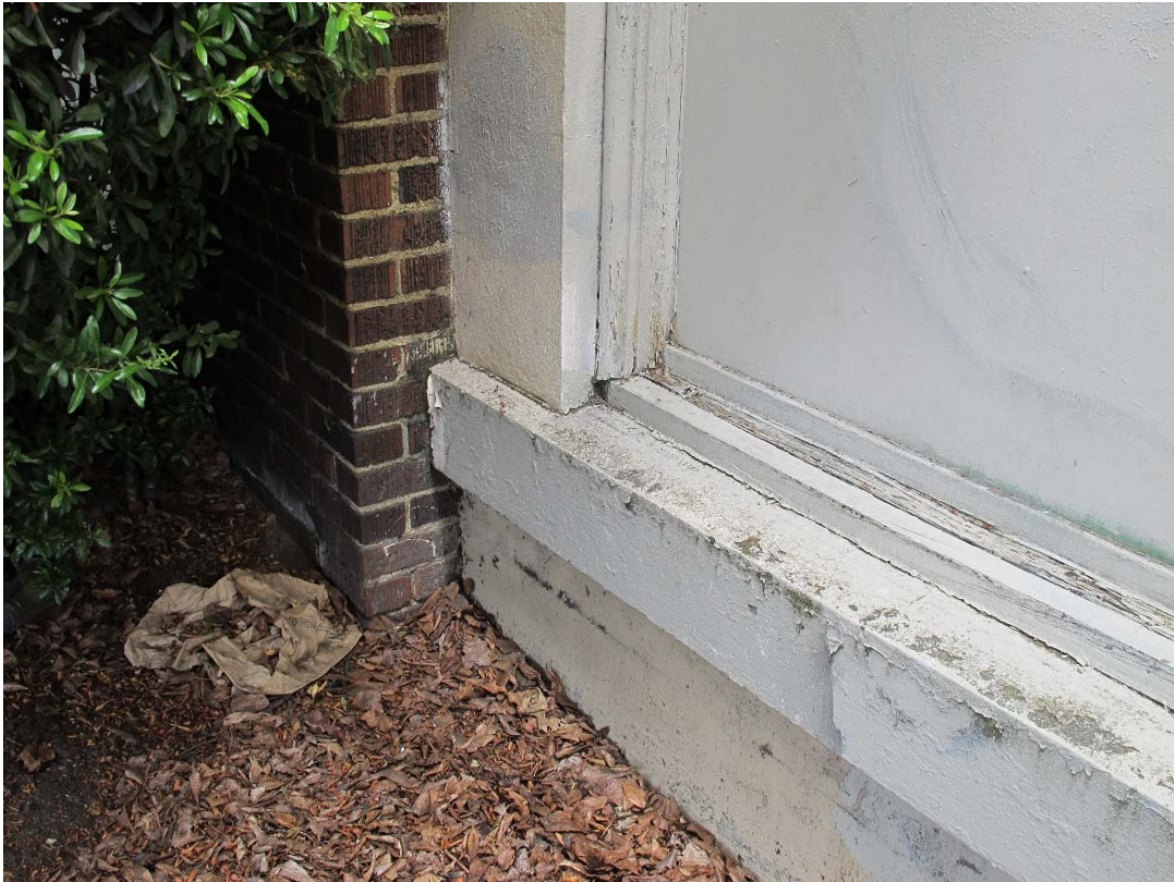
Fig. 66 – West elevation, detail of windows
