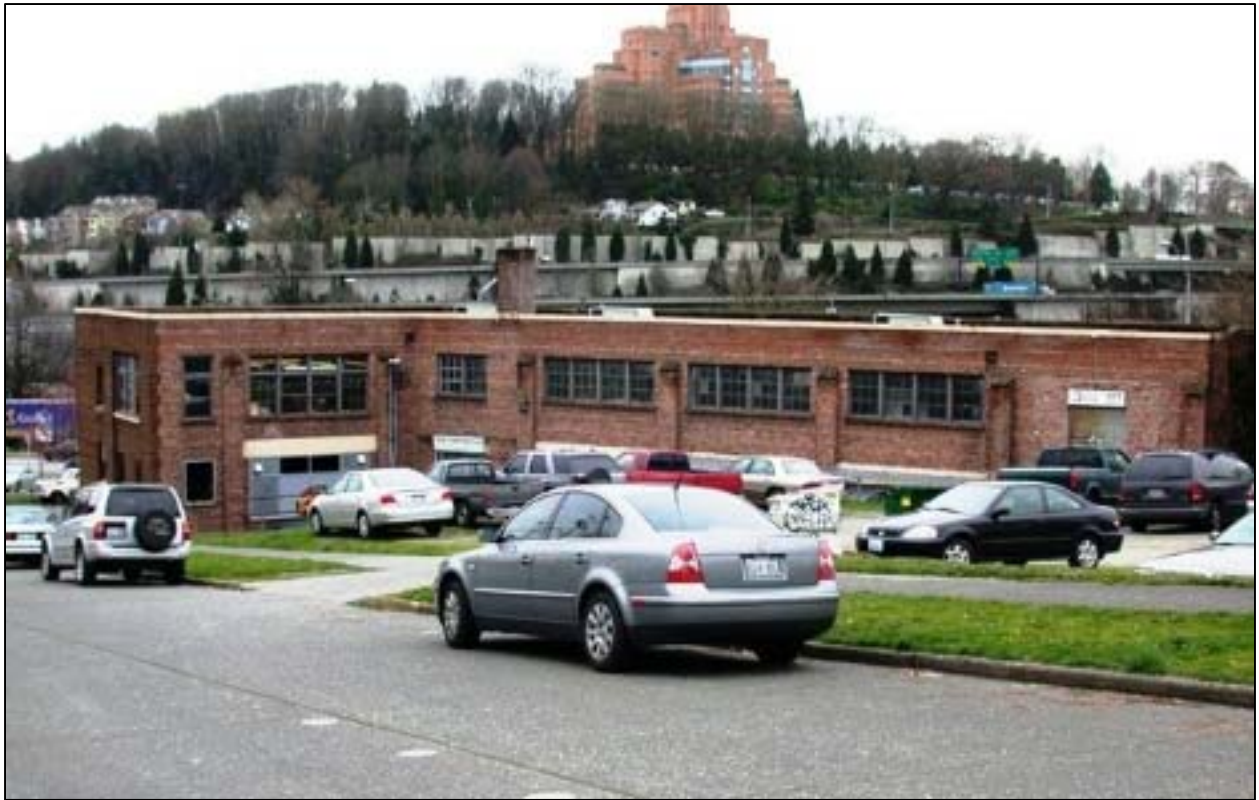
Fig. 55 – 2005 image of the rear of the building (DON)
