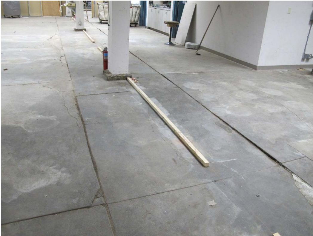
Fig. 100 – Interior, first floor, north wing, detail of floor with reinforced structure. Steel has been added under the floor in recent decades to support the weight of printing machinery.
