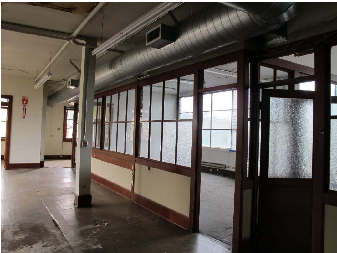
Fig. 111 – Interior, second floor, south offices
