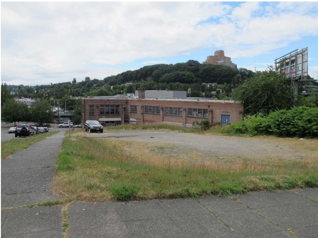
Fig. 87 – Rear of the building and eastern part of the parcel, viewed from uphill on 16 th Avenue South
