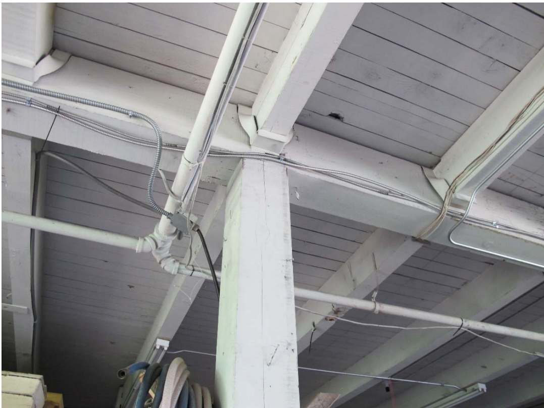
Fig. 103 – Interior, second floor, north part, detail of heavy timber structure
