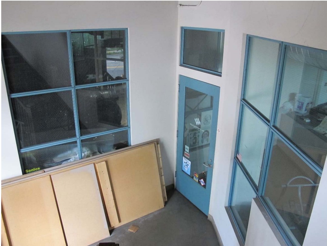
Fig. 94 – Interior, first floor, main entry foyer
