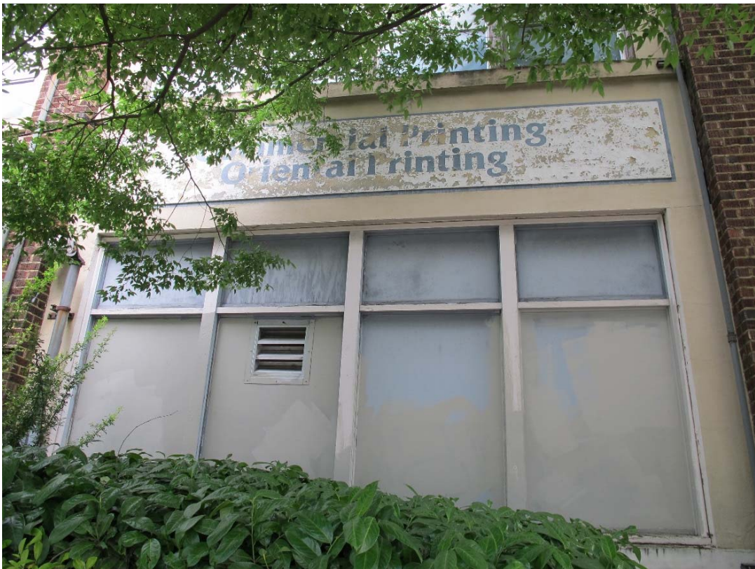
Fig. 67 – West elevation, detail of window with original frame
