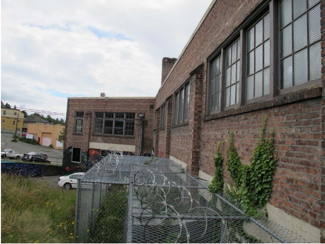
Fig. 78 – North rear elevation and east rear elevation
