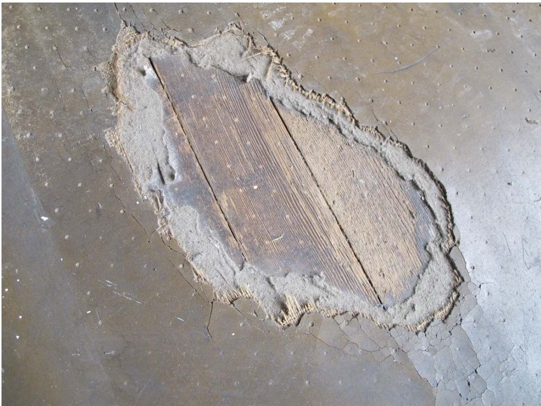
Fig. 117 – Interior, second floor, south offices, detail of linoleum floor
