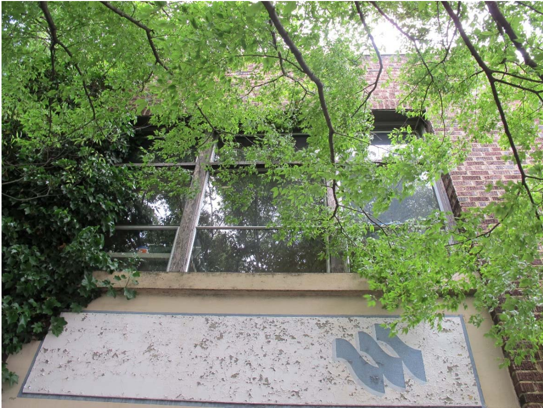
Fig. 68 – West elevation, detail of metal sash windows with original frame
