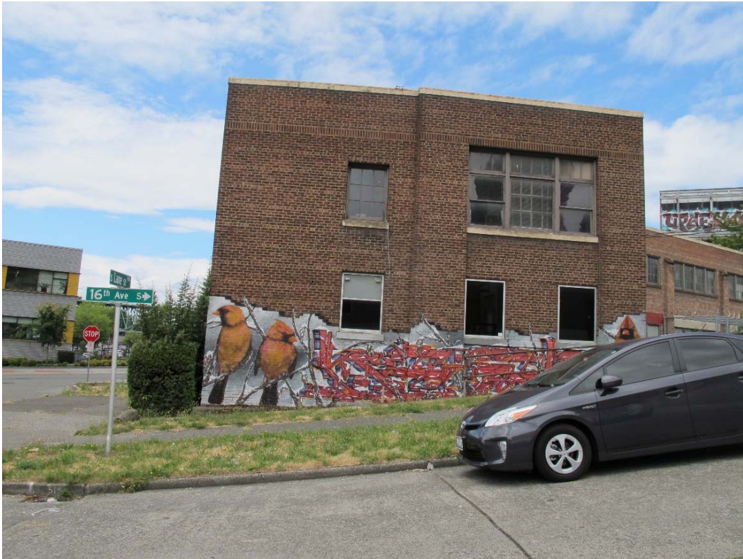
Fig. 76 – East elevation. First floor windows shown here are modern replacements following the 1992 fire.
