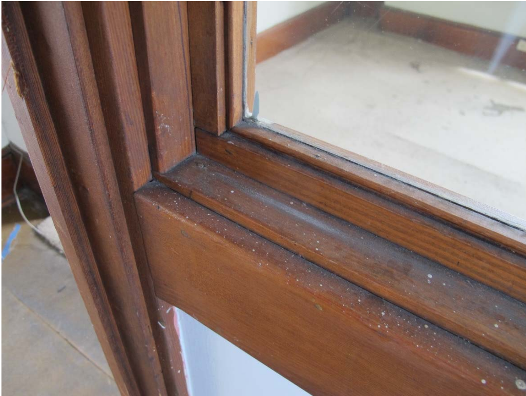
Fig. 114 – Interior, second floor, south offices, detail of interior glazed partitions
