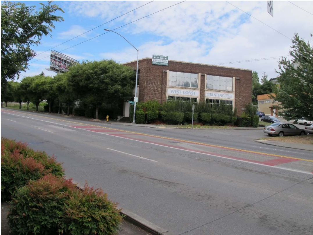
Fig. 74 – View of southwest building corner, looking north on Rainier Avenue
