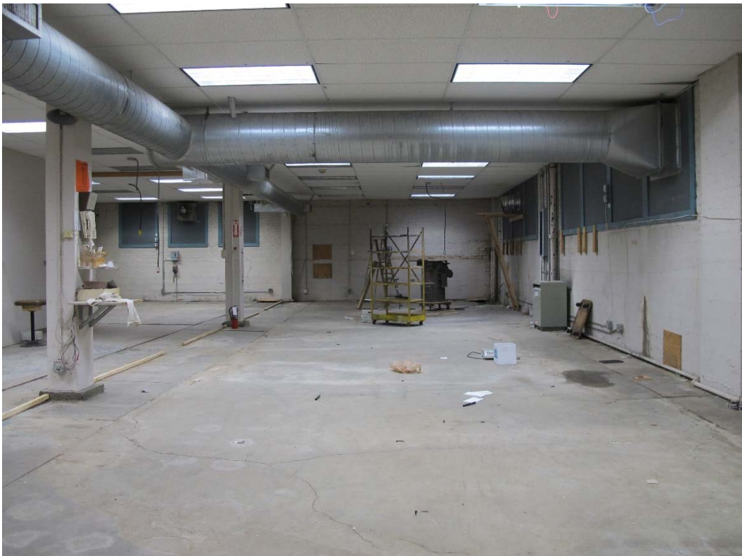
Fig. 99 – Interior, first floor, north wing
