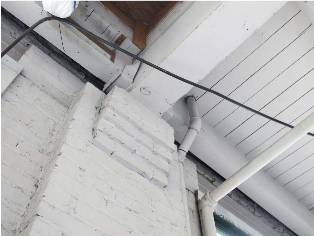
Fig. 104 – Interior, second floor, north part, detail of beam at corbelled wall pier connection
