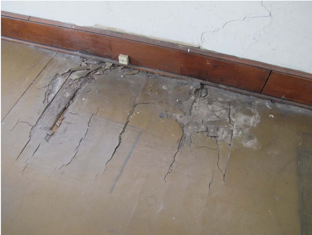
Fig. 116 – Interior, second floor, south offices, detail of linoleum floor
