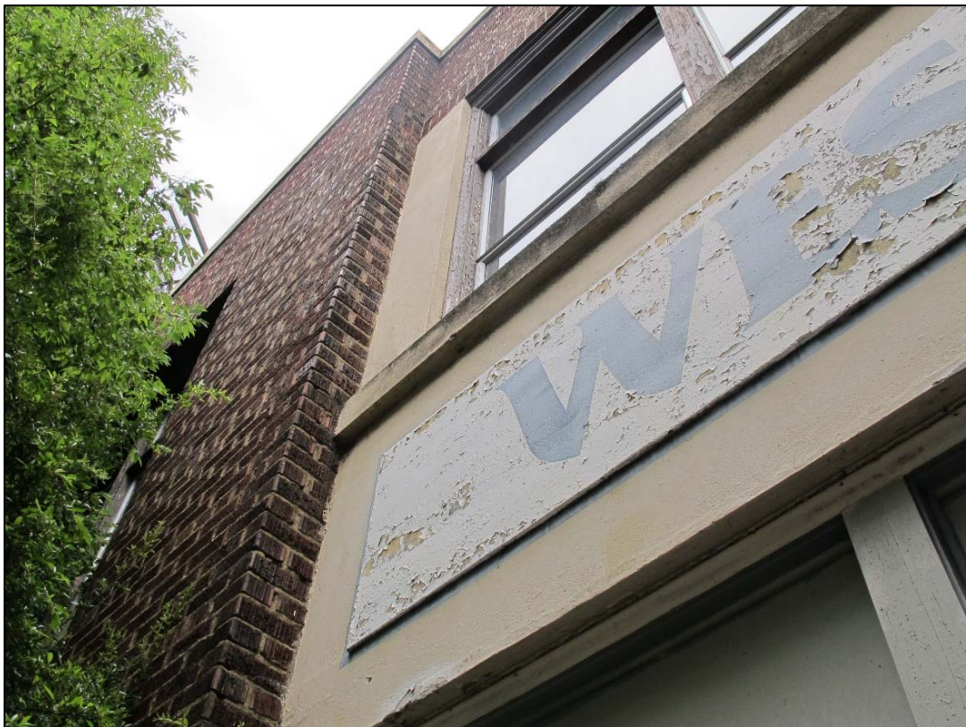
Fig. 65 – West elevation, detail of windows
