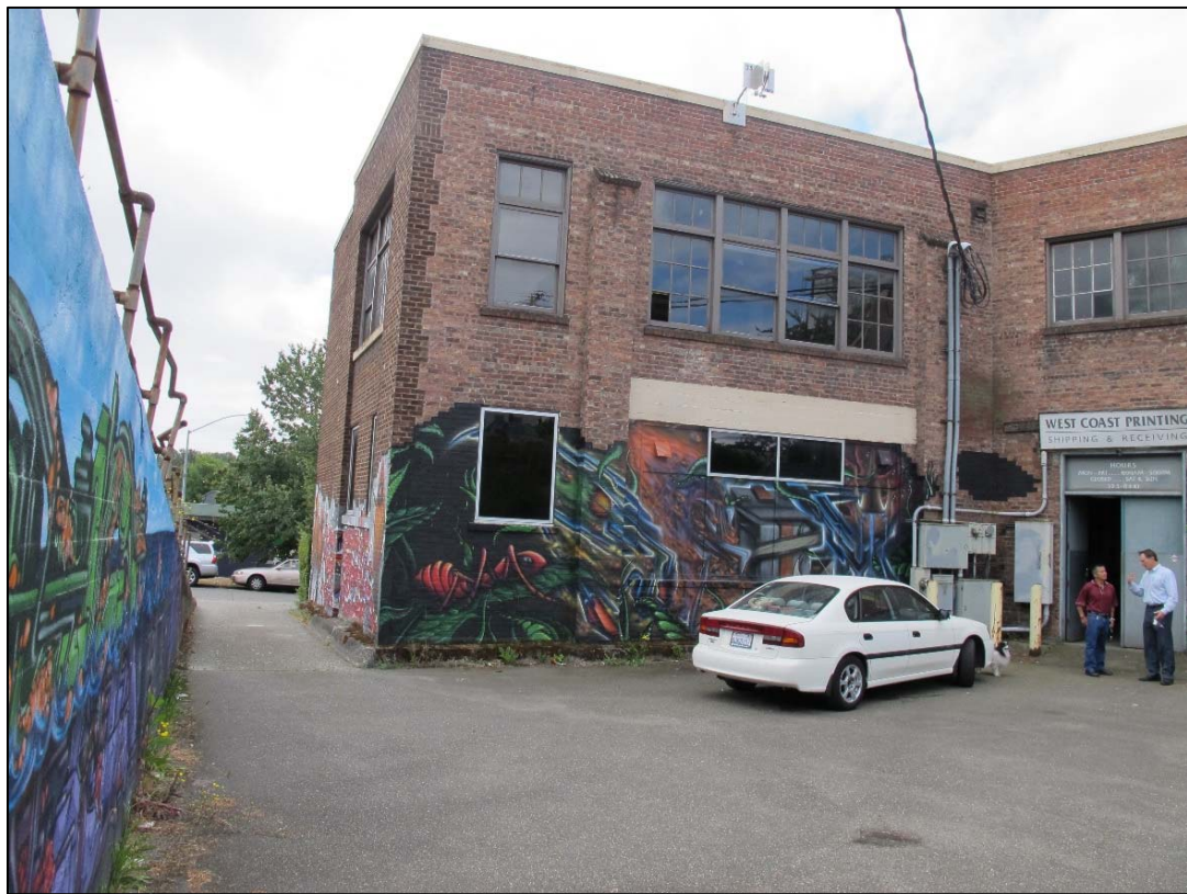
Fig. 81 – North rear elevation
