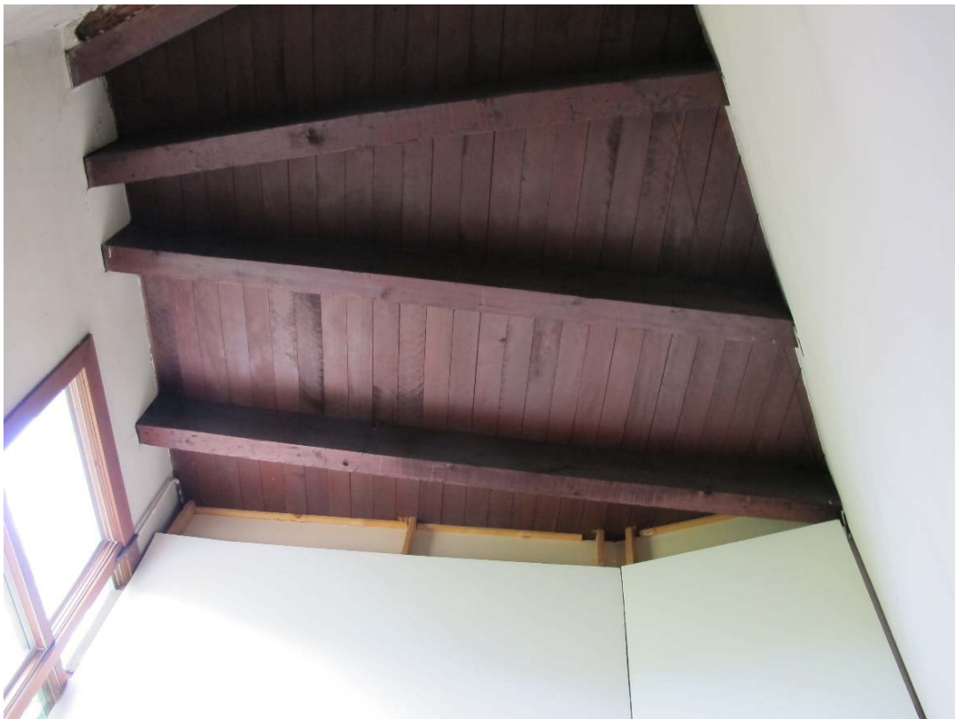
Fig. 91 – Interior, first floor, main entry foyer, view upwards to show detail of ceiling
