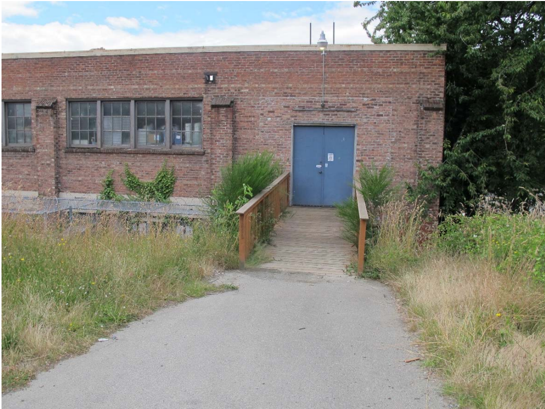
Fig. 84 – East rear elevation, upper floor, showing access door and ramp
