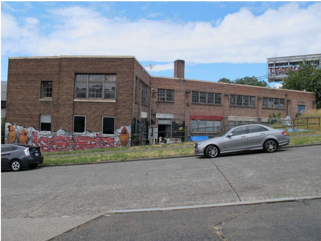
Fig. 77 – Rear of building viewed from the east
