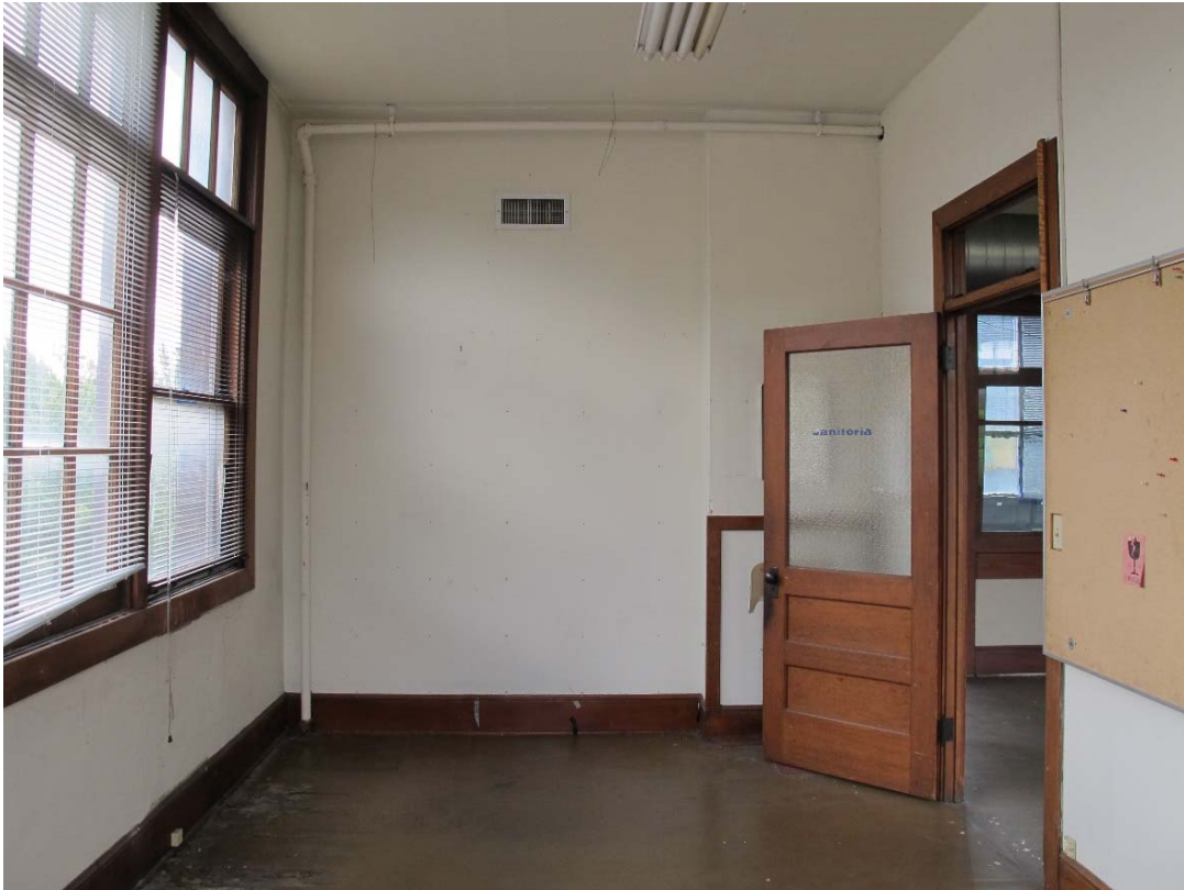
Fig. 122 – Interior, second floor, south wing room
