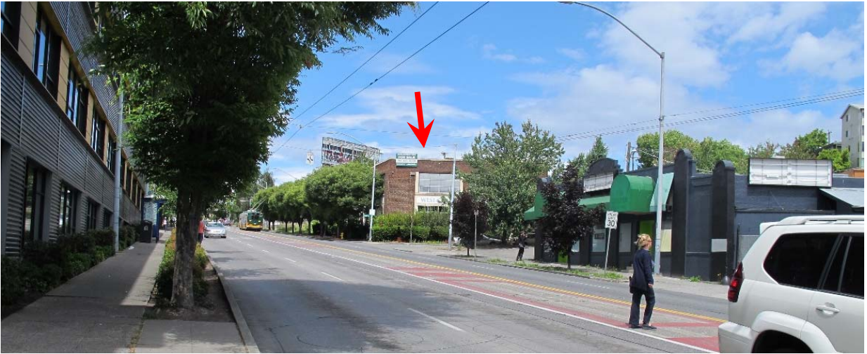
Fig. 57 – Context: View northward on Rainier Avenue. Arrow indicates subject building.
