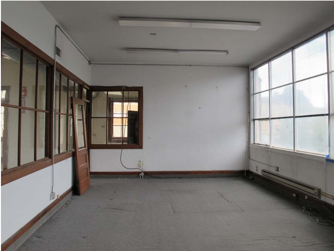
Fig. 108 – Interior, second floor, south offices
