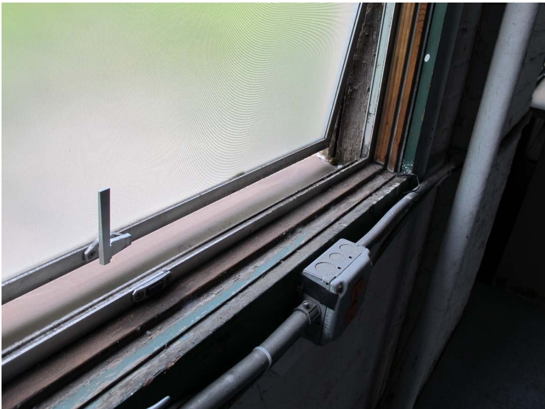
Fig. 69 – West elevation, detail of metal sash windows within original frame (interior)
