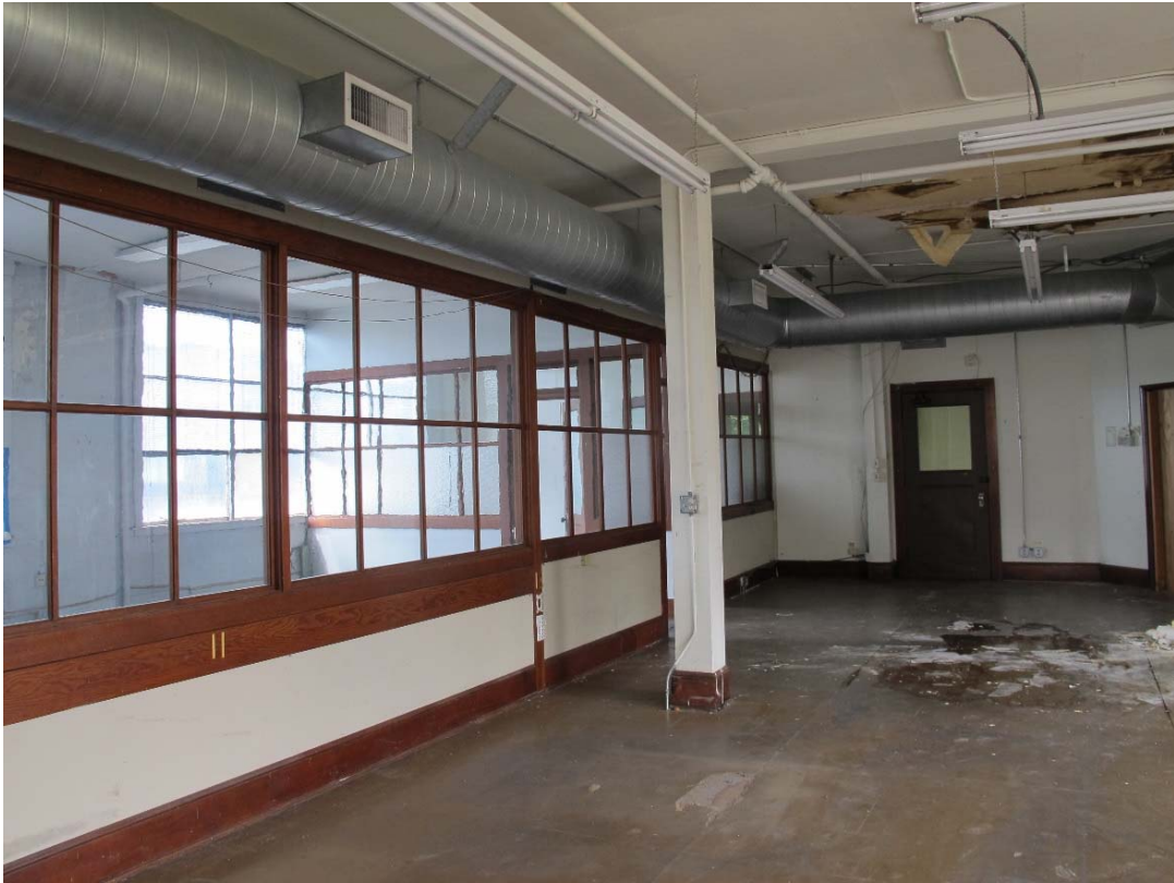
Fig. 112 – Interior, second floor, south offices
