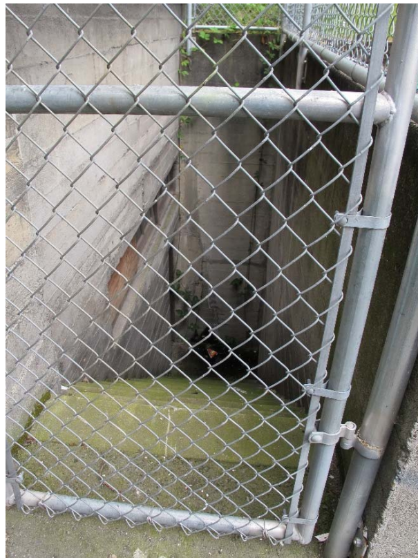
Fig. 85 – East rear elevation, showing access to basement level
