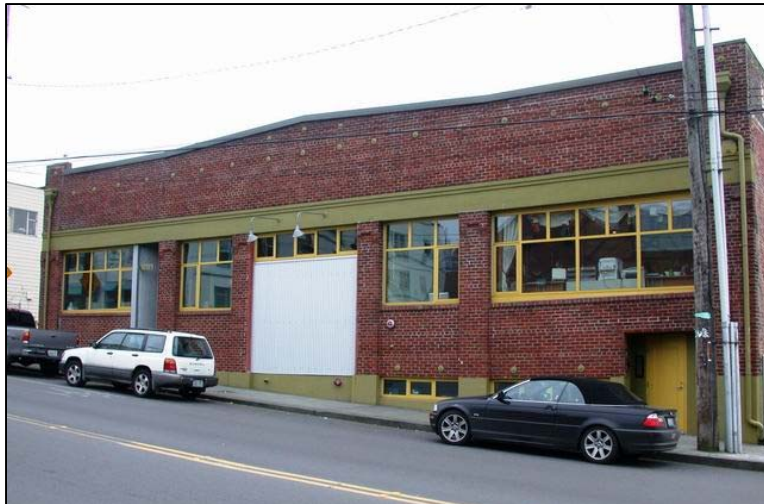
Fig. 48 – Rainier Electric Oven Manufacturing Company (1925), at 1419 South Jackson Street.
