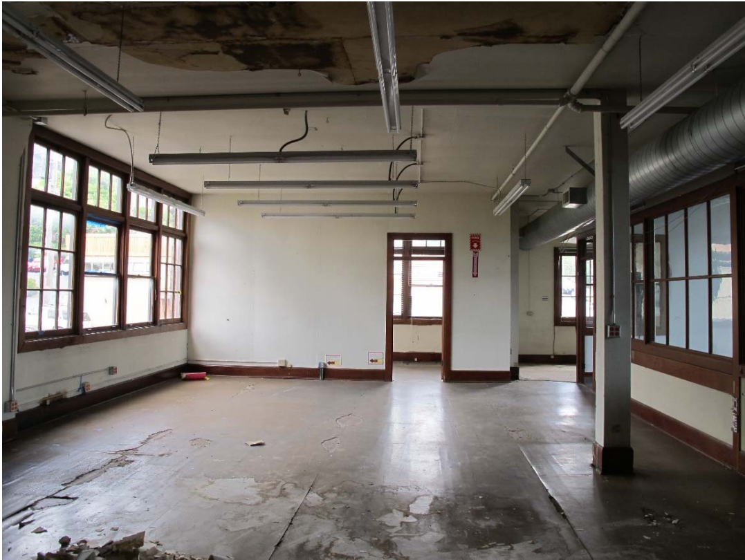
Fig. 110 – Interior, second floor, south offices
