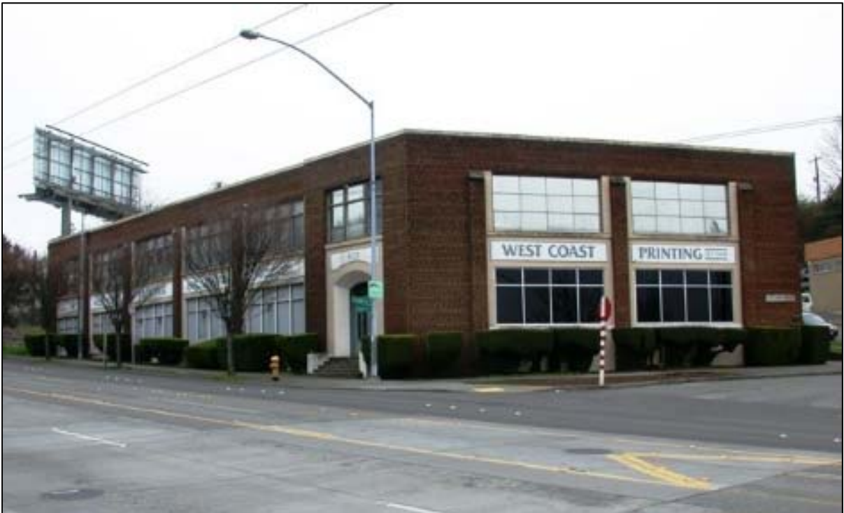
Fig. 54 – 2005 image of the west elevation, unobscured by trees (DON)
