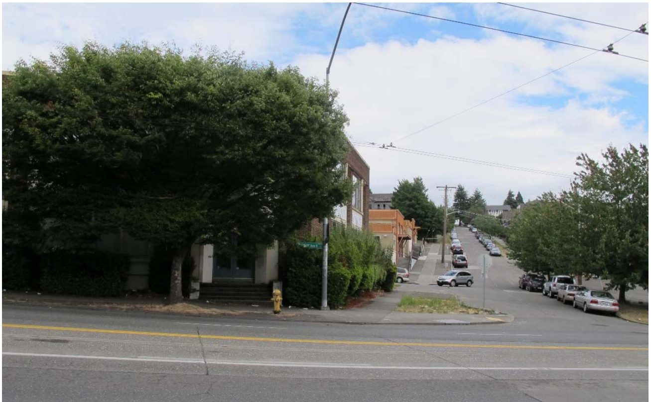
Fig. 73 – View of southwest building corner, looking east on Lane Street
