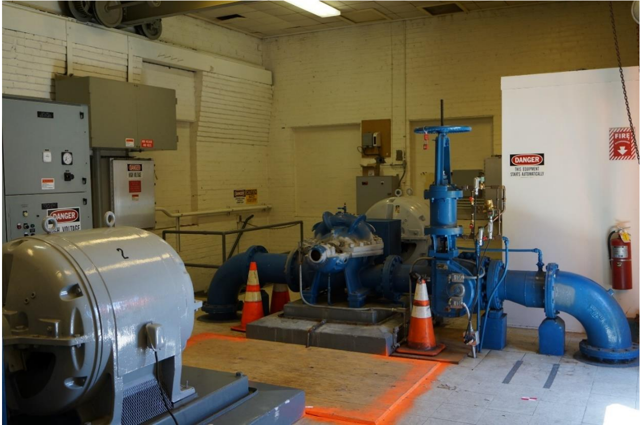
Photo 7. SW Spokane St. Pump Station, May 23, 2019, interior of the main floor, view east.
