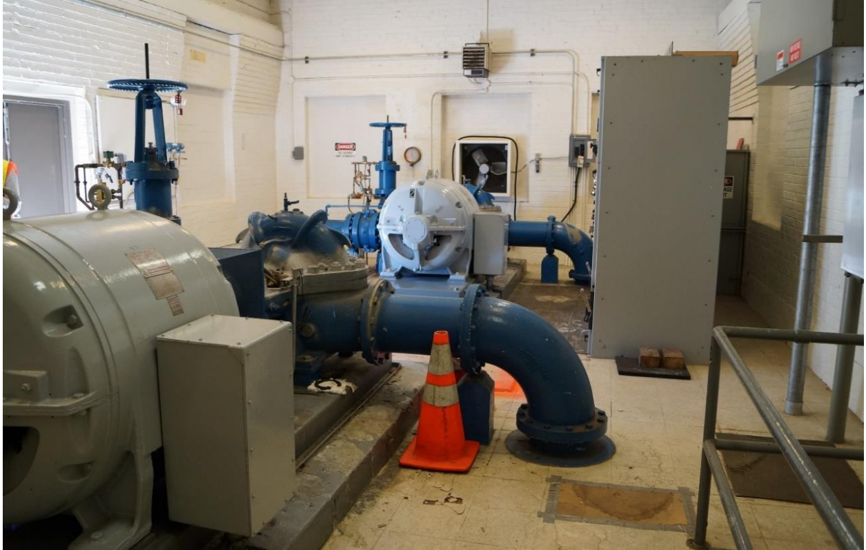
Photo 6. SW Spokane St. Pump Station, May 23, 2019, interior of the main floor, view west.
