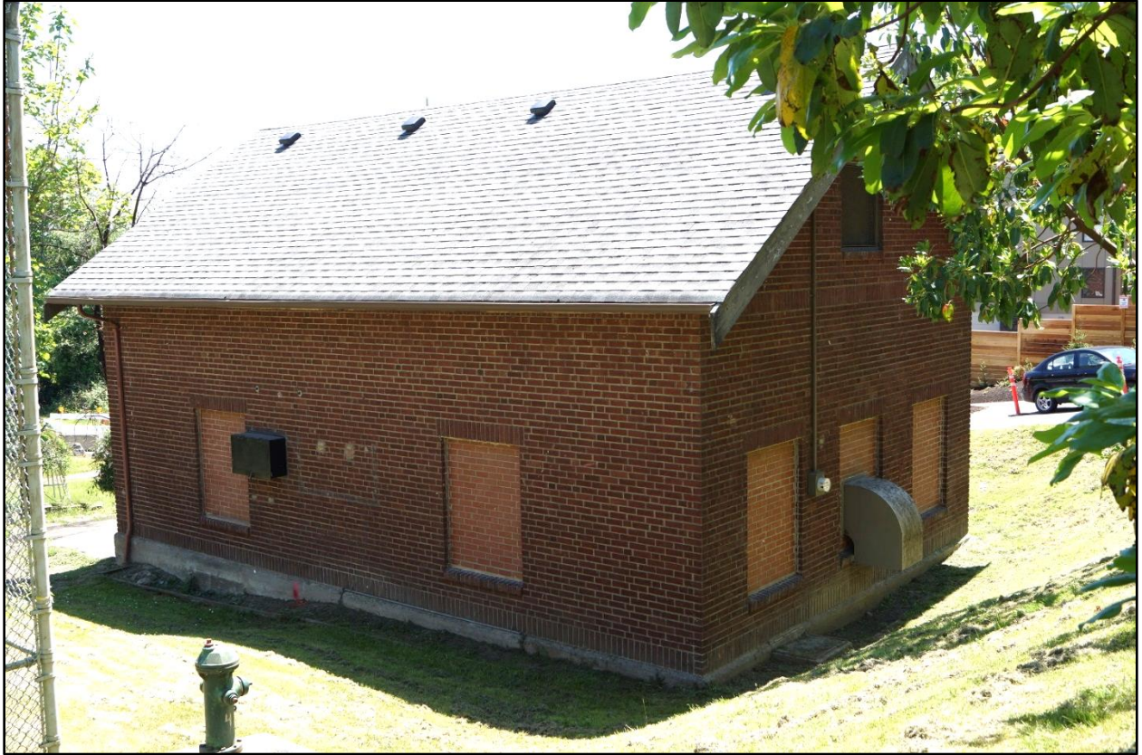
Photo 5. SW Spokane St. Pump Station, May 23, 2019, view southeast.
