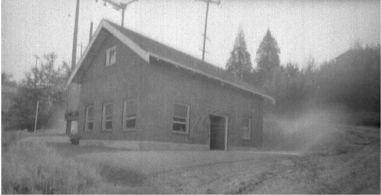
Figure 14. City of Seattle photo of the SW Spokane St. Pump Station, view northeast (May 8, 1931). Photo on file with Seattle Municipal Archives, Seattle.
