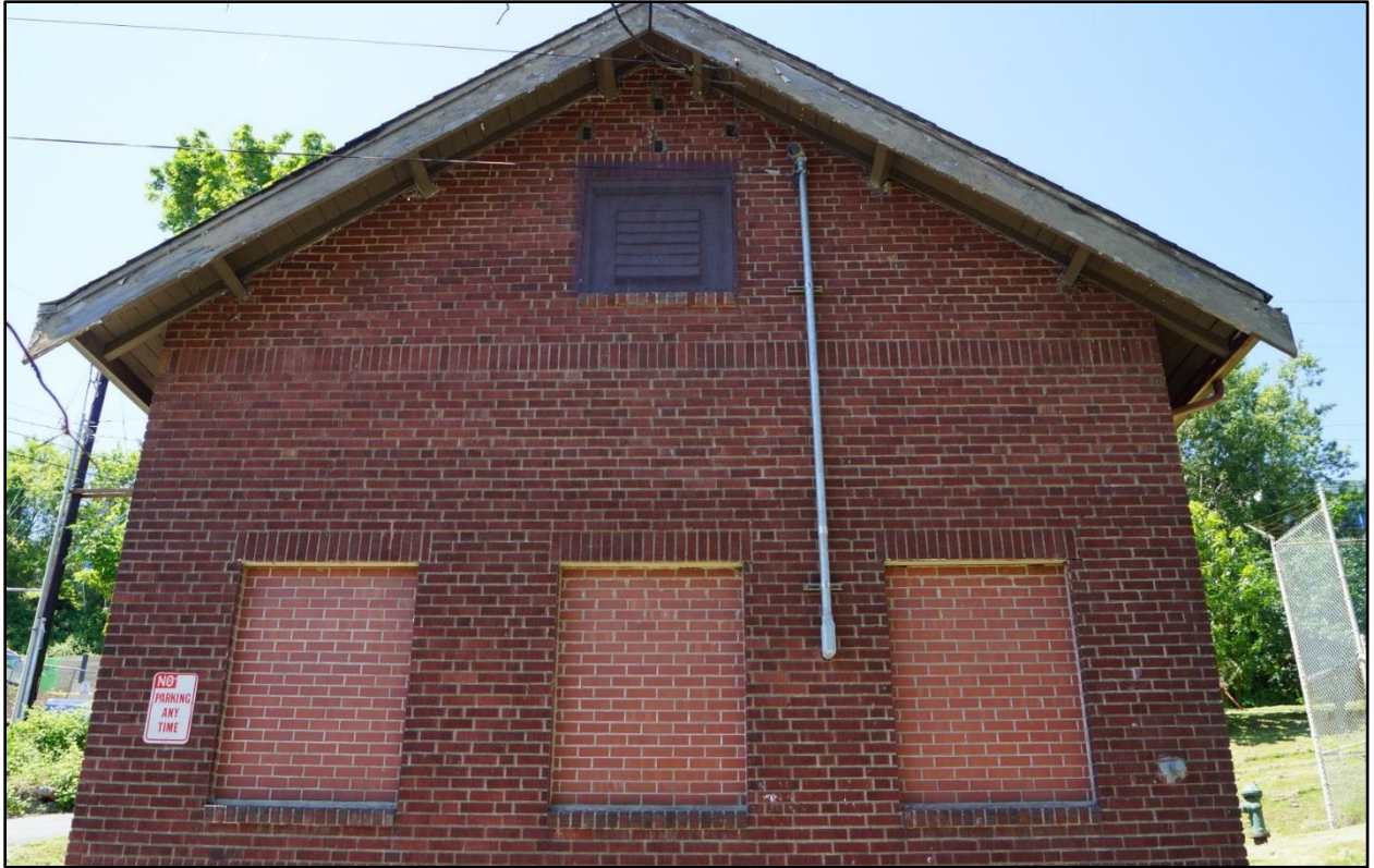
Photo 4. SW Spokane St. Pump Station, May 23, 2019, view west.
