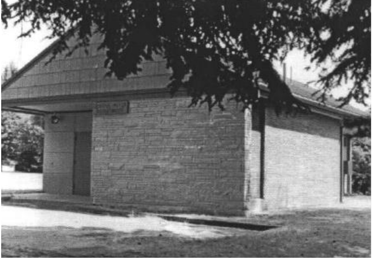
Figure 23. Examples of Seattle pump stations: Roosevelt Way Pump Station (photographed in 2000). Photo on file with the Washington State Department of Archaeology and Historic Preservation.
