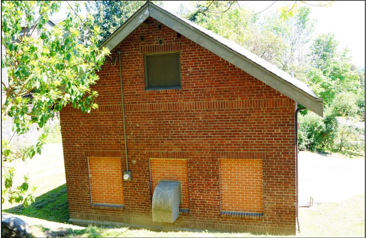
Photo 3. SW Spokane St. Pump Station, May 23, 2019, view east.
