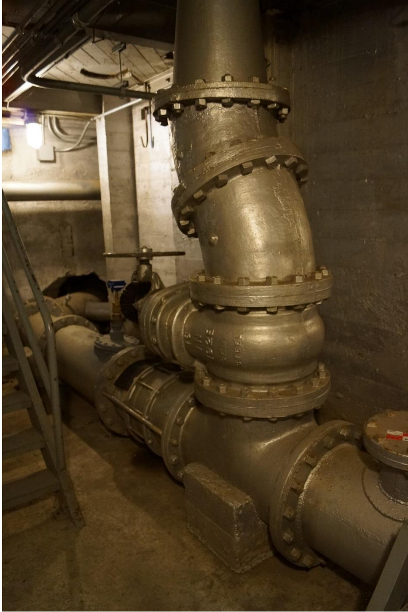
Photo 9. SW Spokane St. Pump Station, May 23, 2019, interior of basement floor, view east.
