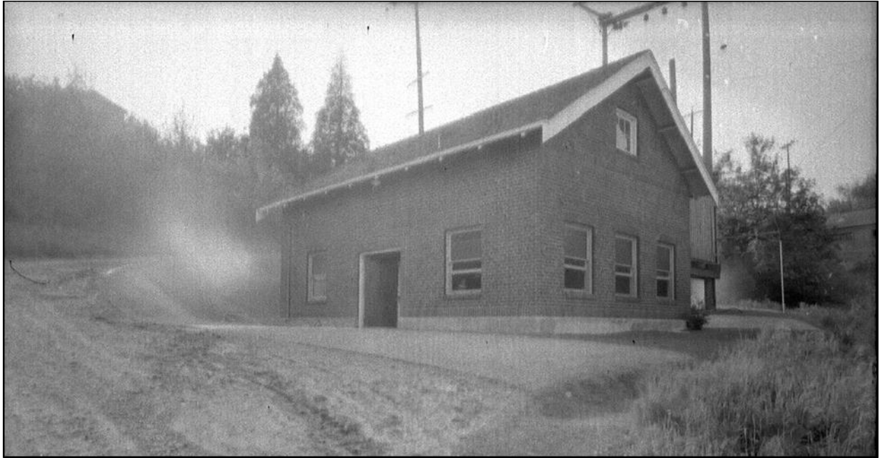
Figure 12. City of Seattle photo of the SW Spokane St. Pump Station, view northwest (May 8, 1931). Photo on file with Seattle Municipal Archives, Seattle.
