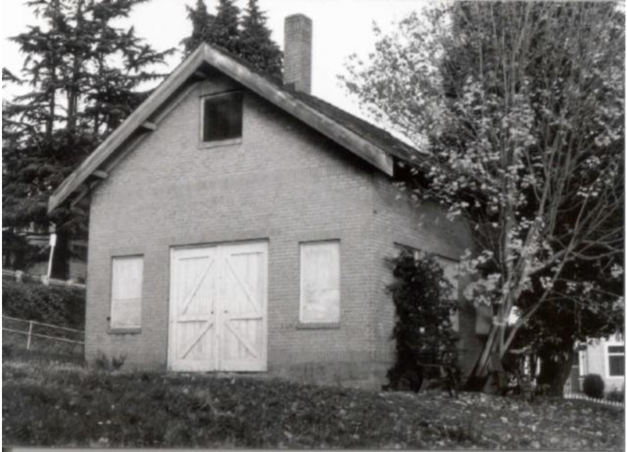
Figure 22. Examples of Seattle pump stations: Queen Anne Pump Station (photographed in 2000). Photo on file with the City of Seattle Department of Neighborhoods, Seattle.
