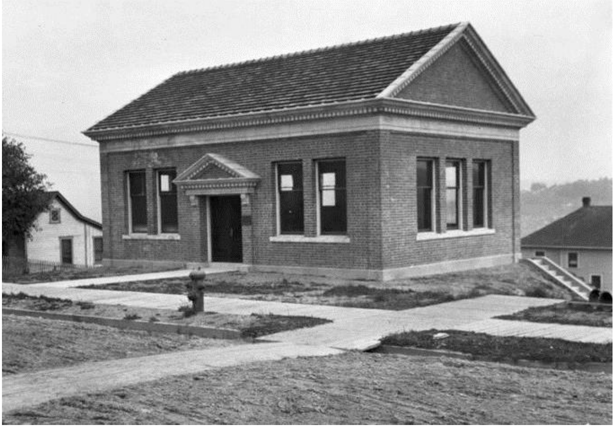
Figure 21. Examples of Seattle pump stations: Interbay Pump Station (photographed October 5, 1911). Photo on file with Seattle Municipal Archives, Seattle.
