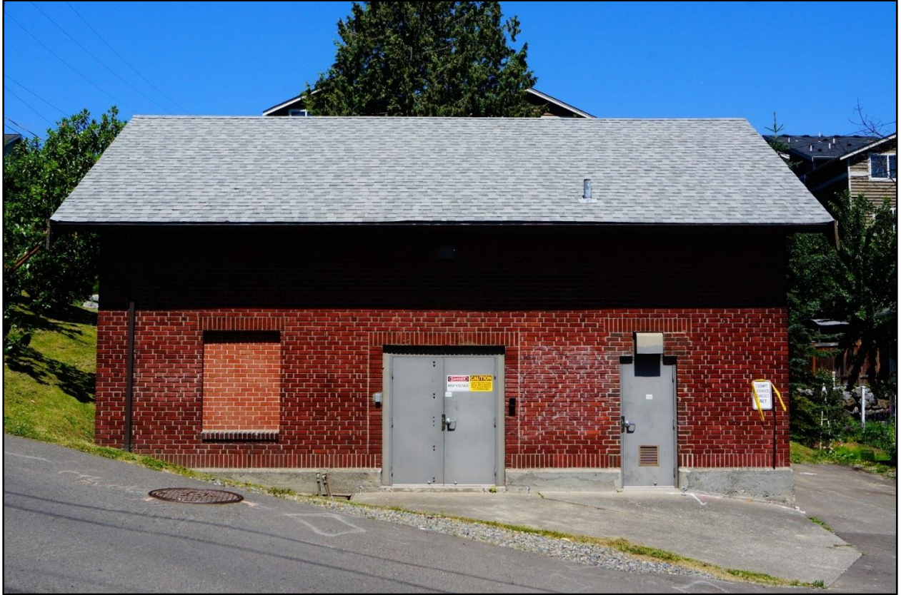
Photo 2. SW Spokane St. Pump Station, May 23, 2019, view north.
