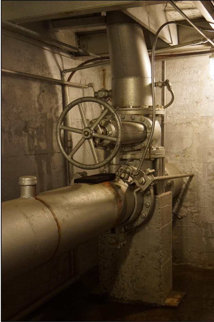
Photo 8. SW Spokane St. Pump Station, May 23, 2019, interior, basement floor, view southwest.
