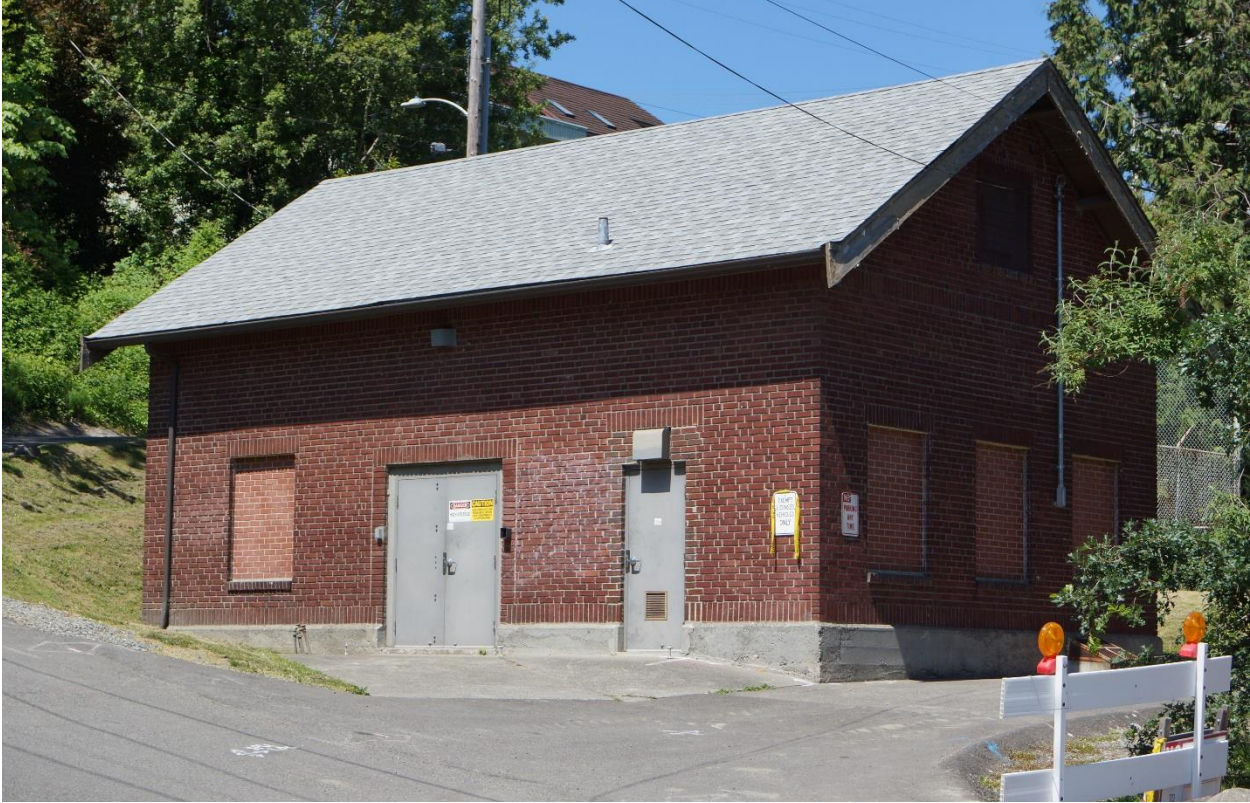
Photo 1. SW Spokane St. Pump Station site, May 23, 2019, view northwest.
