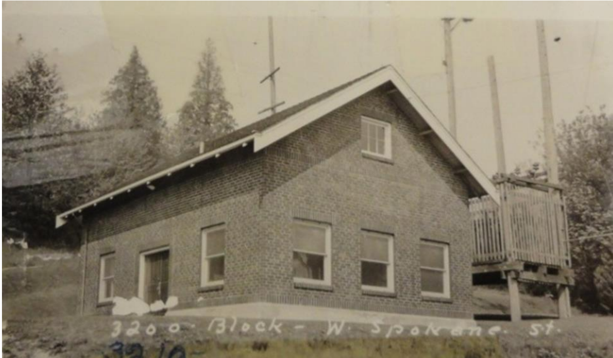
Figure 13. King County Assessor's photo of the SW Spokane St. Pump Station, view northwest (undated, ca 1936). On file at the Puget Sound Regional Branch of the Washington State Archives, Bellevue.
