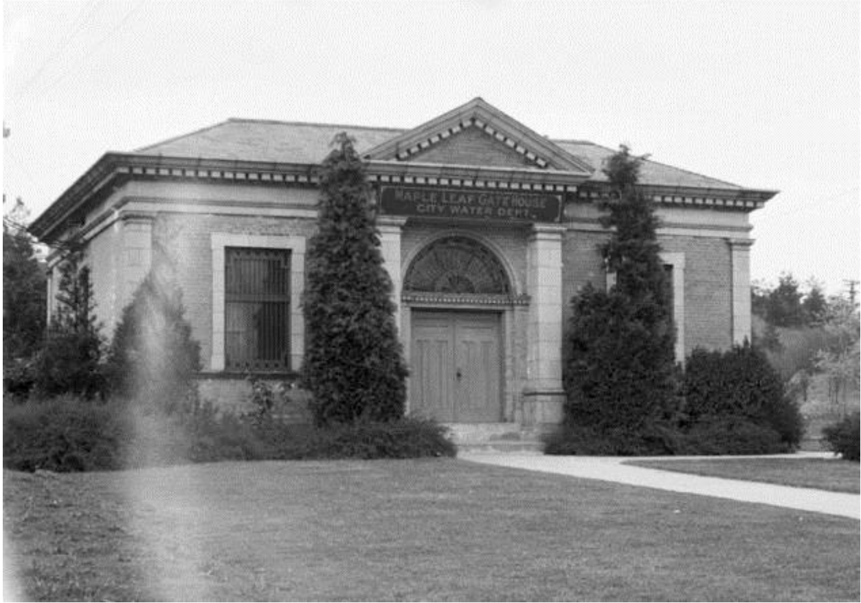
Figure 20. Examples of Seattle pump stations: Maple Leaf Pumping Station (photographed April 29, 1935). Photo on file with Seattle Municipal Archives, Seattle.
