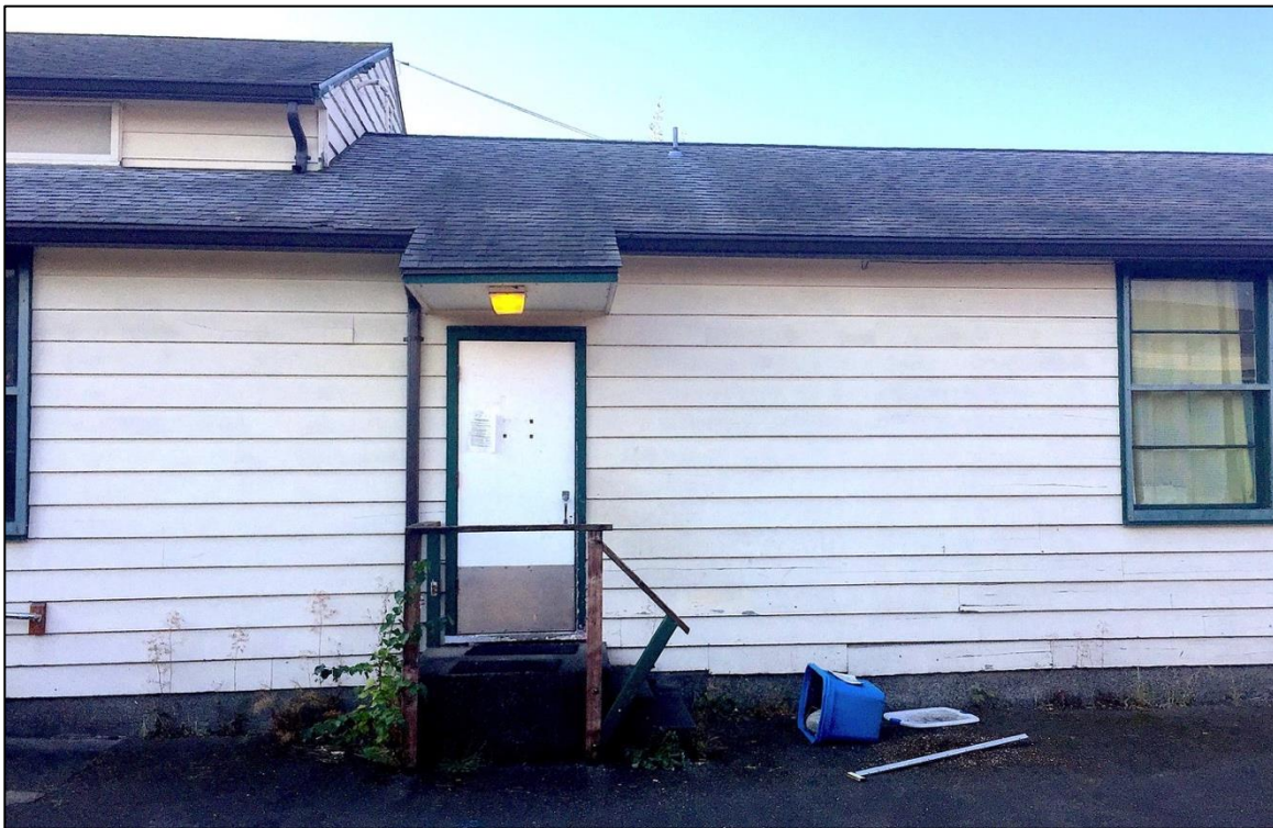
Figure 29. Western extent of the Central Section on the North side ends where the lower roof elevation to the right abuts the higher elevation on the left side of image. The lower roof elevation on the north extends west to the end of the Western Section. The door at finished floor level opens into the Western Section. To the door's right is a wooden, single-hung, four-sash window, which is contiguous to adjacent windows to the West (next figure 30).
