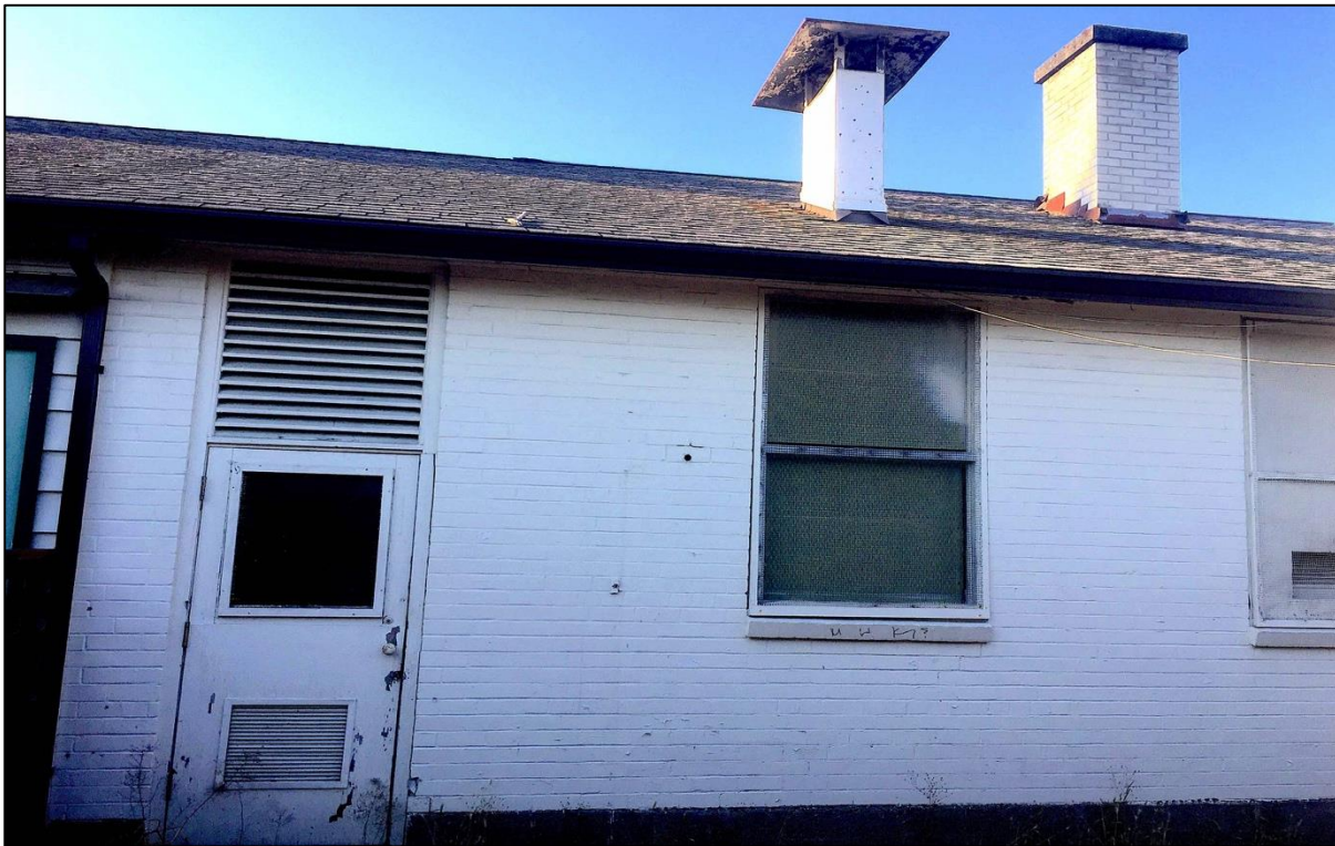
Figure 25. East Section, N side, overlaps Figure 24. Siding is brick masonry. Note white door at ground level with inset vent and window; ventilation extends from the door to the roof; two aluminum-screened, aluminum sash windows with brick window sills. Box vent, concrete-capped chimney visible on roof.
