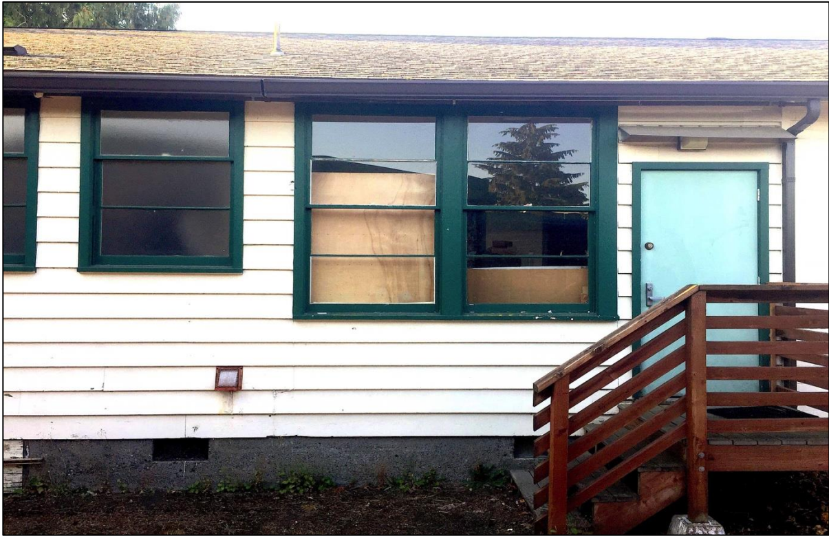
Figure 24. East Section, North side, overlaps Figure 23: L to R are two three-sash windows, two four-sash windows mullied together, a green door at finished floor level, wooden steps and deck to the green door.
