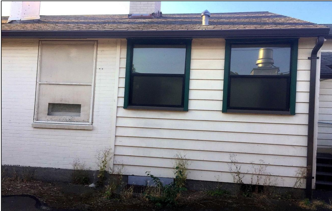
Figure 26. The Eastern Section, north side, west end, and just around the corner is the Central Section. The window in the brick part of the exterior wall (L) overlaps with Figure 25. Here, brick abuts a short section of cedar lap siding (R) which has two single-hung, two-sash vinyl windows with green wood trim.
