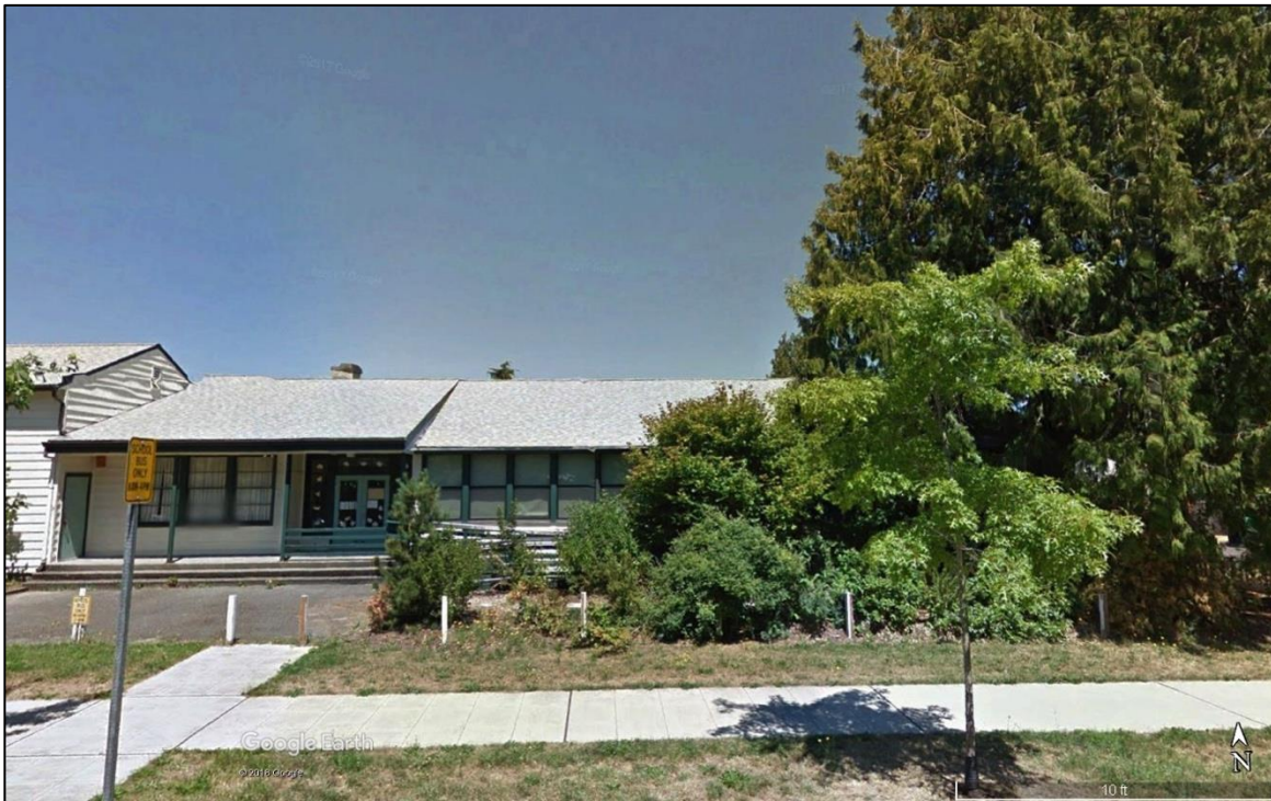
Figure 18. South street view of the original Shearwater Community Center. Three long concrete steps lead up to the porch and main entrance, under an extended roof supported by two green-painted wooden posts.
