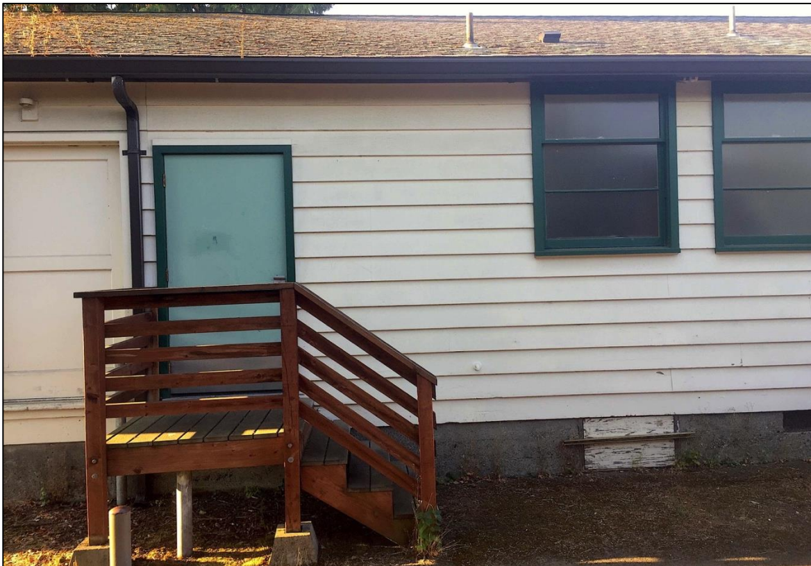
Figure 23. Eastern Section, north side, image overlaps with Figure 22, showing green door at finished floor level, wooden steps to it, two windows, secure boarded crawlspace opening in foundation, and a vent.
