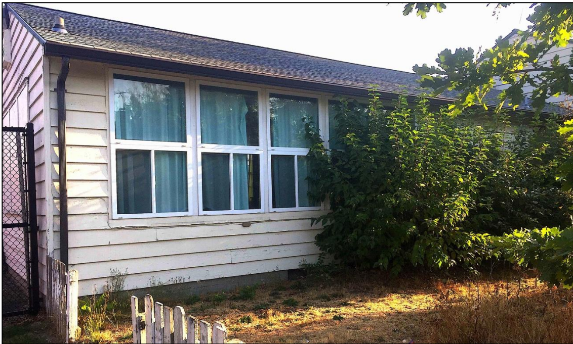
Figure 33. Southwest corner of the Western Section, showing new replacement vinyl windows. These are the only windows that do not have green-painted wooden frames.
