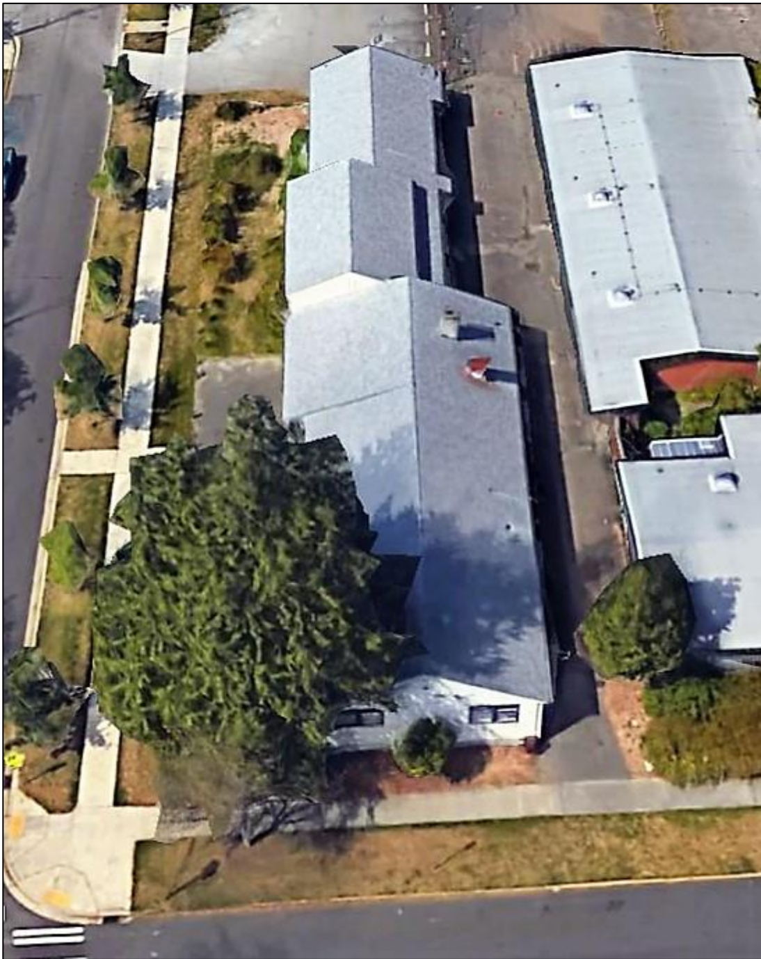
Figure 17. A tilted Google Maps image of Decatur Annex from the East (bottom) to the West (top). This perspective highlights the three sections of the building, provides a view of the roof and its different elevations and extensions, and the concrete-covered chimney, and vent box in the Eastern Section (original Shearwater Community Center). The lighter-colored roofing material on Decatur Annex today replaced the original asphalt roofing in 2009. On the North side of Decatur, there are short roof extensions to provide small porches for two door accesses into the Central and Western Sections, plus an extension over the offset to the north on the Western Section's northern exposure. On the South side of Decatur, there is a slightly shallower slope to the roof that covers the main entrance and porch area of the original Shearwater Community Center.
