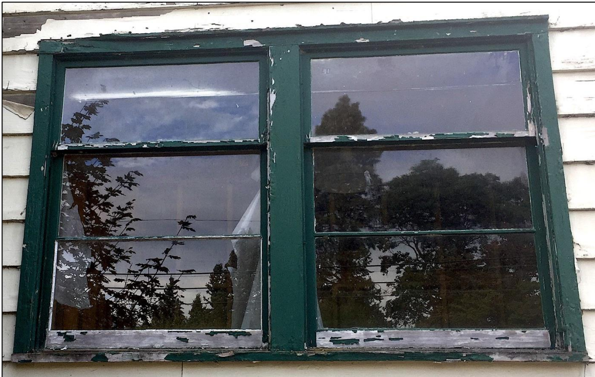
Figure 21 . Close up of the northeast pair of windows on the East side of Decatur in Figure 20. The windows have not been replaced by vinyl or aluminum, it is not clear whether these windows date from 1945 or were replacement wood windows in 1961 (see Appendix 1).
