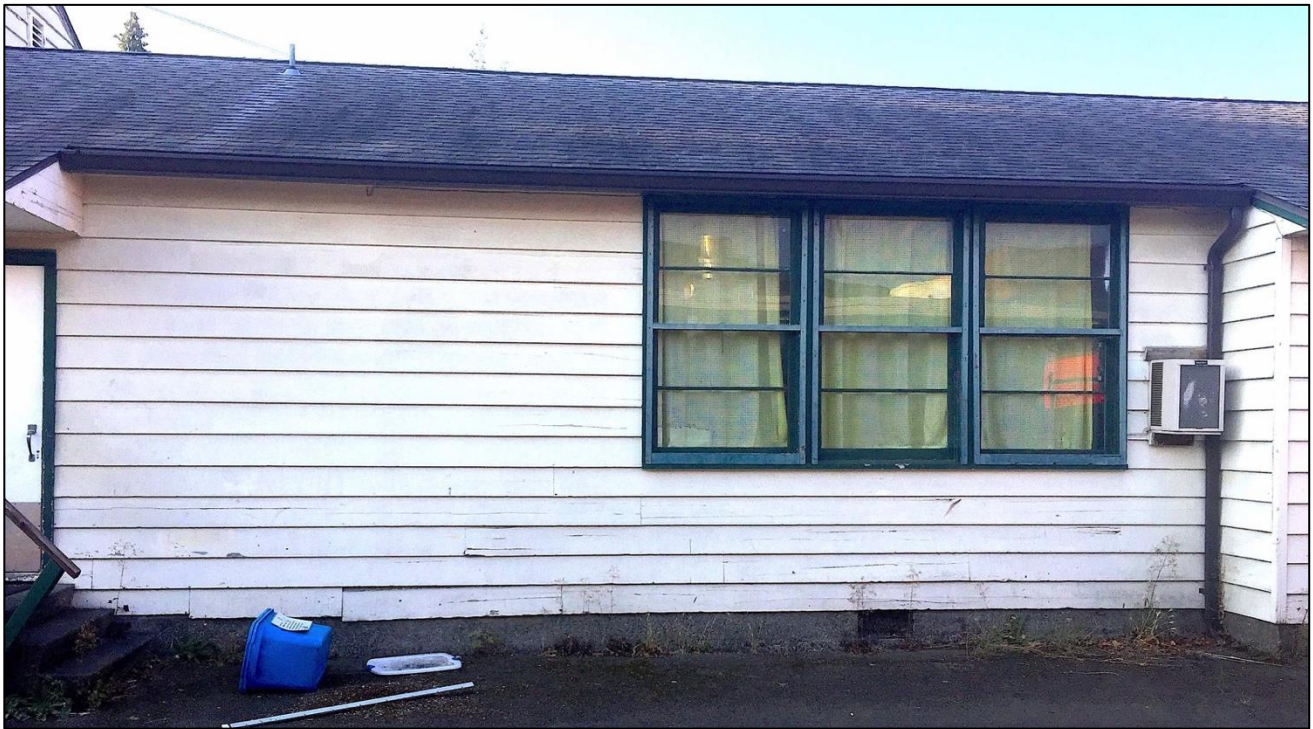
Figure 30. Central Section, Northern Exposure, West Side, showing the three wooden windows mullied together. At the right in the image is the only eastern exposure of the Western Section, which extends about a foot further north than the Central Section. Note the concrete foundation is shorter at this end.
