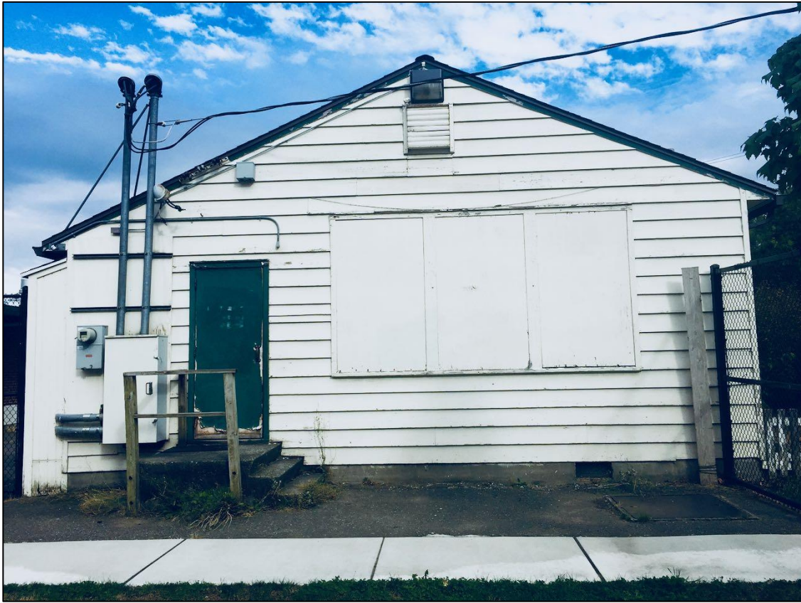
Figure 32. Western Section, West Side. Asymmetrical roof, unlike the symmetrical East Side. Left side door is at the finished floor level, reached by wooden steps and deck. To the right of the door are three boarded windows, and to left of the door is what appears to be an enclosed area used for electrical utilities.
