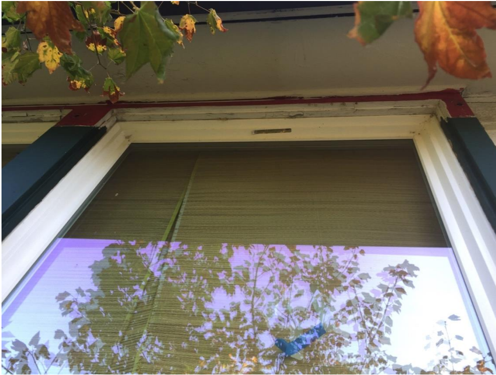
Figure 34. Central Section, close up of a replaced vinyl window on the east side of the Southern Façade of the Central Section. It shows red trim on the outside, which may or may not be significant historically.
