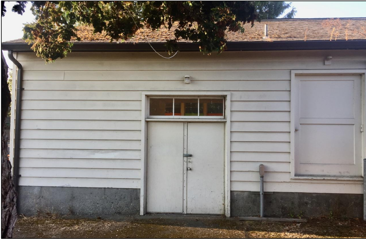
Figure 22. Eastern Section, north side, east end, door (L) at ground level; door (R) at finished floor level.
