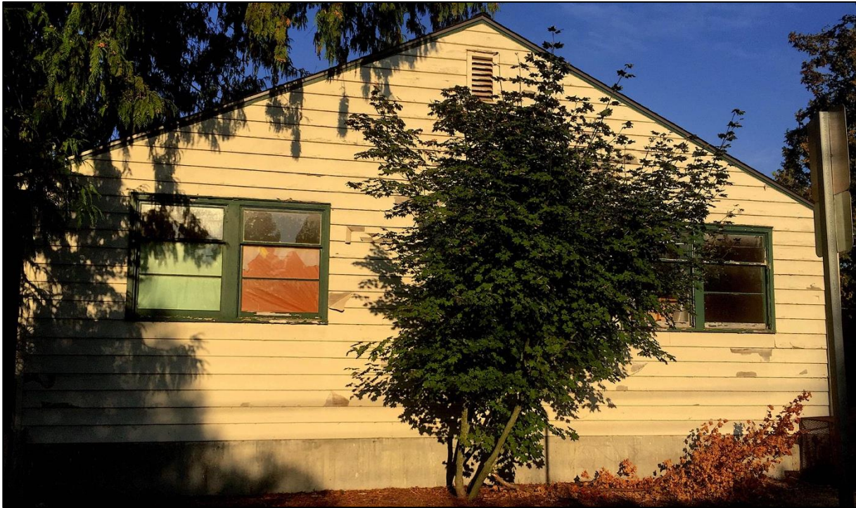
Figure 20 . East side of Decatur Annex, East Section. Note peeling paint, including around the windows, and the concrete foundation at the base of the wooden frame structure.
