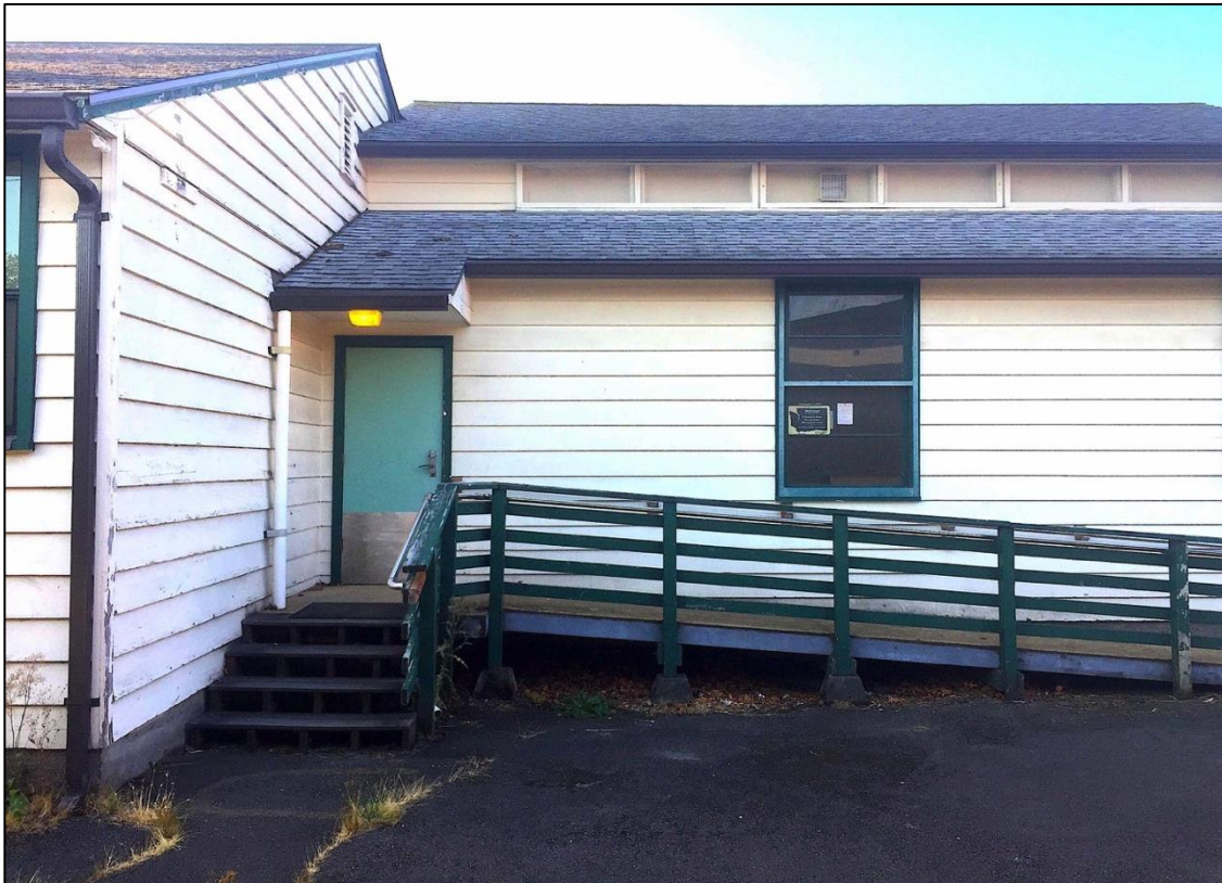
Figure 27. The wall on the left side of this image is the extent of the Eastern Section's West side. The Central Section is offset to the south about three feet, with a lower roof that has two elevations.
