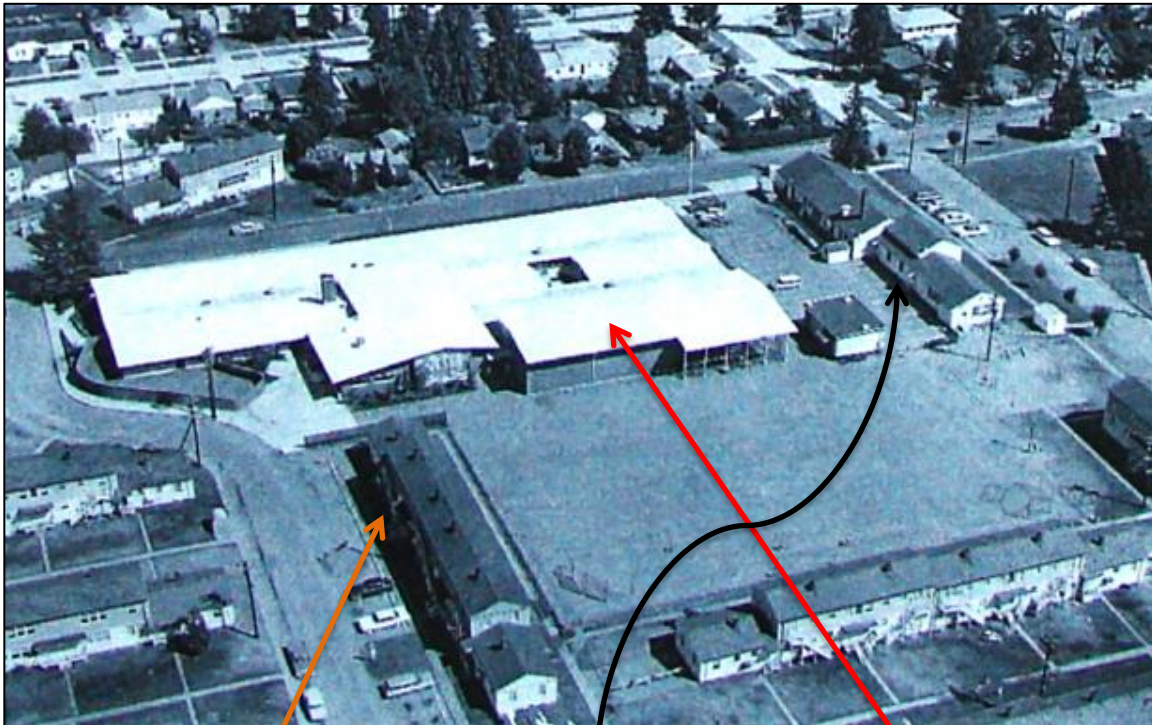
Figure 5. Aerial view showing that years after Decatur Elementary School had been built in 1961, Shearwater housing and Community Center remained in use. City of Seattle Archives, 1965.
