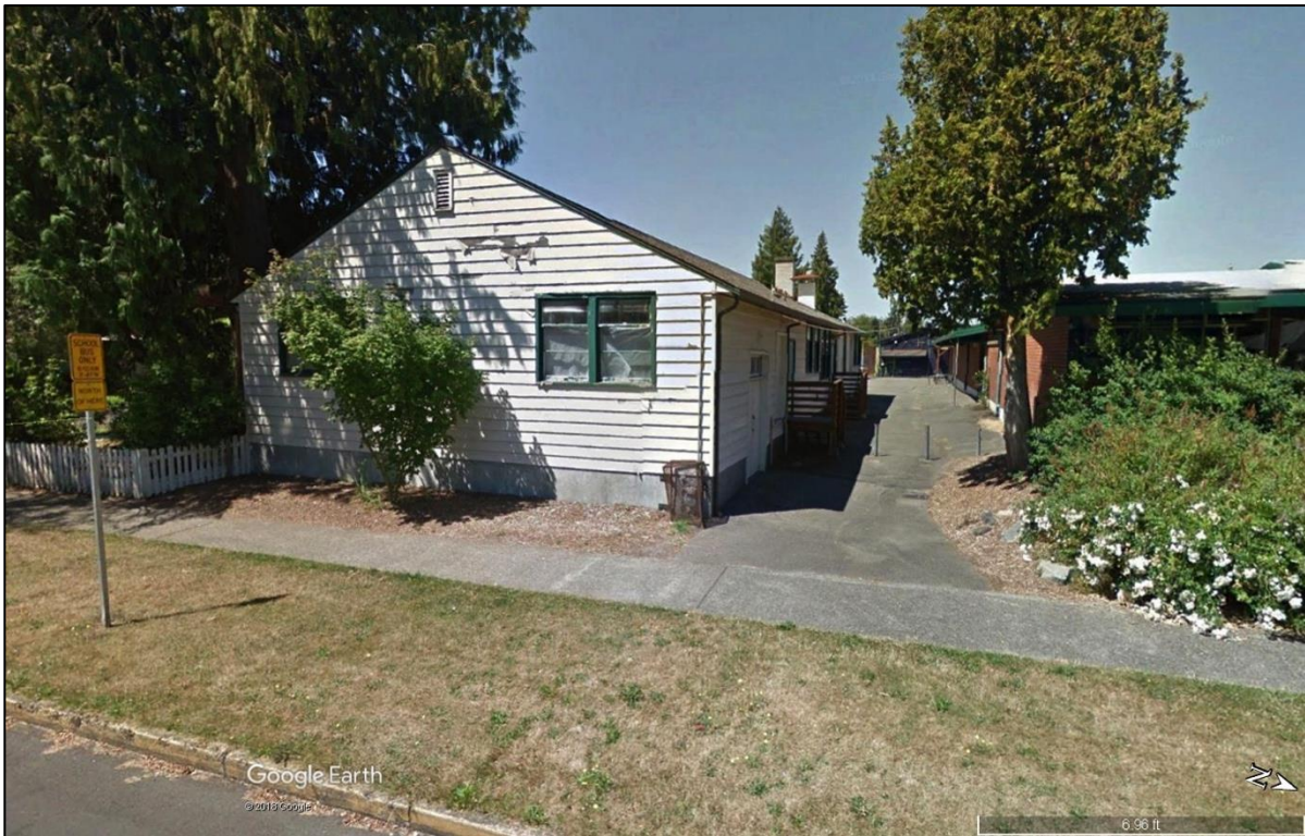
Figure 16. Google Maps image of the north side of Decatur Annex from the East, looking West from 43 rd Ave NE, along the open space between the Decatur Annex and Decatur Elementary School to the North (right side of image).
