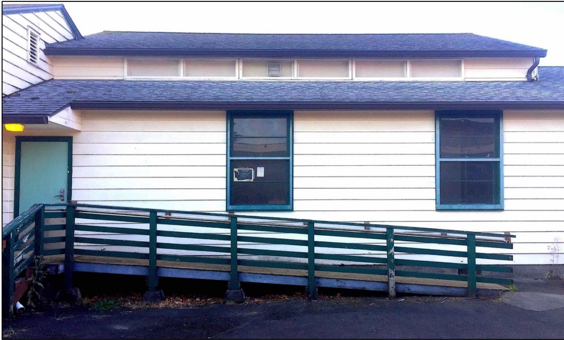
Figure 28. Central Section, North side, showing higher and lower roof elevations. There is row of short wide windows above the lower roof, and two single-hung, wooden two-sash windows, green trim below it.
