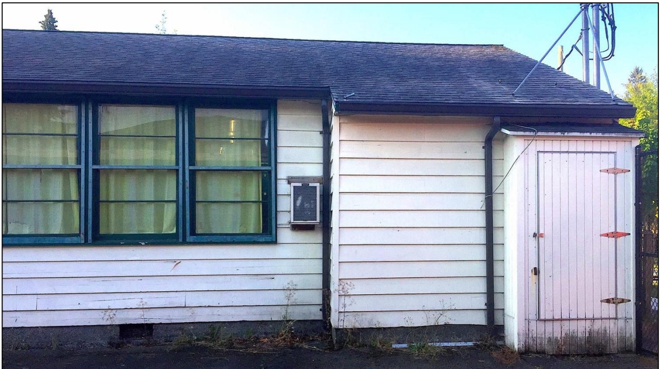
Figure 31. Western Section, North side, West end. The main structural feature is the short extension of the end of the Western Section's northern wall and roof towards the North by about a foot. The box on the wall to the right of the windows is an air conditioner. The tall wooden unit on the right houses the electrical utility panel.
