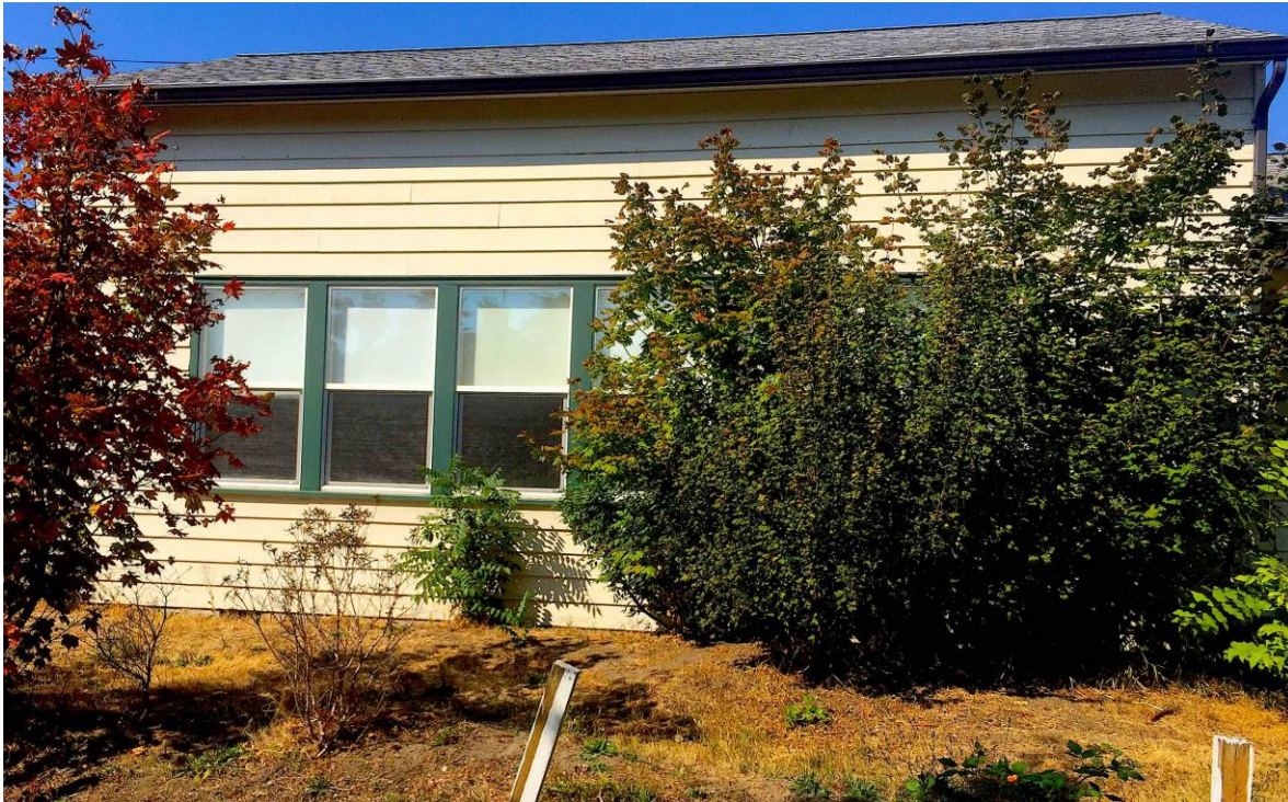
Figure 35. Central Section, south side. There are seven contiguous windows on this side (four behind shrubbery). The original windows have been replaced with double hung two-sash vinyl windows, framed and mulled together with green-painted wood.
