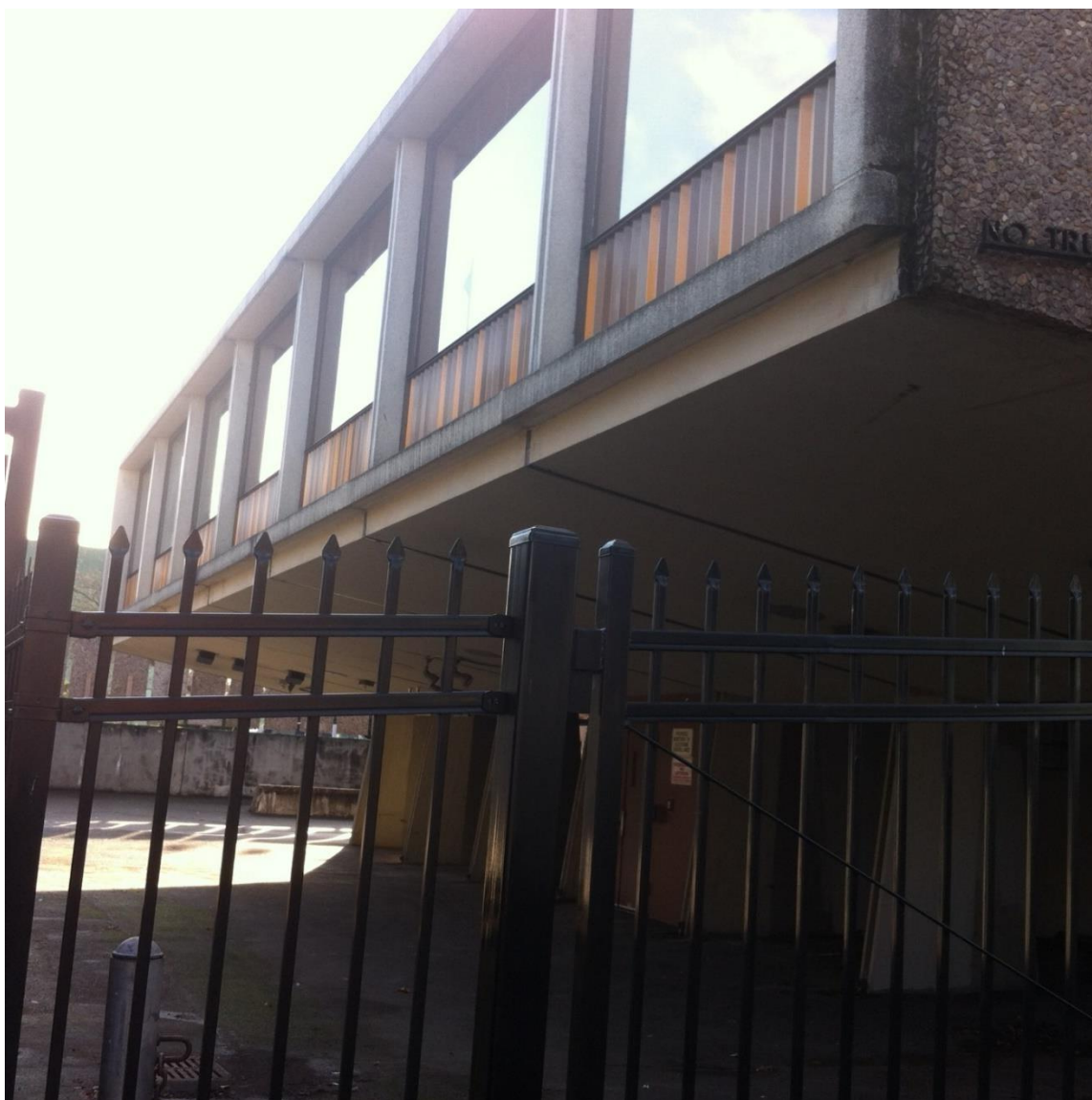
Figure 7: East elevation and parking spaces between pilotis. Looking southwest. Photo Date: January 6, 2016.
