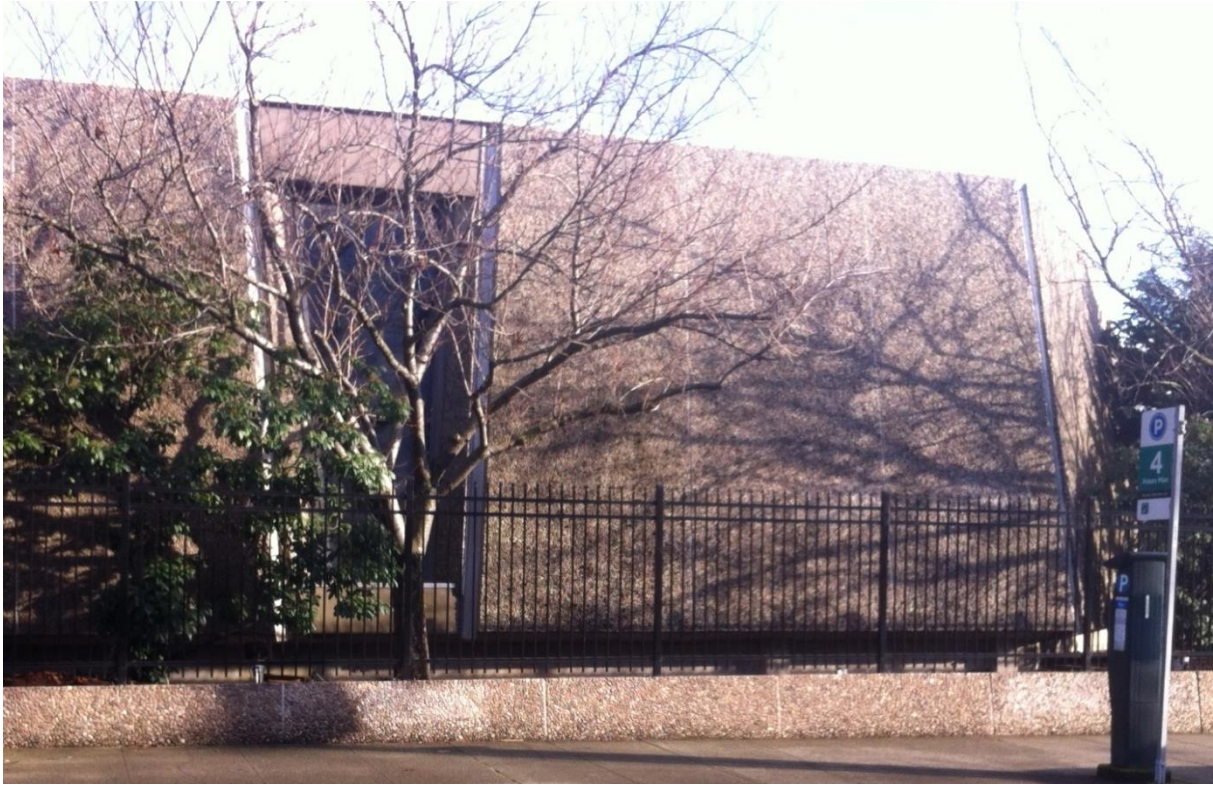
Figure 11: Western elevation looking east. Window and all panels showing added in 1985. Photo Date: January 6, 2016.
