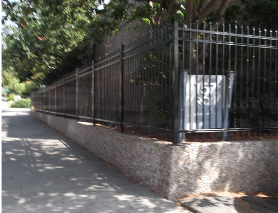
Figure 21: Aluminum fence addition ca. 2008. Looking north on Warren Street. Photo Date: 2015.
