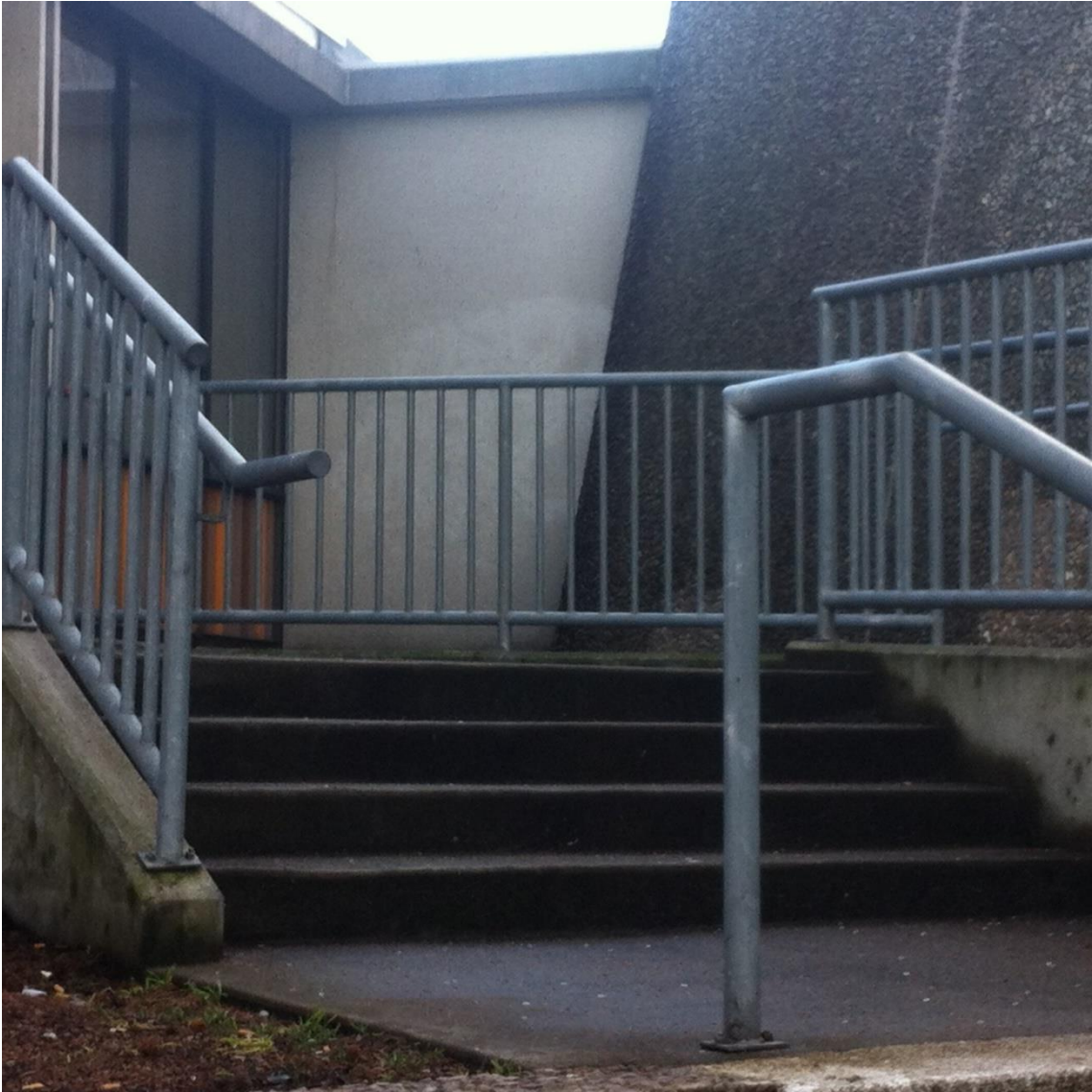
Figure 6: North elevation looking south where two wings connect. Photo Date: January 6, 2016.
