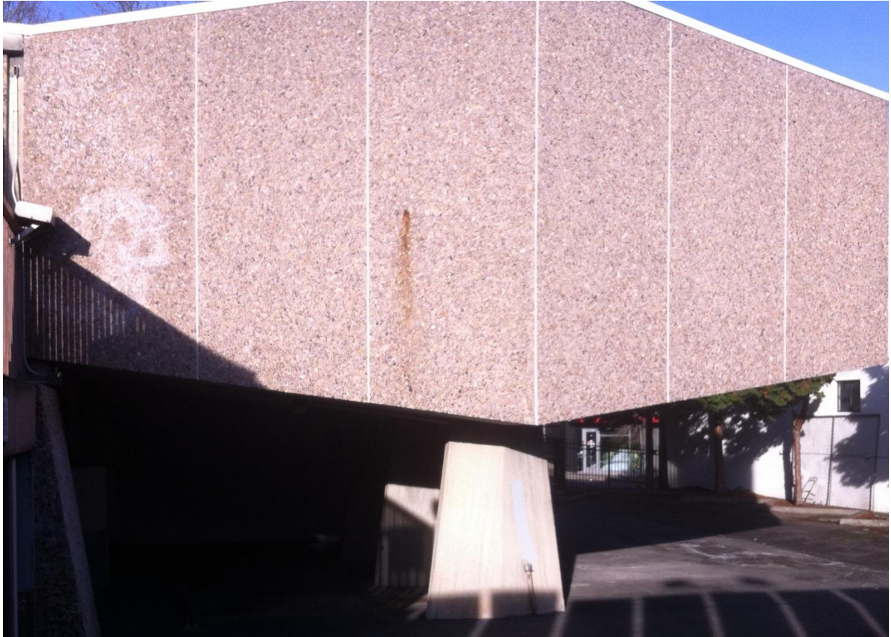
Figure 14: Southern elevation of hexagonal office wing looking north. Photo Date: January 6, 2016.
