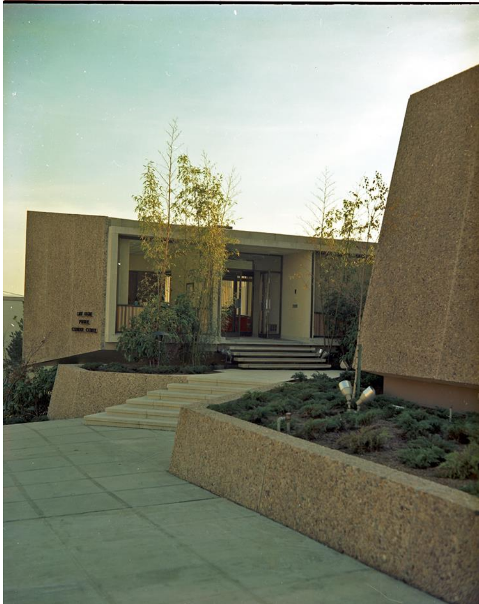
Figure 26: Power Control Center. Looking southeast towards the hexagonal eastern wing and building entrance. Photo Date: 1968.
