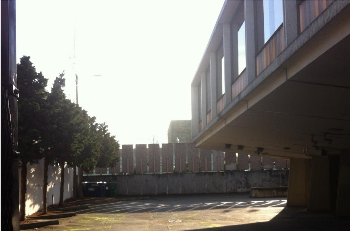
Figure 9: Parking lot and fence panels. Looking south. Photo Date: January 6, 2016.
