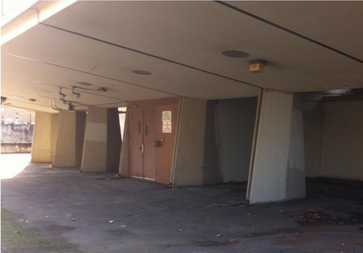
Figure 8: Parking spaces under east wing and basement entrance; looking southwest. Photo Date: January 6, 2016.
