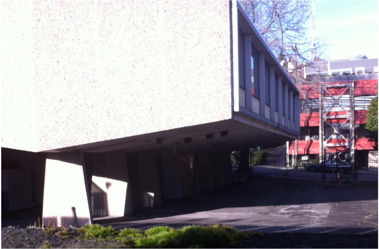
Figure 15: Southern and eastern façades and parking area looking north. Photo Date: January 6, 2016.
