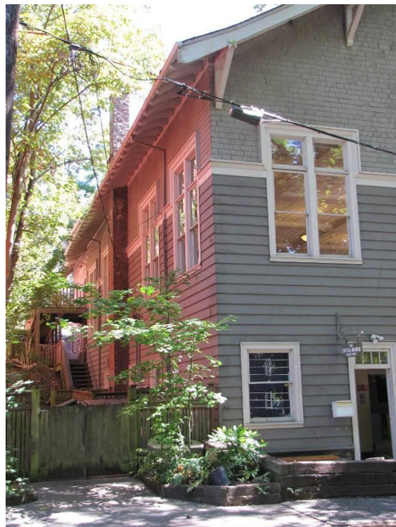
Figure 25. Southwest corner. Image courtesy of DAHP, 8/16/2016.
