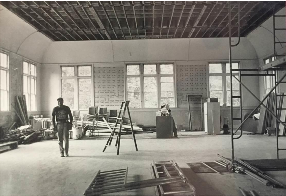
Figure 18. Ca. 1992 images of repairs to damage caused by an arson fire.
