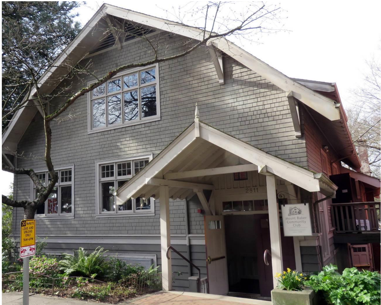
Figure 23. Front east facade.
