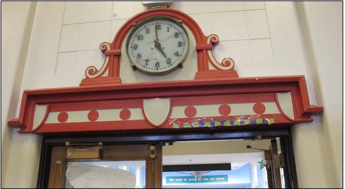
Figure 45 • Clock at entry to former auditorium existing library/resource room, 1914 Addition (Edgar Blair)
