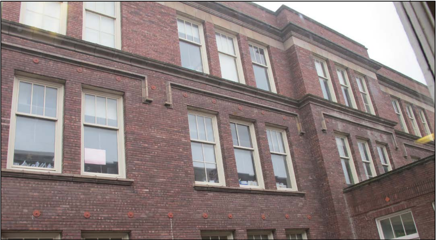
Figure 24 • Lincoln High School, 1907 Central Block (James Stephen), northern façade
