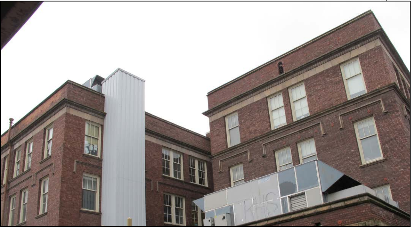
Figure 25 • Lincoln High School, 1907 Central Block (James Stephen), eastern façade northern wing, northern and eastern façade central wing
