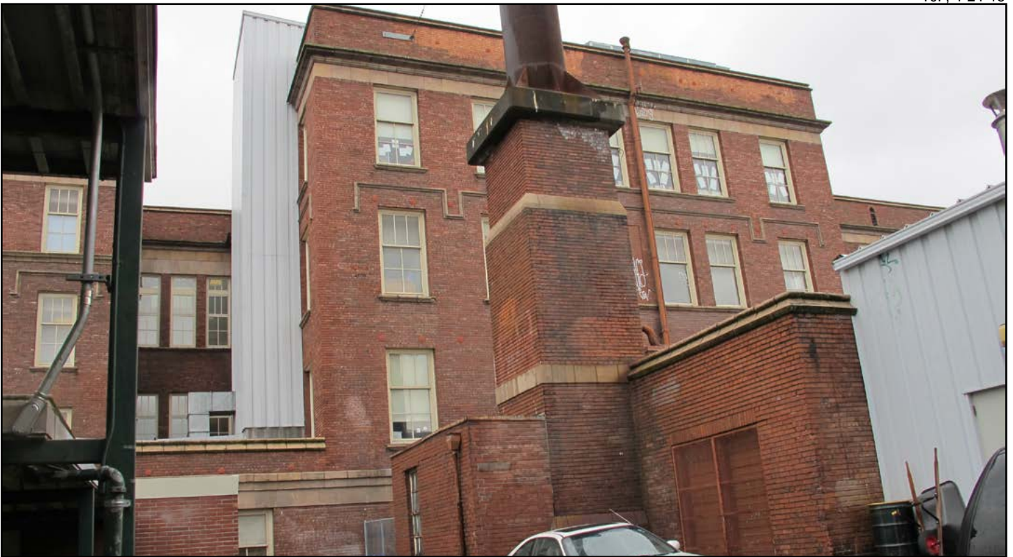
Figure 26 • Lincoln High School, 1907 Central Block (James Stephen), central wing, 1913 Blair boiler addition
