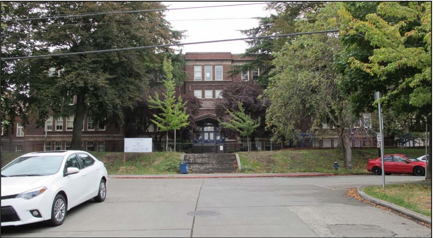
Figure 21 • Lincoln High School, 1907 Central Block (James Stephen), western façade
