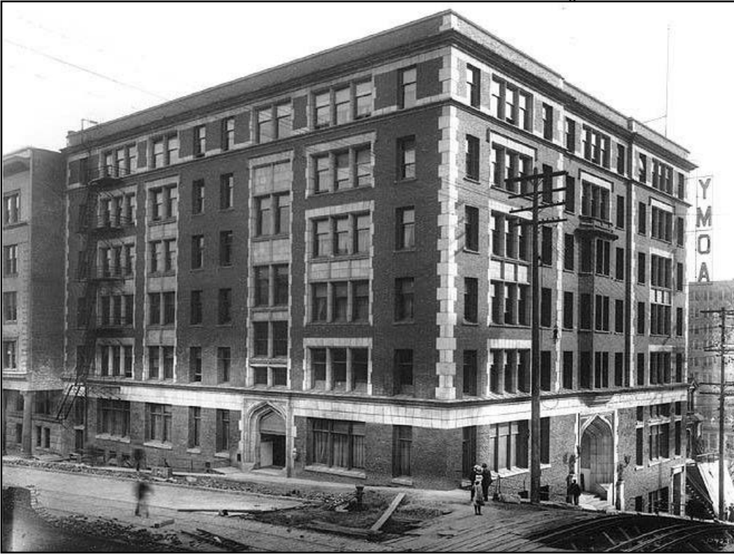
Figure 133 • Seattle YMCA, at Madison Street and Fourth Avenue (1909, Pearson Construction Co., contractor, demolished)
