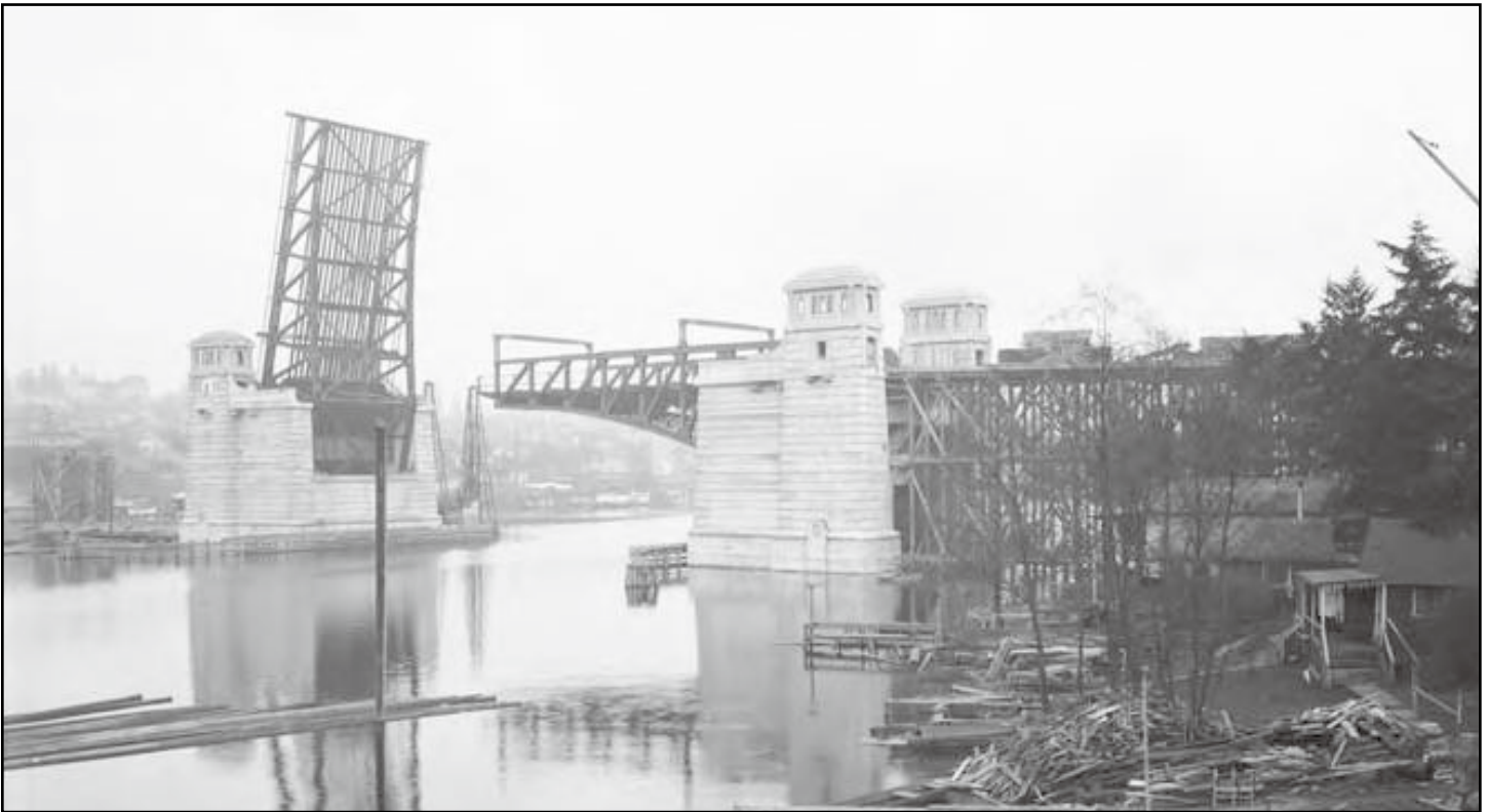
Figure 87 • University Bridge under construction, ca. 1919
