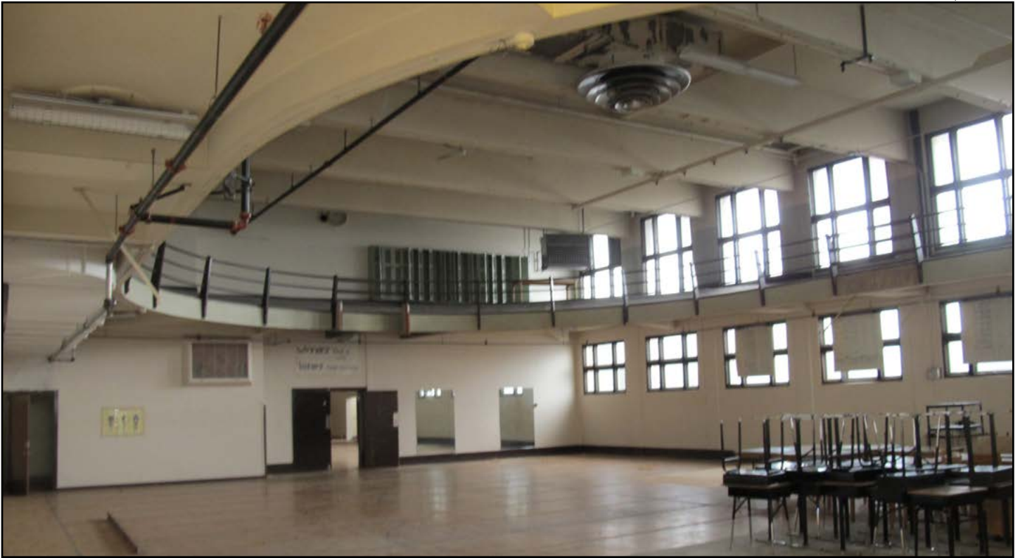
Figure 49 • Eastern “Boys” Gymnasium, 1914 Addition (Edgar Blair)
