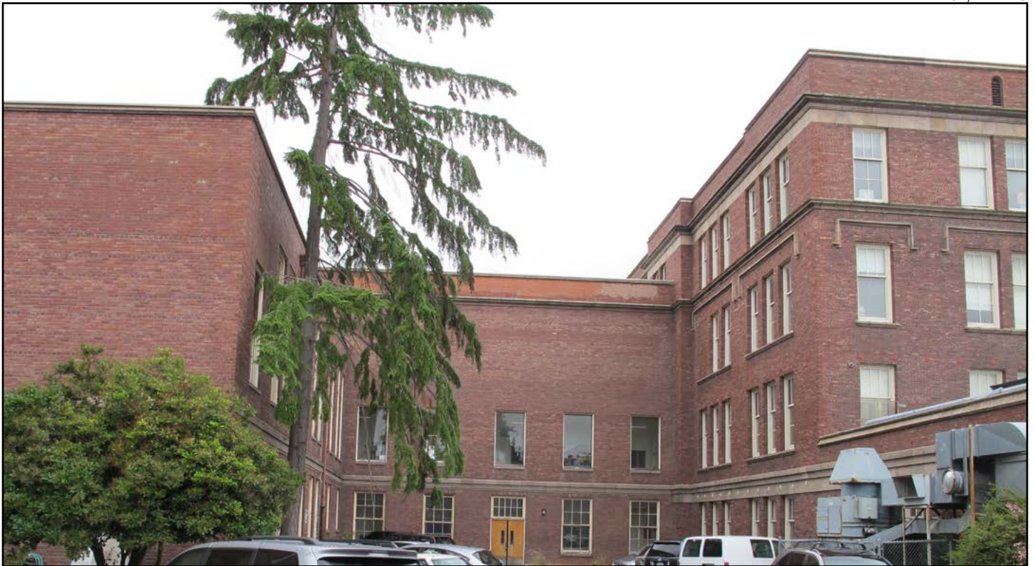
Figure 28 • Lincoln High School, 1907 Central Block (James Stephen), southern façade and 1930 Naramore southern addition
