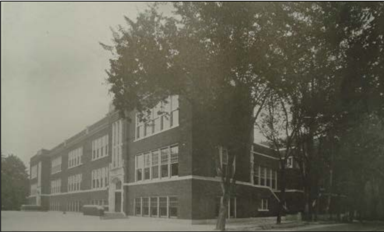
Figure 130 • Couch Elementary School, Portland, Oregon (1914-1915, Floyd Naramore)
