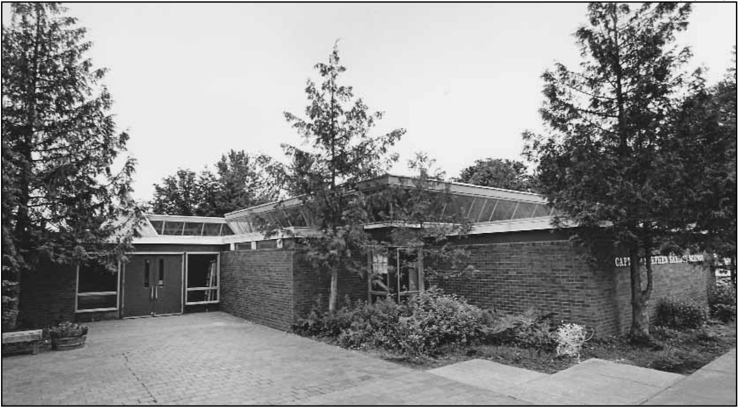
Figure 129 • Captain Steven E. Sanislo School (1970, Sullam, Smith & Associates, altered)
