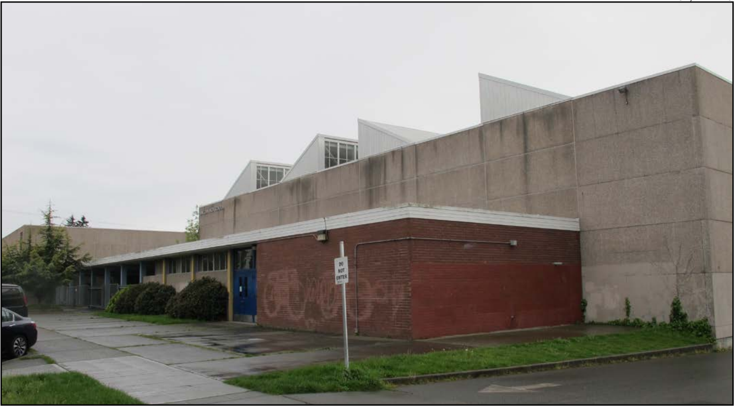
Figure 63 • Eastern façade of gymnasium viewing south, 1958 buildings (NBBJ)
