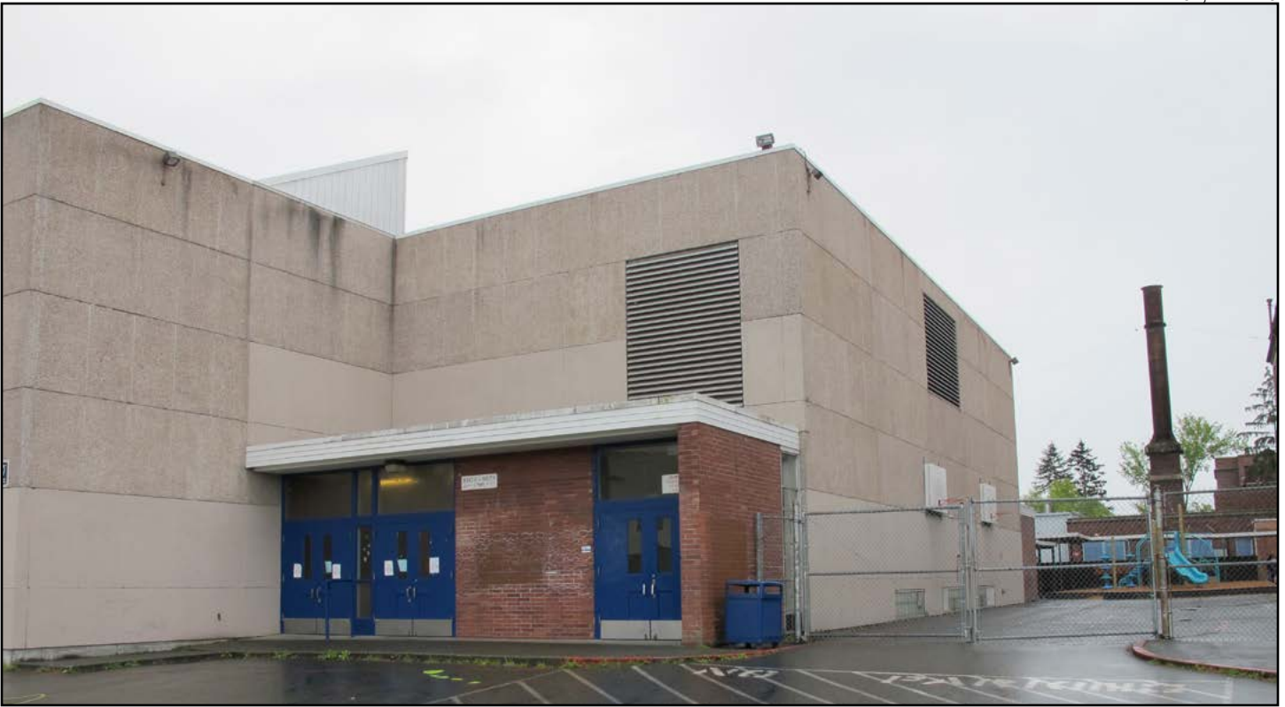
Figure 65 • Western façade viewing south, 1958 buildings (NBBJ)
