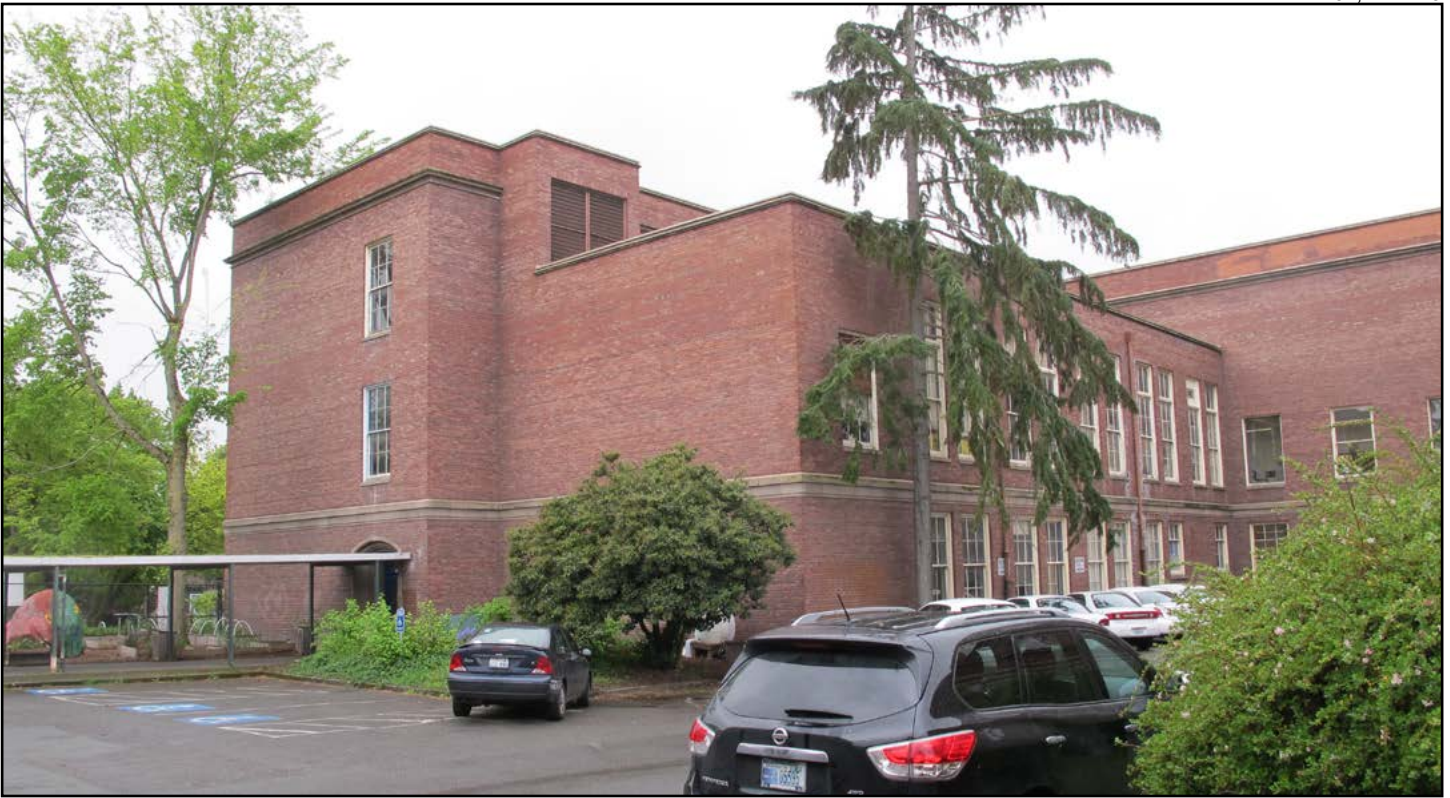
Figure 55 • Eastern and northern façades, 1930 Addition (Floyd Naramore)
