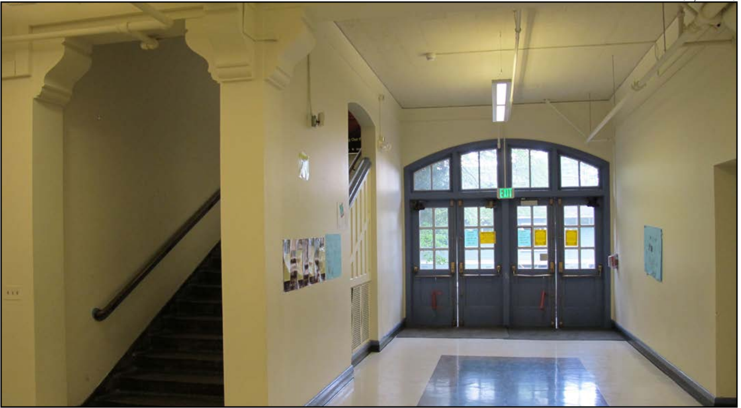
Figure 57 • Southern entry, 1930 Addition (Floyd Naramore)
