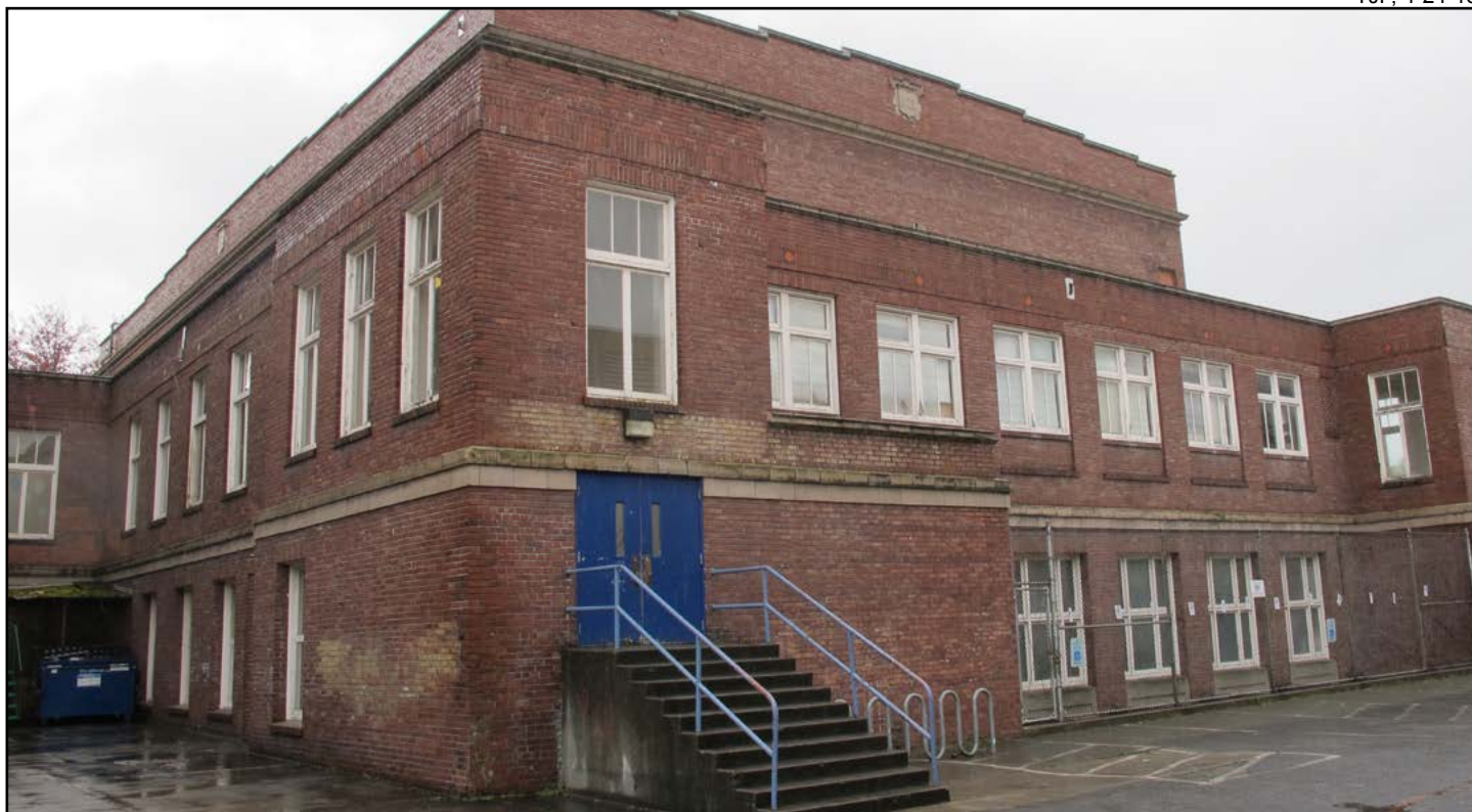
Figure 42 • Lincoln High School, 1914 Addition (Edgar Blair), western and southern façades
