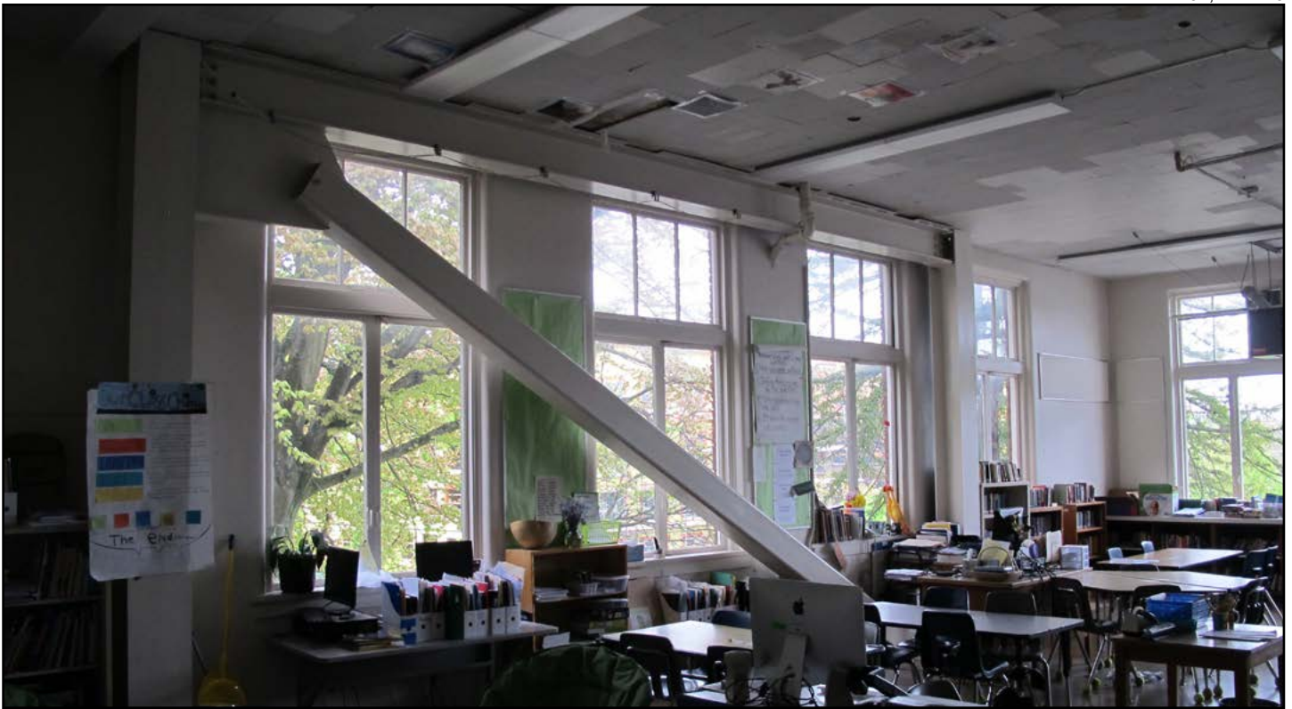
Figure 47 • Classroom with seismic retrofit steel at western end 1914 Addition (Edgar Blair)
