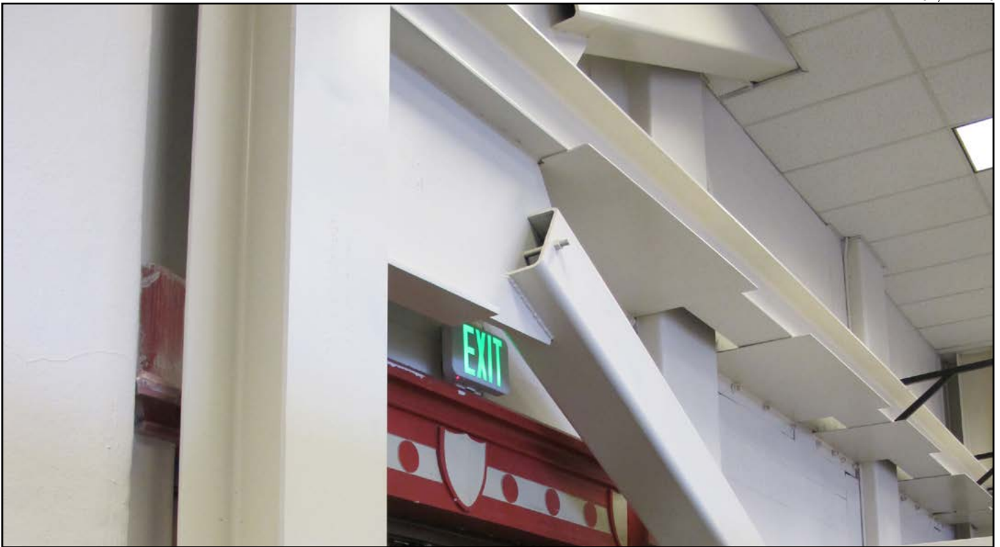
Figure 46 • Seismic retrofit steel at existing library/resource room, 1914 Addition (Edgar Blair)
