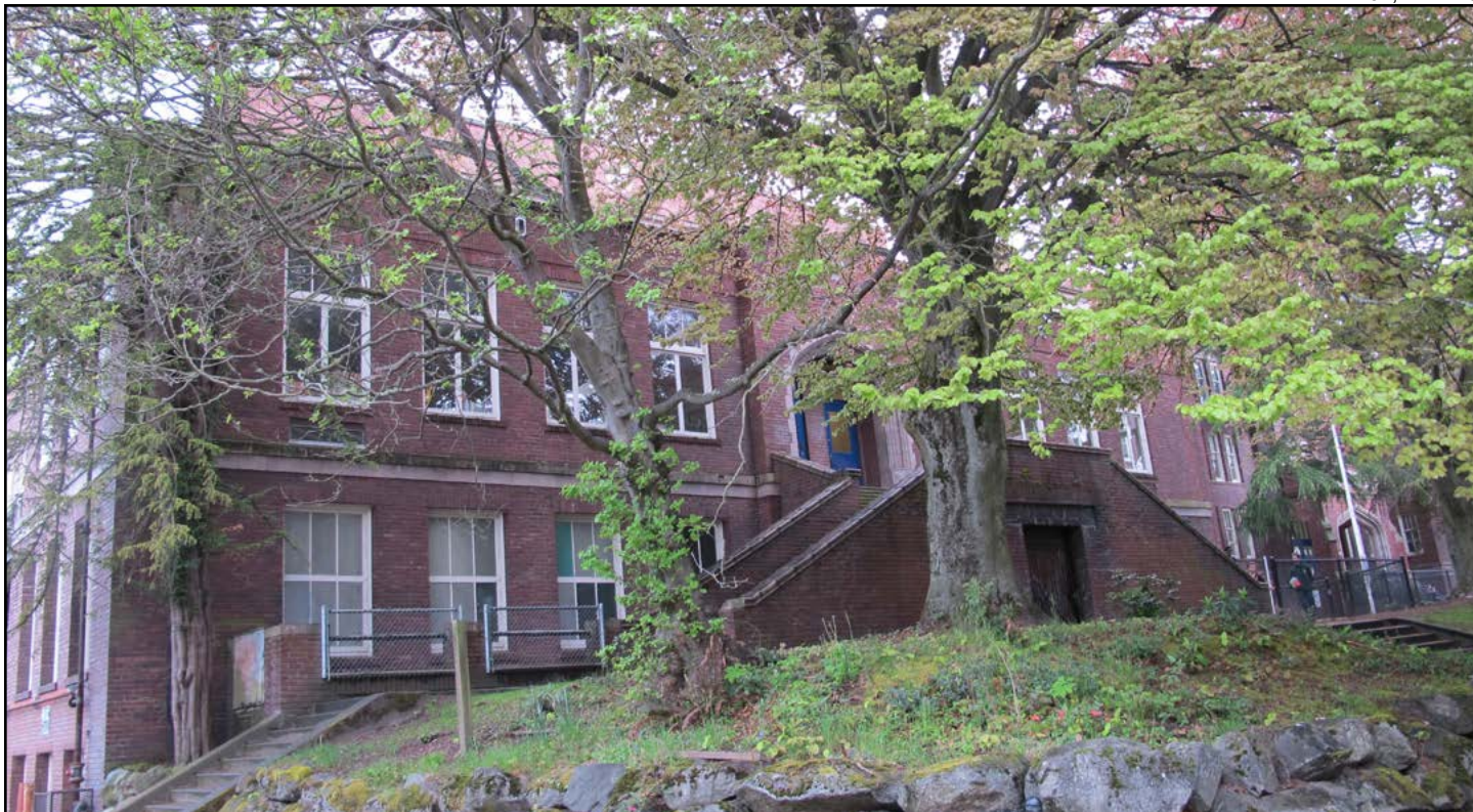
Figure 39 • Lincoln High School, 1914 Addition (Edgar Blair), western façade
