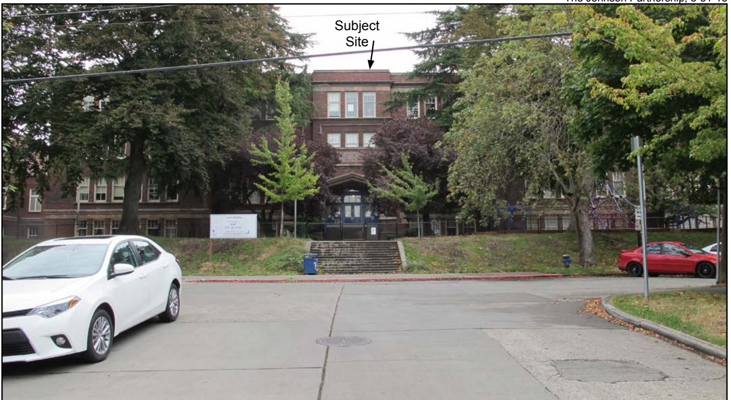
Figure 5 • View B - Viewing east from N 44th Street
