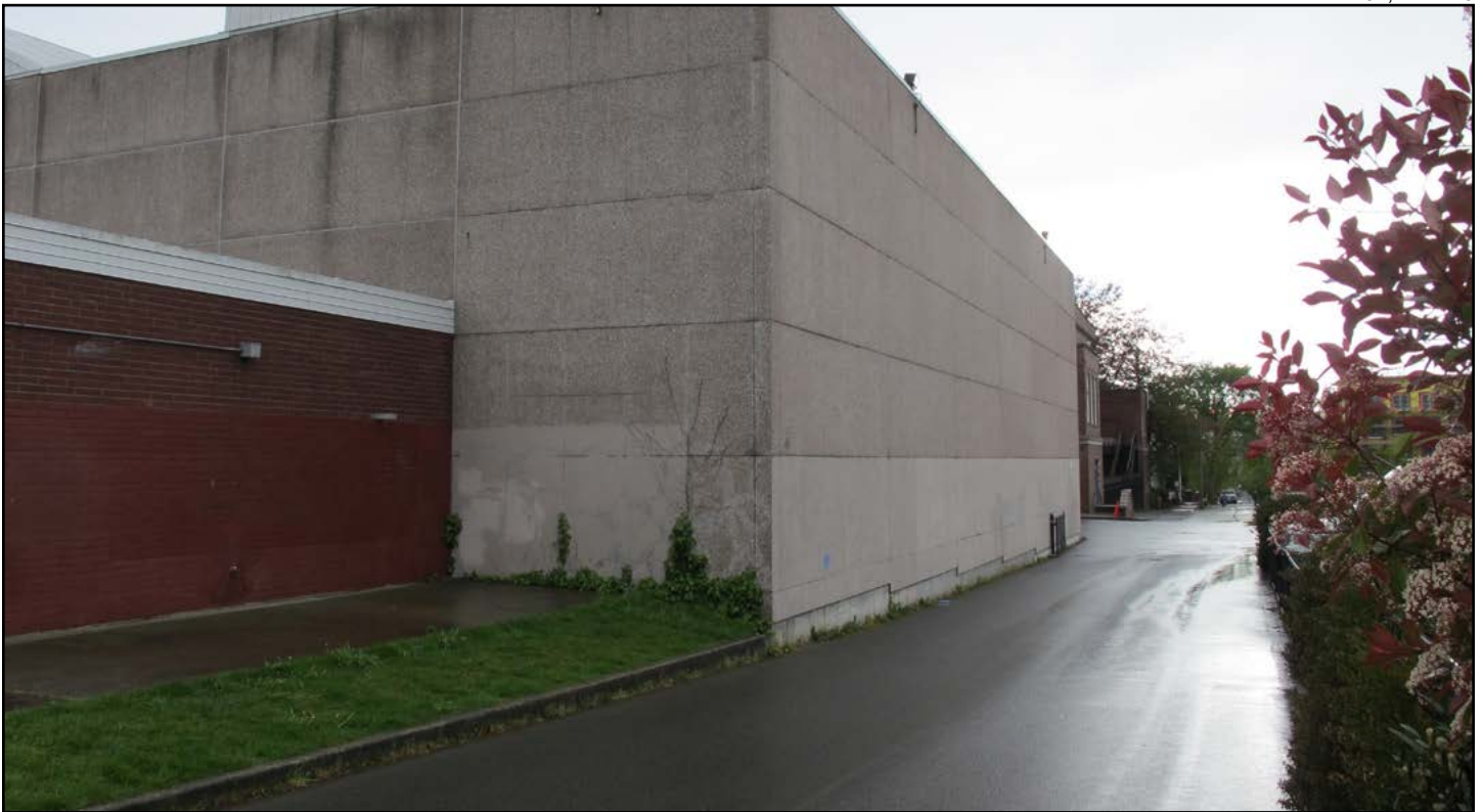
Figure 64 • Northern façade viewing west, 1958 buildings (NBBJ)
