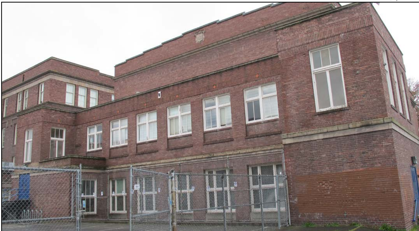
Figure 41 • Lincoln High School, 1914 Addition (Edgar Blair), western façade
