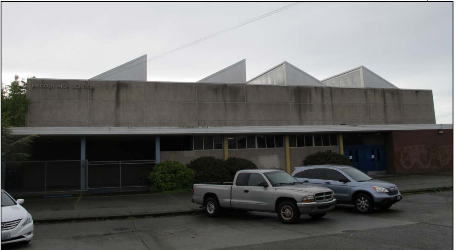
Figure 62 • Eastern façade of gymnasium, 1958 buildings (NBBJ)
