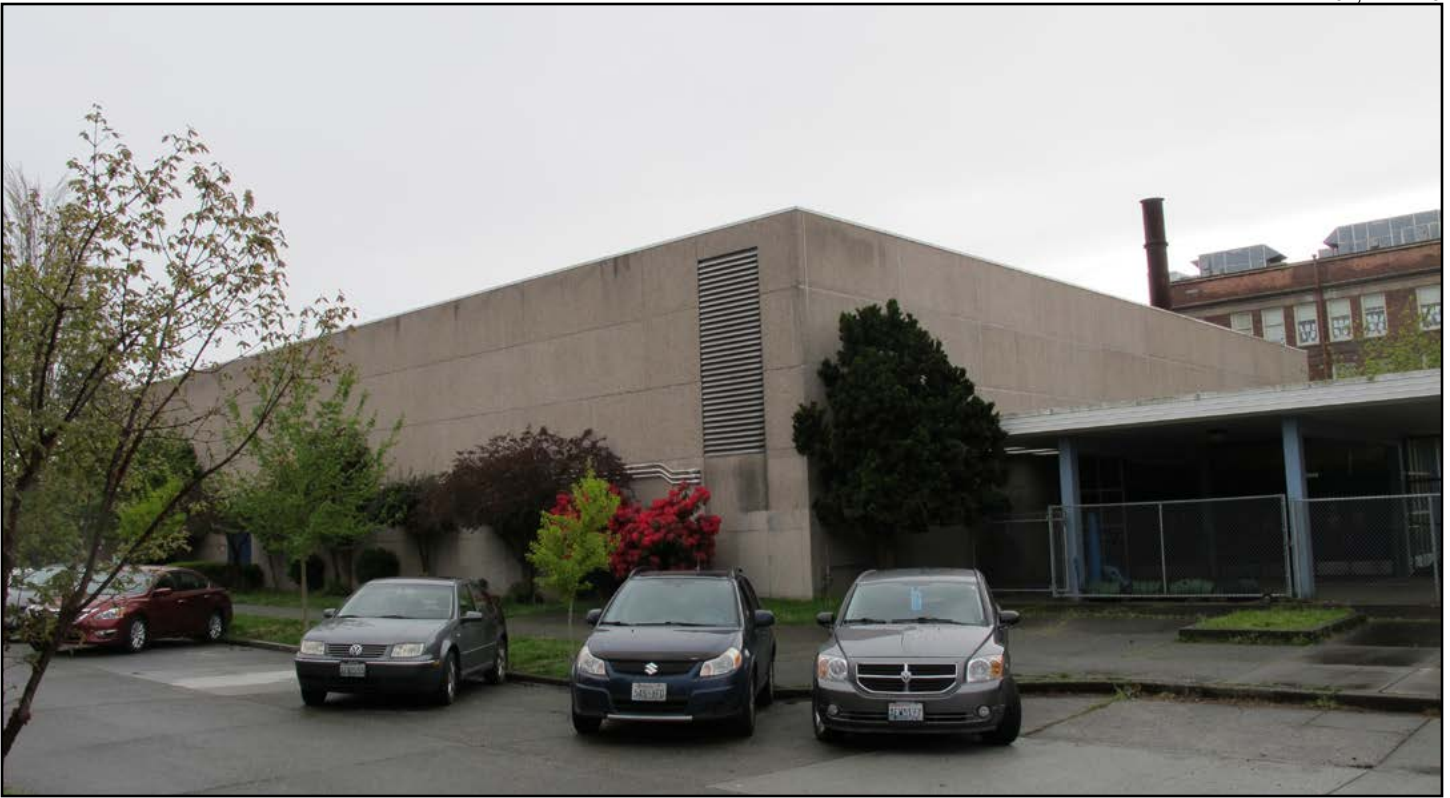
Figure 73 • Eastern façade auditorium, 1958 buildings (NBBJ)
