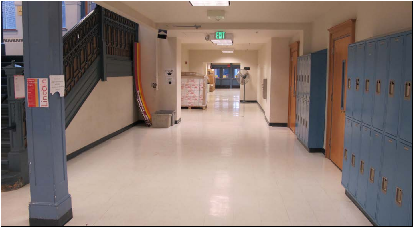
Figure 37 • Lincoln High School, 1907 Central Block (James Stephen), basement hall viewing east
