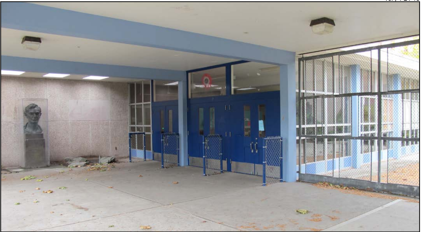
Figure 72 • Northern entry to auditorium, 1958 buildings (NBBJ)
