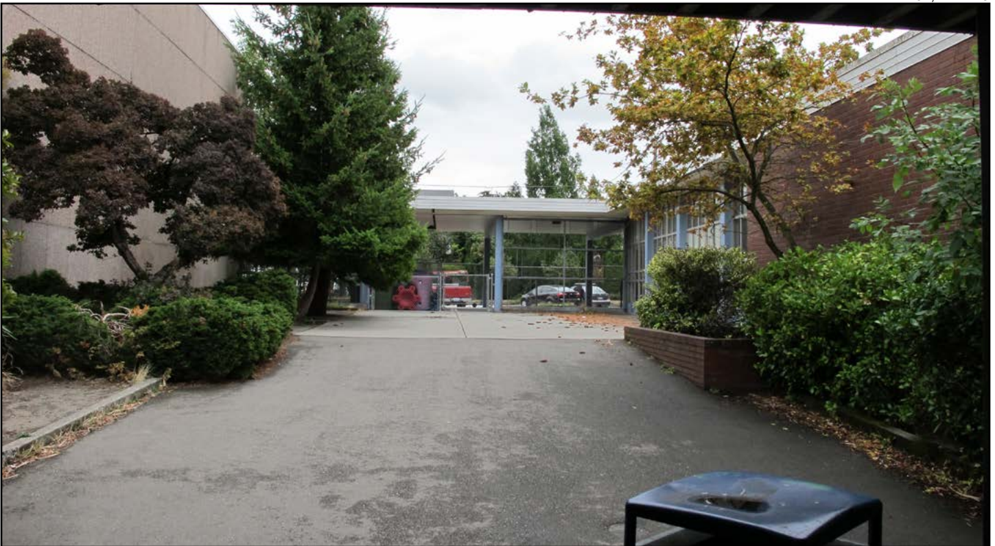
Figure 66 • Southern façade of gymnasium, northern façade auditorium, and connecting breezeway, 1958 buildings (NBBJ)
