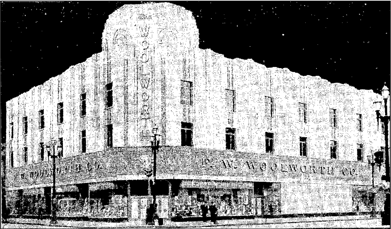
Figure 134 • Woolworth Building at Third Avenue and Pike Street (now the Ross building, 1940, J.B. Warrack, contractor)
