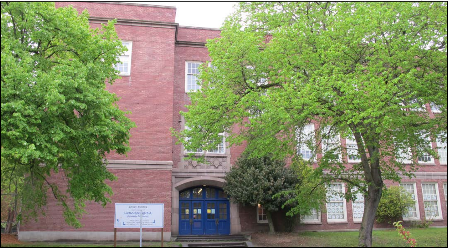
Figure 51 • Southern façade, 1930 Addition (Floyd Naramore)
