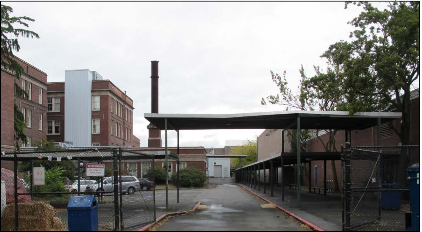
Figure 77 • Western façade auditorium complex, viewing north, 1958 buildings (NBBJ), with 1914 boiler room in the distance (Edgar Blair)
