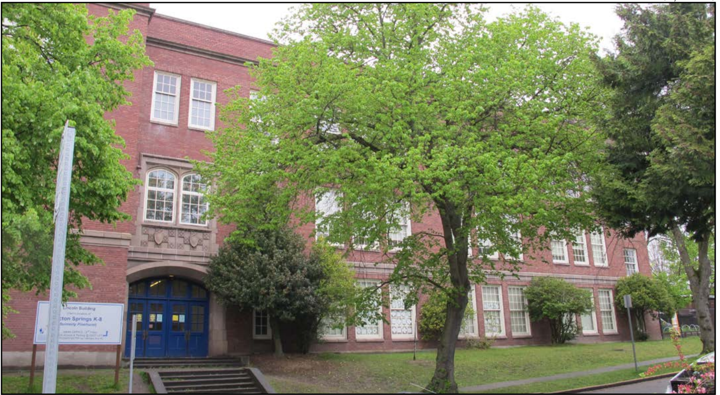
Figure 52 • Southern façade, 1930 Addition (Floyd Naramore)
